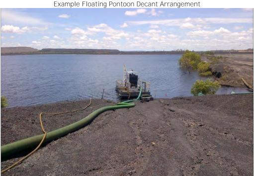
Plate 4 Example Floating Pontoon Decant Arrangement
