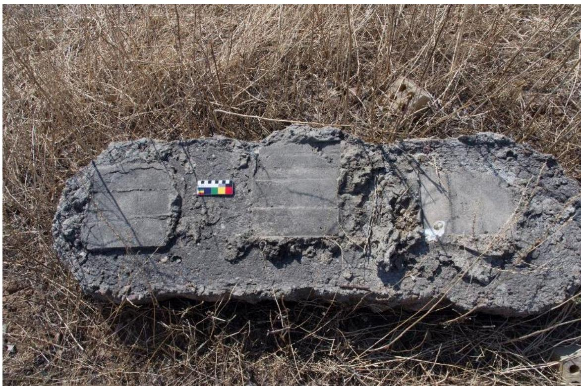
**Figure 21** Detail view of concrete piers showing evidence of the former location of posts
