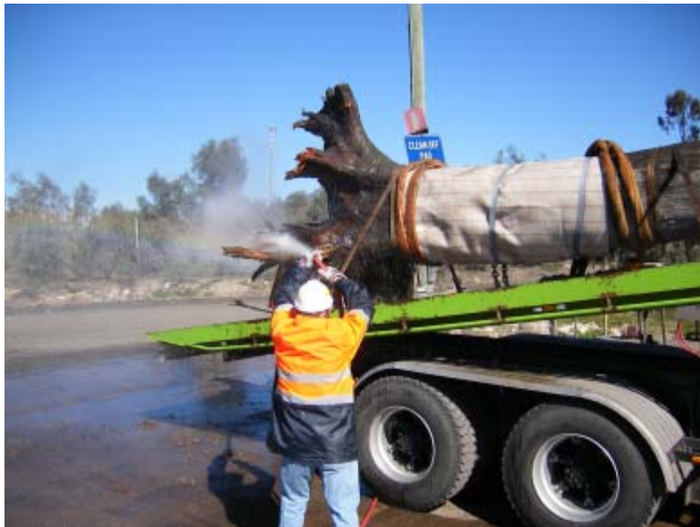
(Fig.11 – High-pressure hose used clean root crown)
