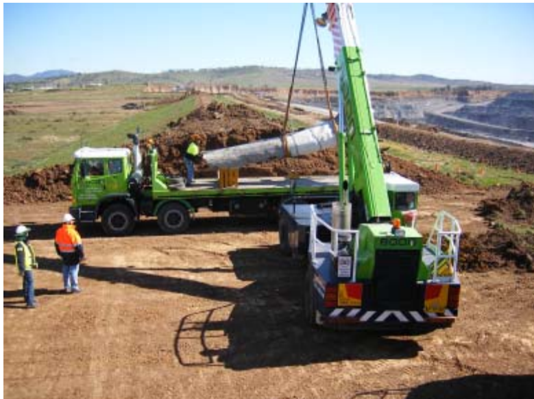
(Fig.9 – Crane lowers the tree onto the truck for transport to the storage area)
