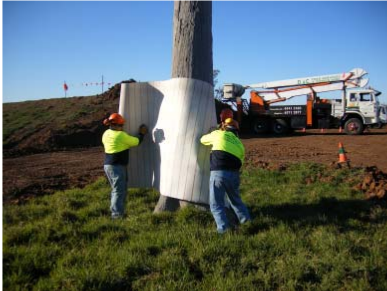
(Fig.2 – Arborist installing carpet belt around butt of tree to protect scarred area)
