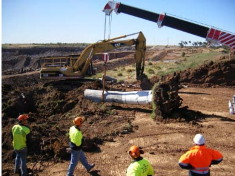
(Fig.8 – Once laid down excess soil can be cleaned from the root crown)
