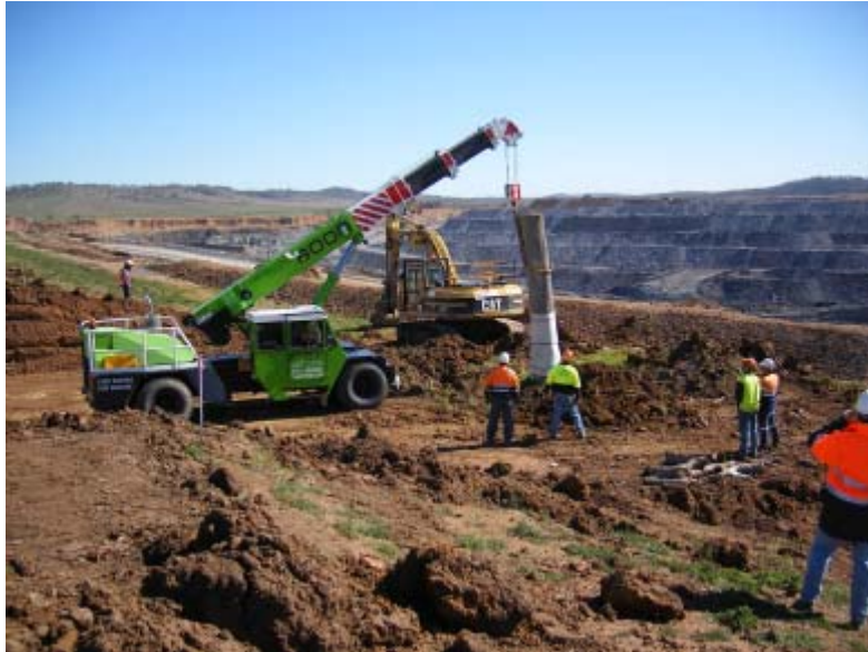
(Fig.7 – Franna crane & excavator working together to dislodge tree)
