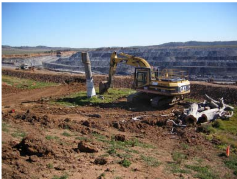
(Fig.5 – An excavator cutting s root trench)
