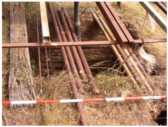
Figure 44 Timber-lined well at MP13
