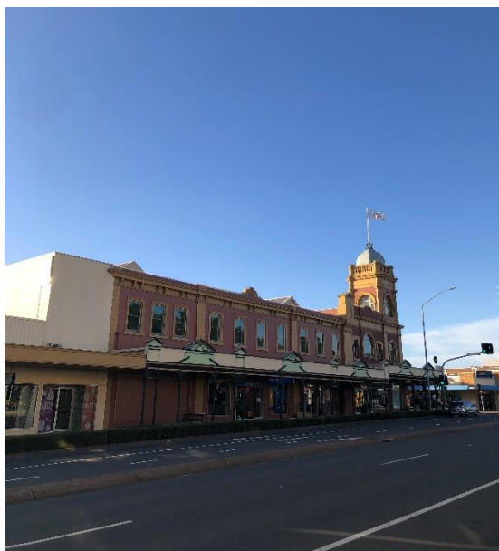
Plate 4-1 Bridge Street Muswellbrook
