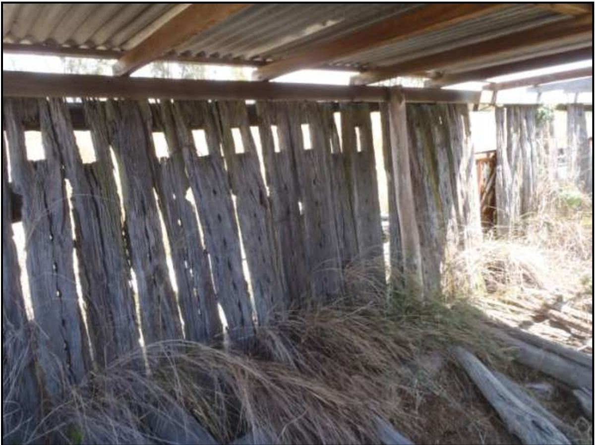
Plate 86: P20. Part of shearing shed showing wall constructed of slit rail fence posts.
