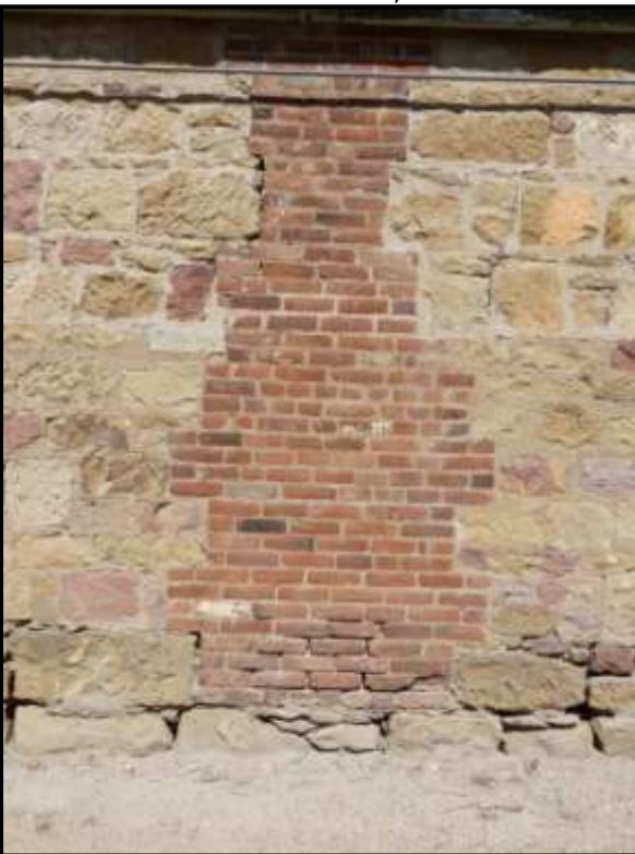
Plate 611: P17. Brickwork in chimney on north east.
