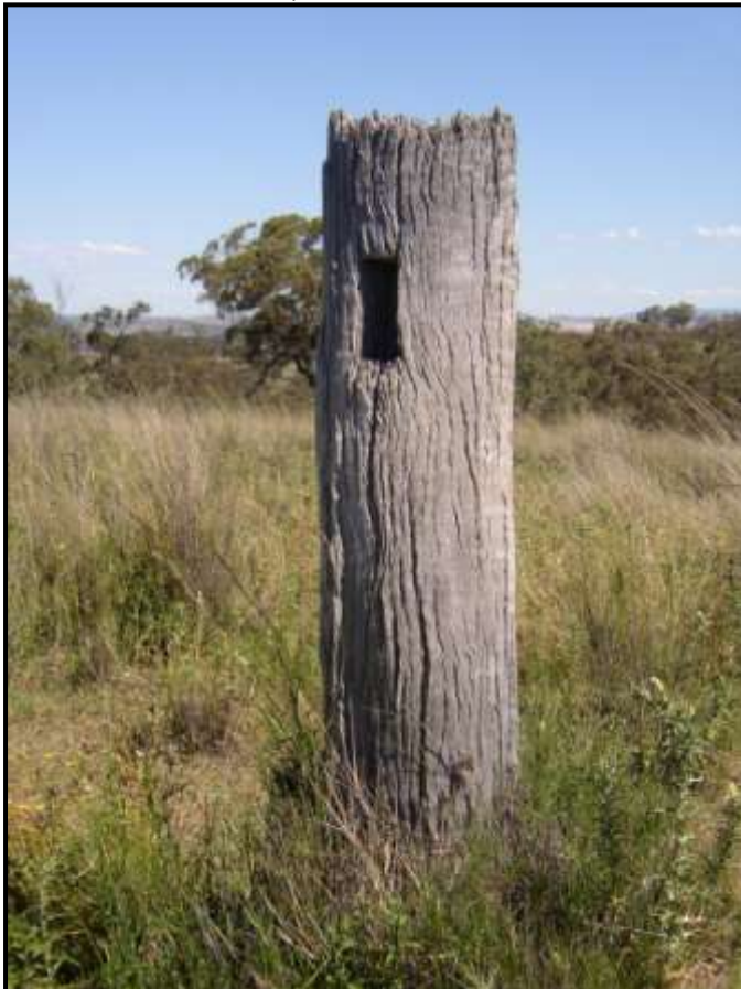
Plate 308: P2. Post shown with single mortise. Fence has been top rail with wires.
