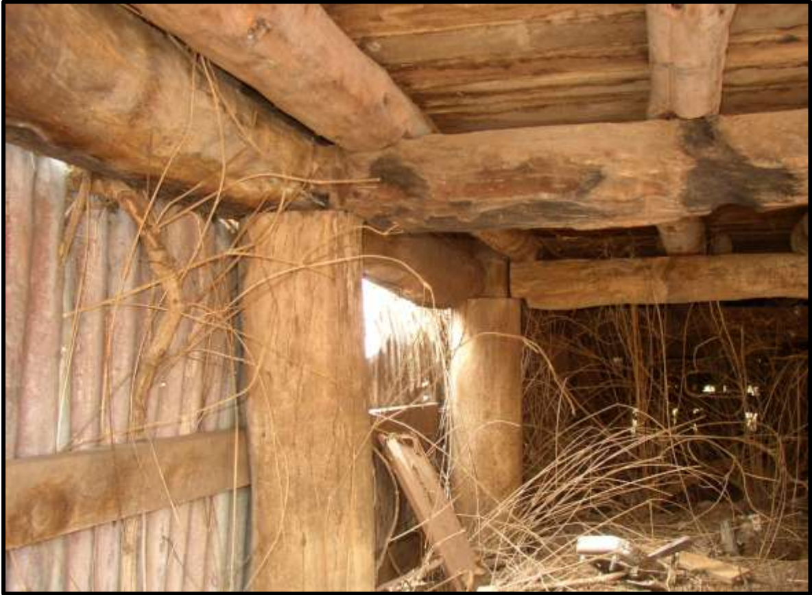
Plate 24: P25 Under floor view of shearing shed showing use of round timber.
