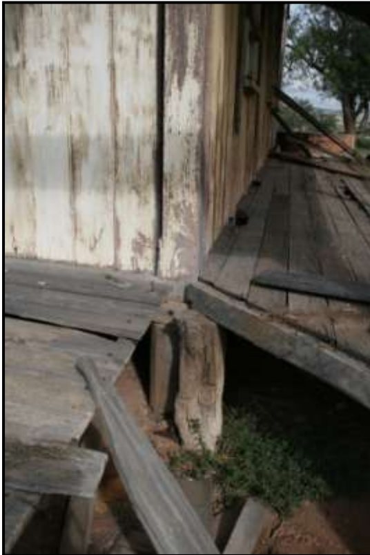
Plate 506: P10 & 14. North east corner showing slabs & earth-fast corner post. View of front veranda with four-pane windows.
