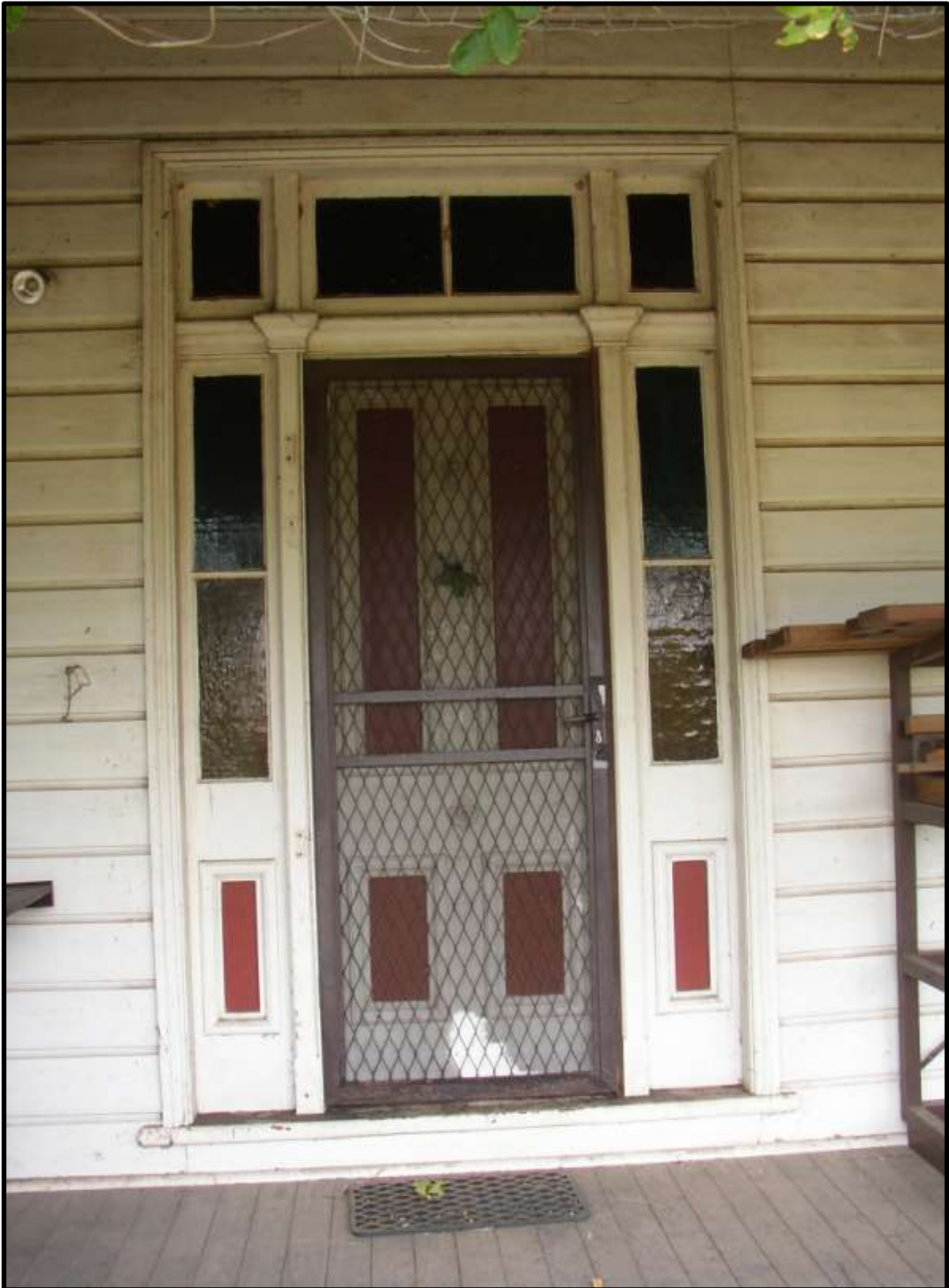
Plate 09: P34 Front door, note glass panels, fan light, decorative timber each side of door and weatherboard style.
