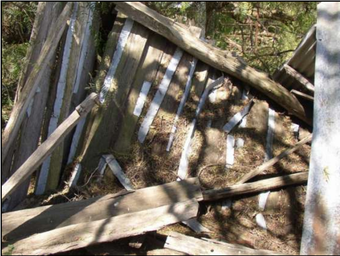
Plate 343: P12. Part Site B, possible lean-to. Slabs with metal strips to close gaps.
