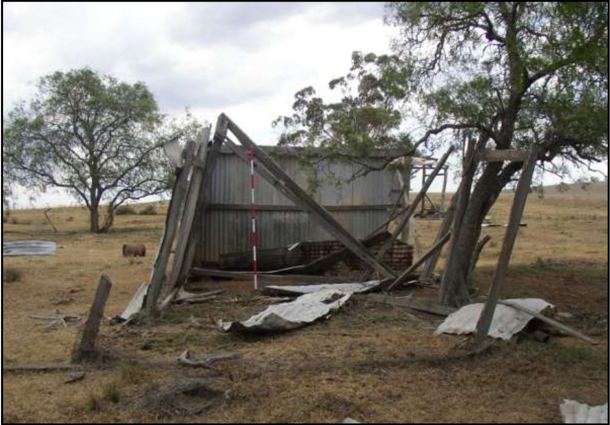
Plate 133: P63. Fowl house looking west. Note beam near scale with mortises.
