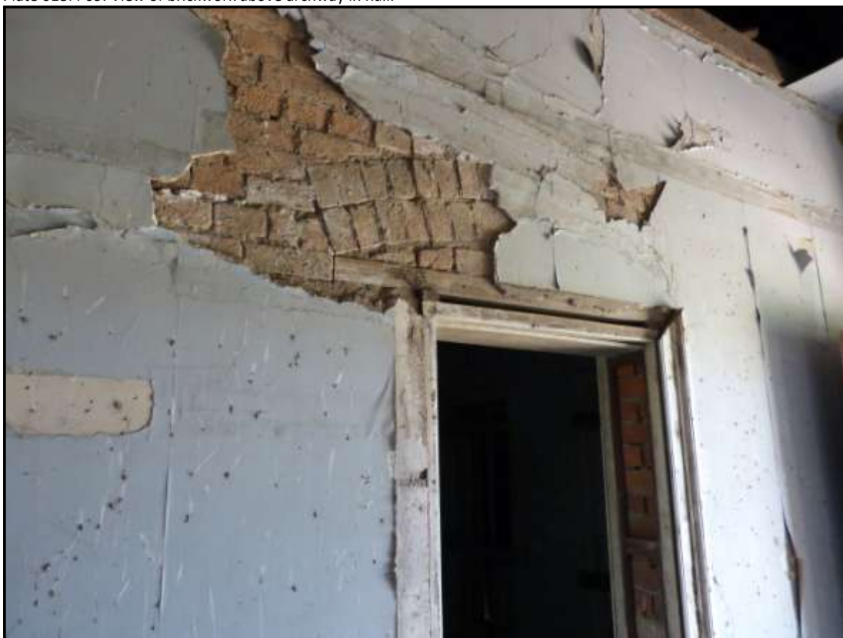
Plate 619: P10. View of timber lintel and ached brickwork above doorway.
