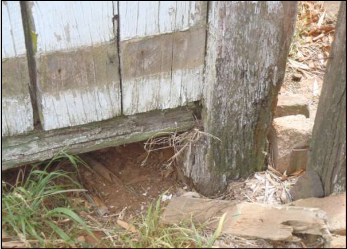
Plate 460: P42a. Earth fast post on south east corner of detached room.
