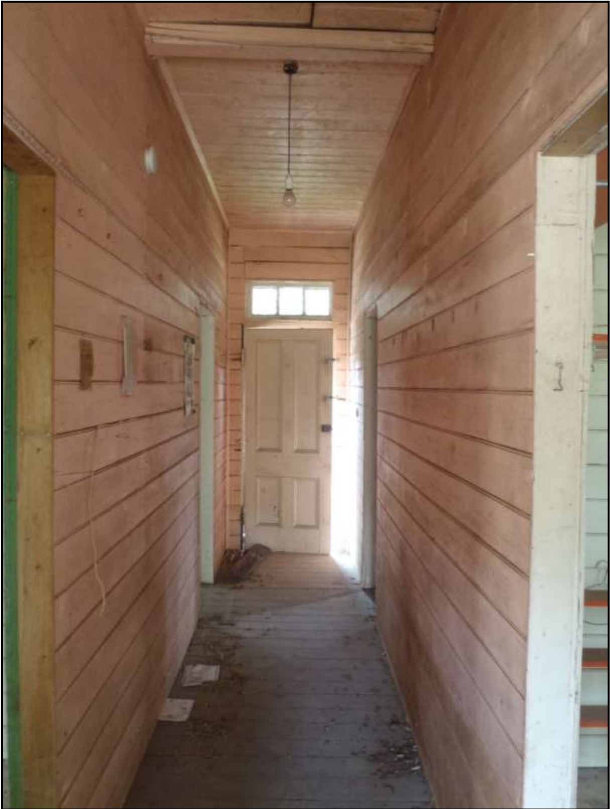
Plate 453: P36. View of hall looking towards front door. Note lack of skirting boards or architrave around doorways.
