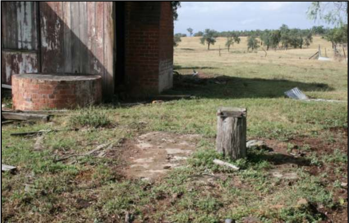
Plate 503: P04. Block for separator and concrete slab, remains of dairy. Note brick tank stand and vertical slab walls.
