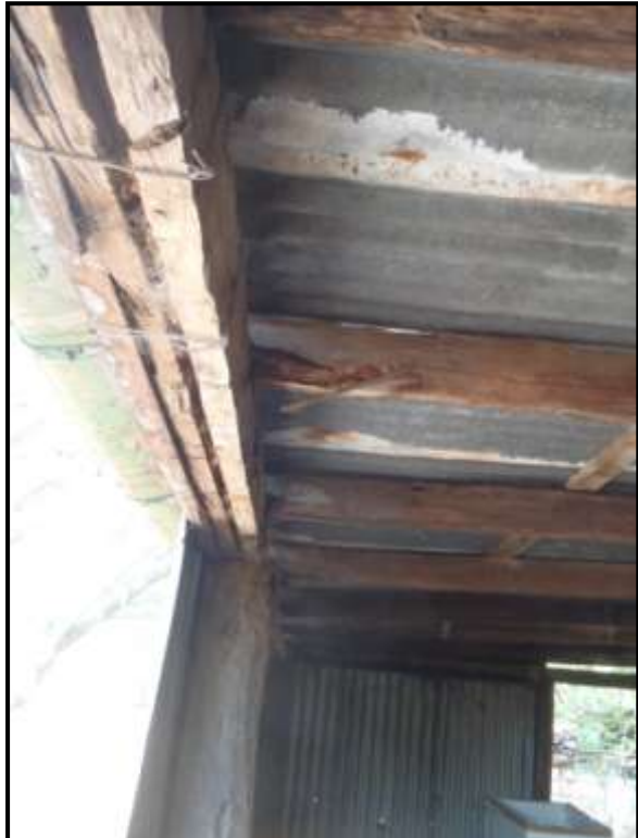
Plate 459: P145 & 146. Frame of car shed utilising recycled material. Beam above came from slab building.
