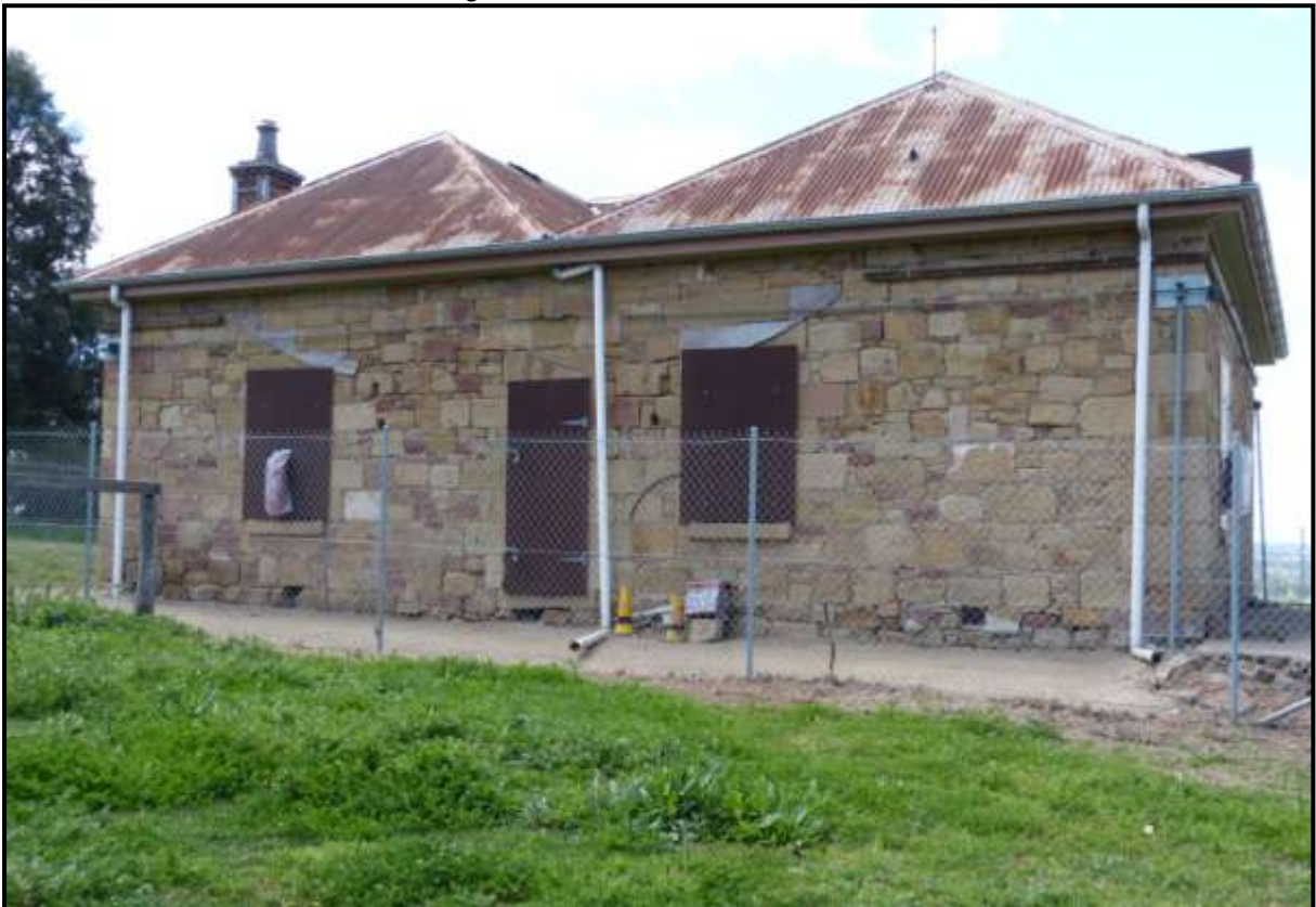
Plate 608: P01. View of west or rear of building. Evidence is visible in the stone where the veranda and covered walkway were attached to the building.
