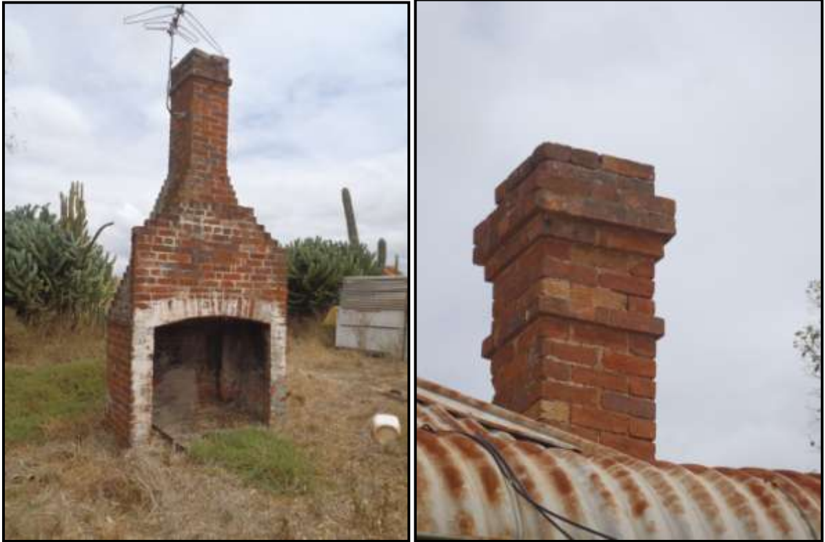
Plate 462: P46 & 49. View showing chimney style and bricks used.
