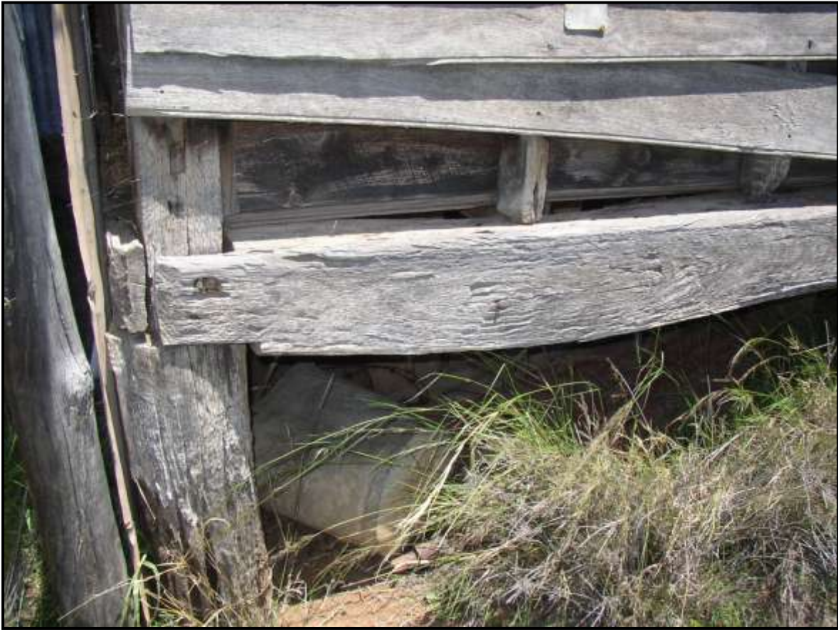
Plate 298: P5. Example of how bearers are mounted and secured to earth fast posts.
