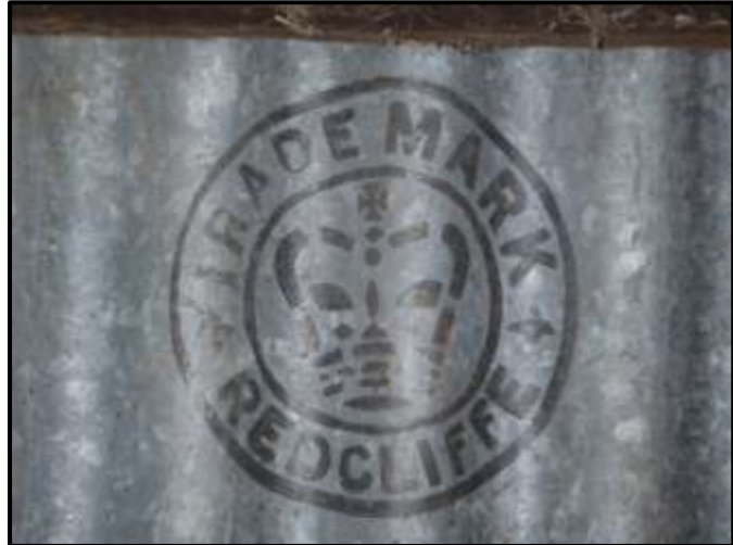
Plate 538: P199. Brand on corrugated iron in south end of hall
