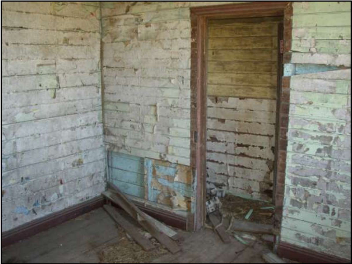
Plate 300: P7. Evidence of wallpaper and painting on back of hall lining.
