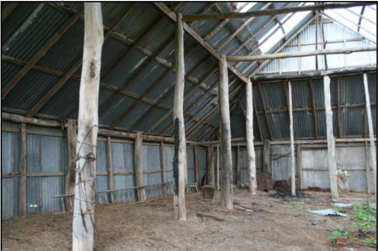
Plate 487: P46. E Hay shed. Note pole construction.
