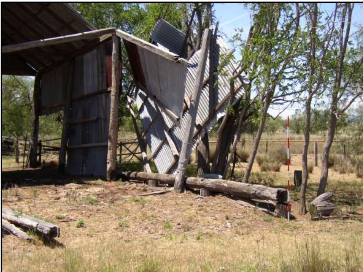
Plate 233: PE5. Heavy bed log in shearing shed portion of Area E.
