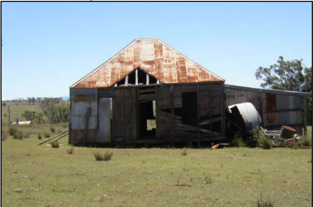
Plate 295: P1. Back of house looking north. Note roof line that indicates another part of the building extended from here.
