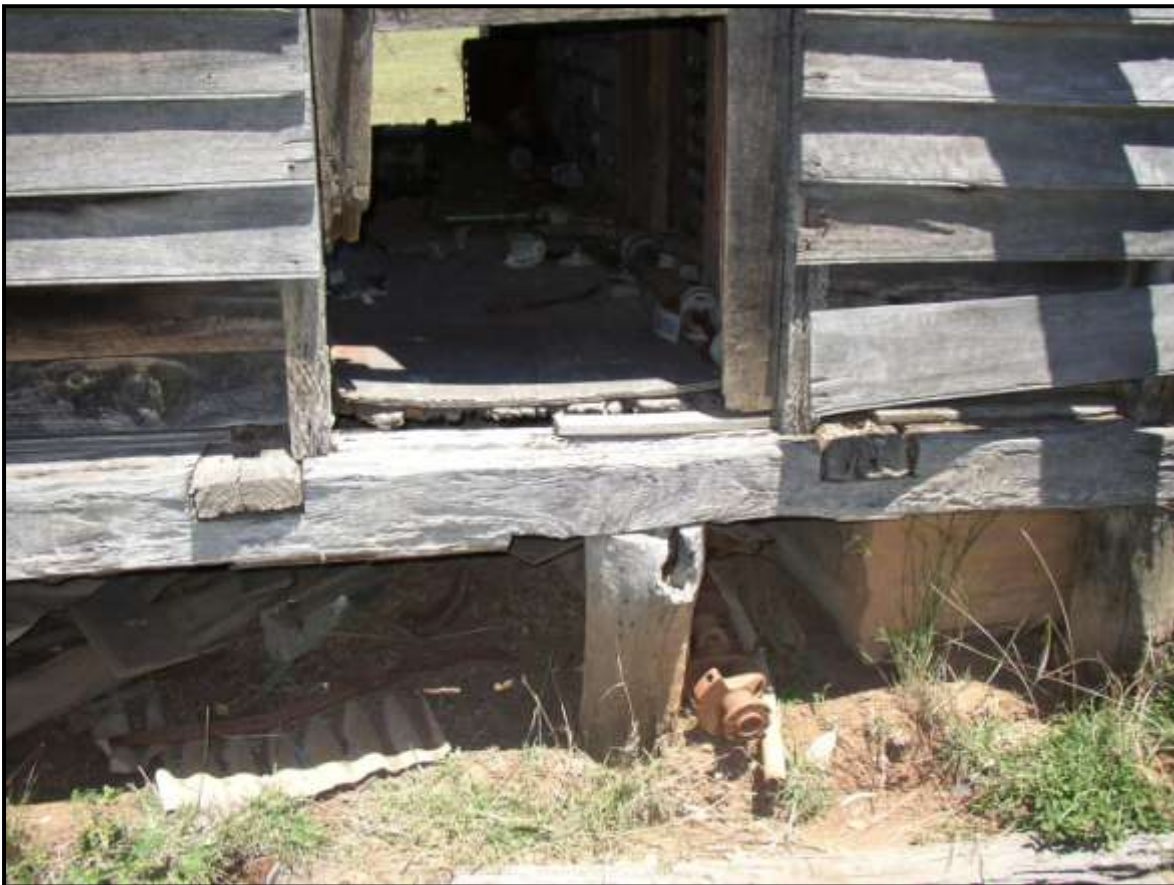
Plate 297: P4. Front door. Note how joists are let into bearers. Also beading on weatherboards.
