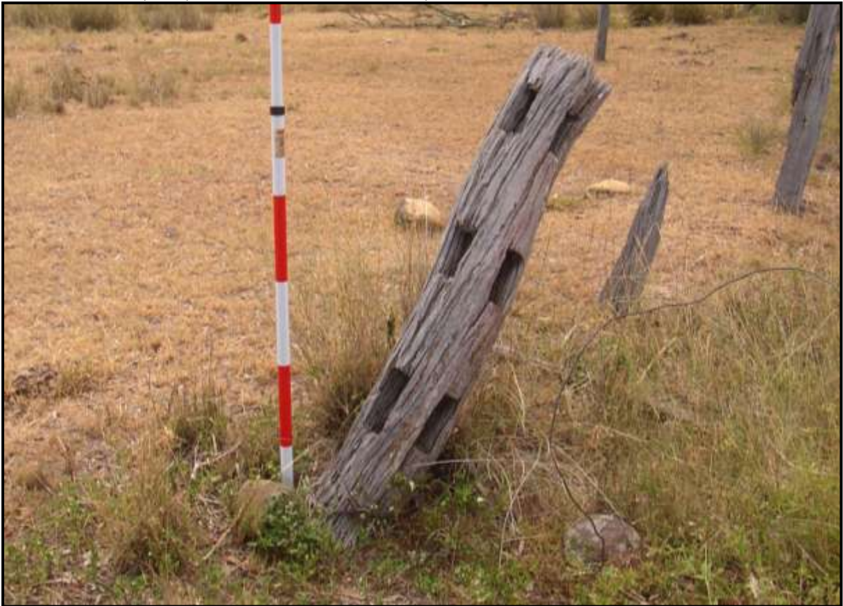
Plate 154: P40 Example of post on site mortised to take three rails at a corner.
