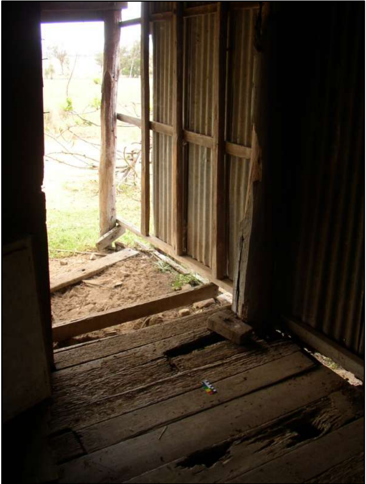
Plate 38: P06 Front doorway. Note width of floorboards, rough bush timber, corrugated iron walls.
