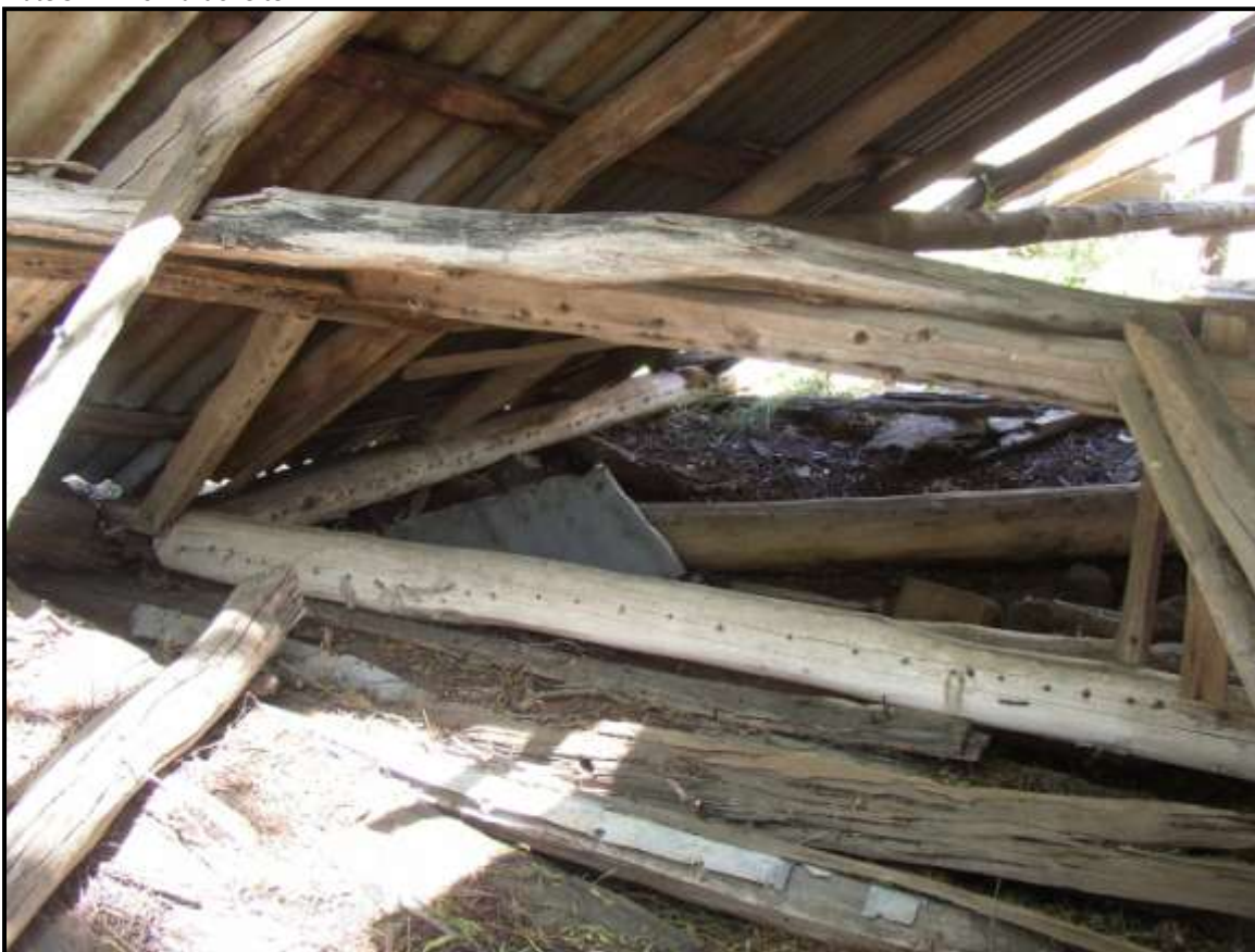
Plate 342: P12. Part of Site B. Note clouts on rafters where material has been held on.
