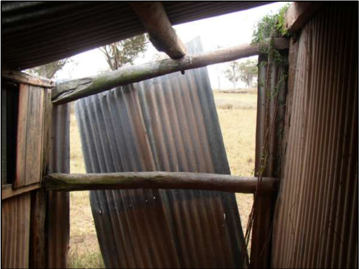
Plate 39: P05 Narrow room across the back of the main room. North wall of bush timber and corrugated iron. Iron had been painted to improve appearances.
