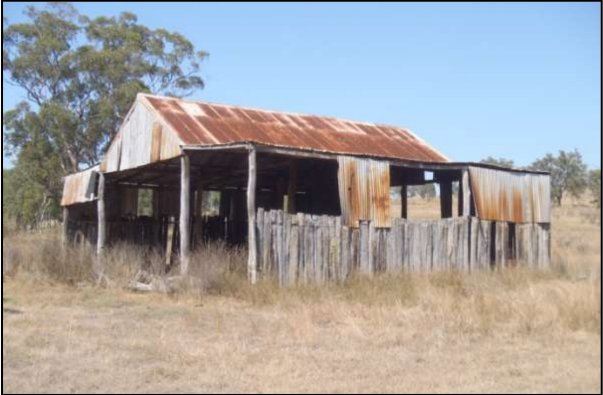
Plate 554: P137. Hay shed. Note use of recycled slabs in walls.
