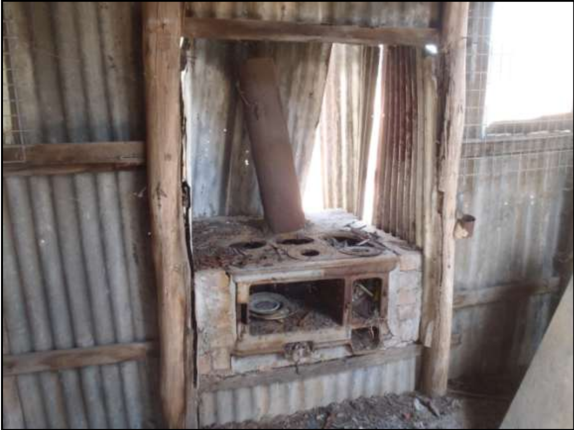
Plate 74: P12. Photograph of stove in hut. Note use of round timber in construction.
