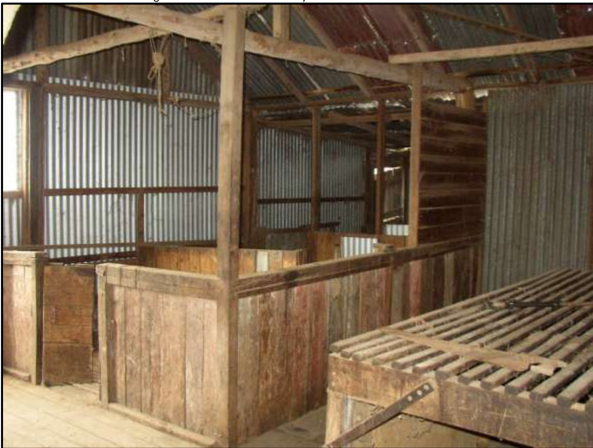
Plate 269: P2.9. View in shearing shed of catching pens. Walls made from split slabs.
