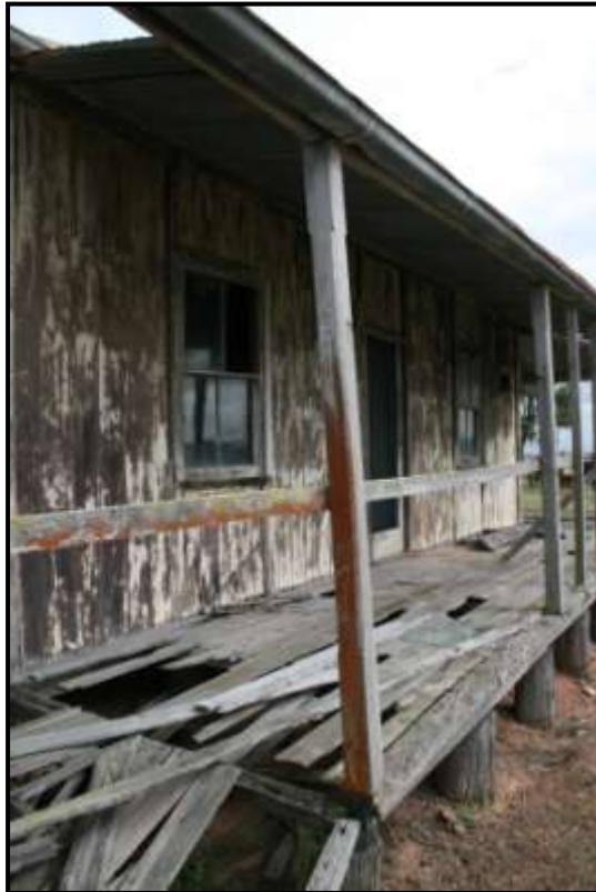
Plate 506: P10 & 14. North east corner showing slabs & earth-fast corner post. View of front veranda with four-pane windows.
