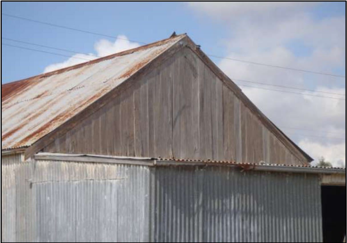
Plate 525: P202. Timber gable at north end of hall.
