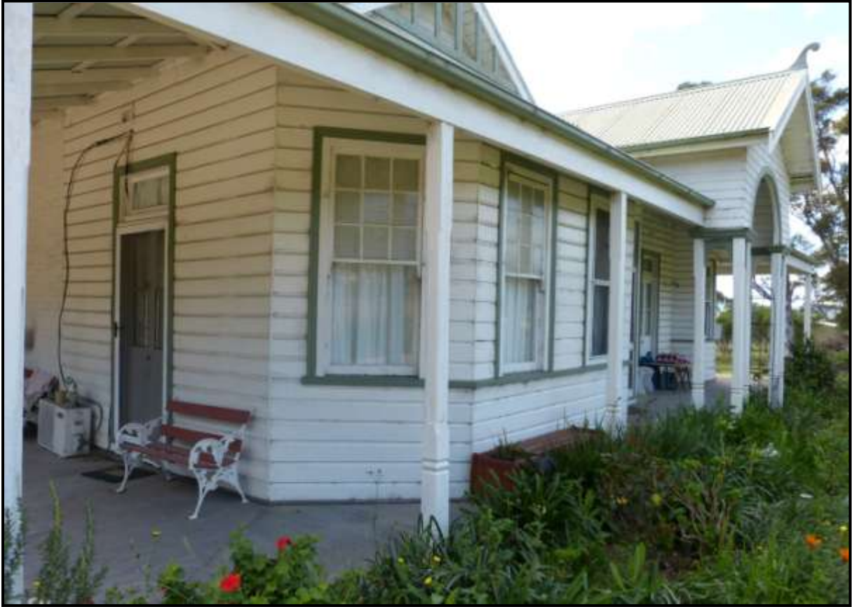
Plate 367: P20. View of large bay window. French doors on left are same as in Plate 360. Note decorative veranda posts and window style.
