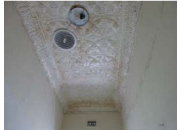
Plate 380: P10. Wunderlich ceiling in bathroom
