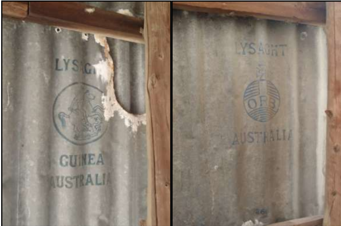
Plate 76: Brands of Lysaght corrugated iron used in hut. The Guinea sheet on the left has been recycled from another building.
