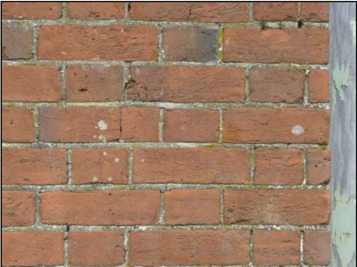
Plate 432: P31. Example of Flemish bond in south wall of 1845 section.
