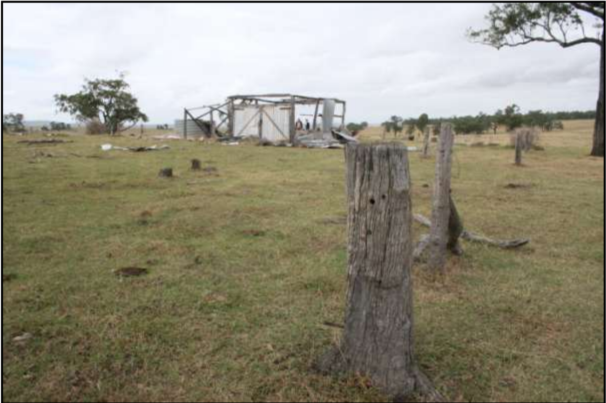
Plate 516: P23. Tree cut off in situ and utilised as a strainer post.
