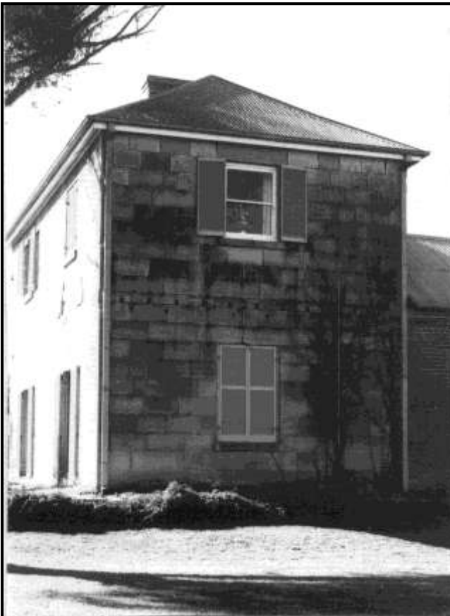
Plate 422: Southern end of sandstone section of homestead. Hole in wall shows where veranda was mounted. T Tame 1976.
