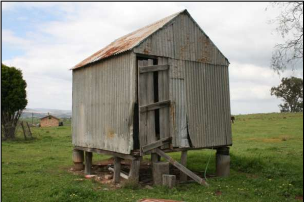
Plate 489: P59. G Shed. Note metal around piers. Dairy J in background.
