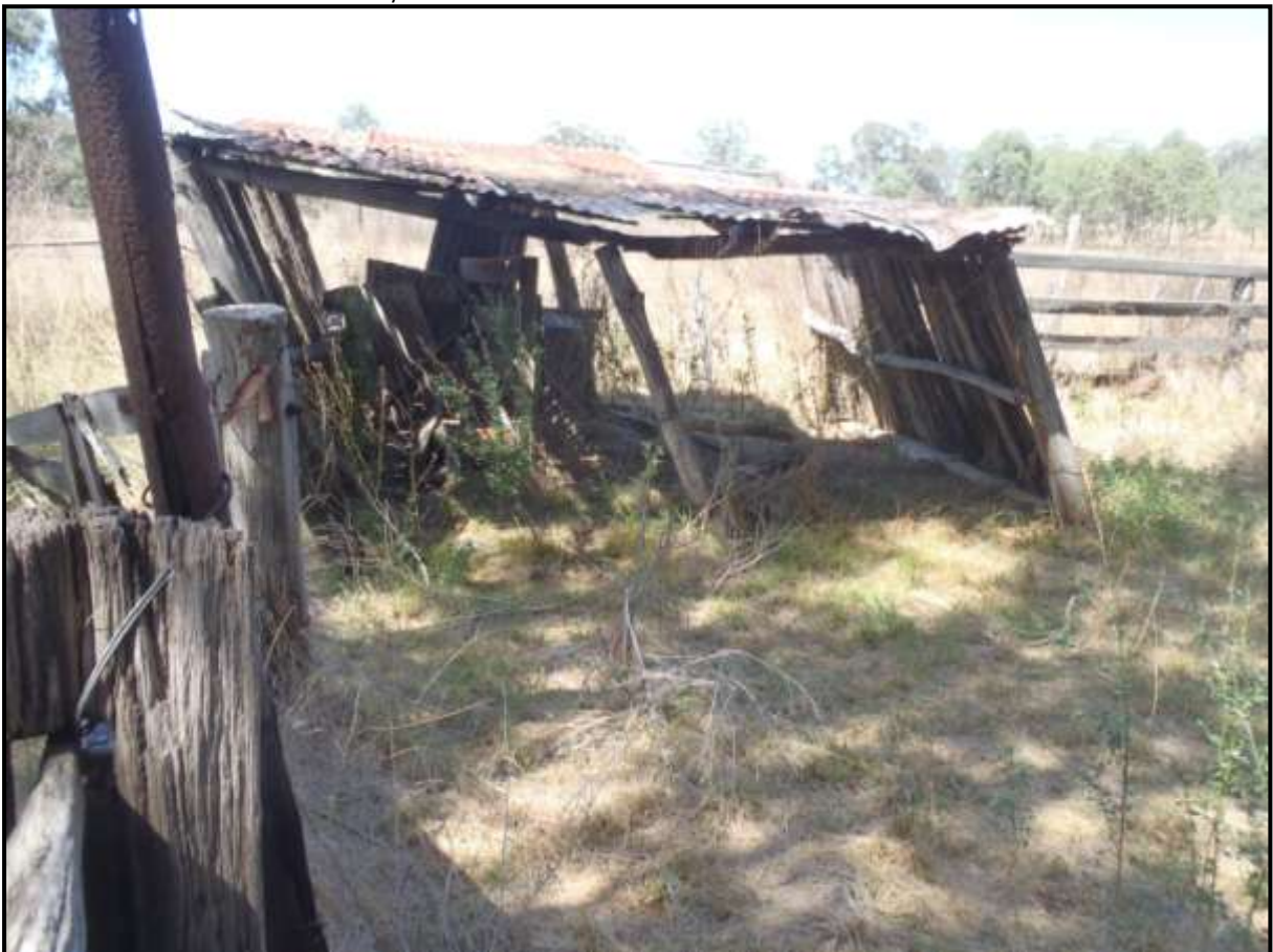
Plate 553: P141. Remains of cow bails. Note use of recycled slabs in wall.
