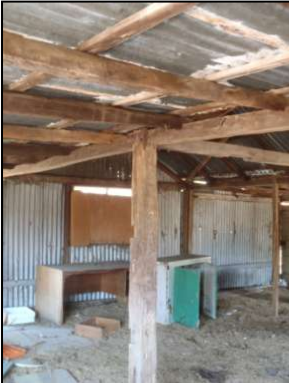
Plate 459: P145 & 146. Frame of car shed utilising recycled material. Beam above came from slab building.
