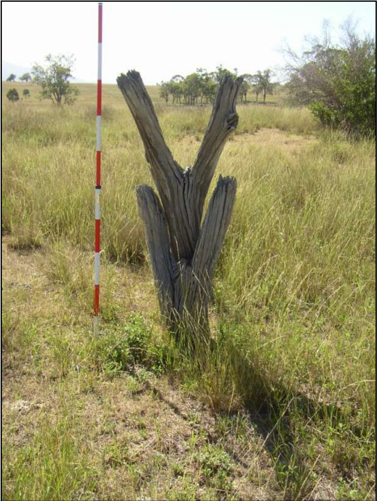
Plate 246: P4. View of forked limbs used as posts.
