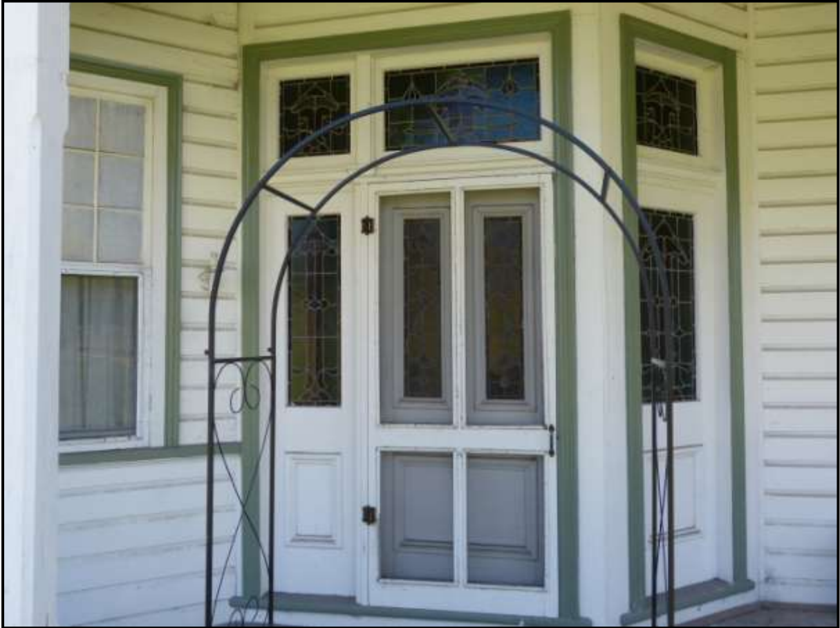
Plate 363: P21. Front door with leadlight panels. Window on left is part of the large bay window.
