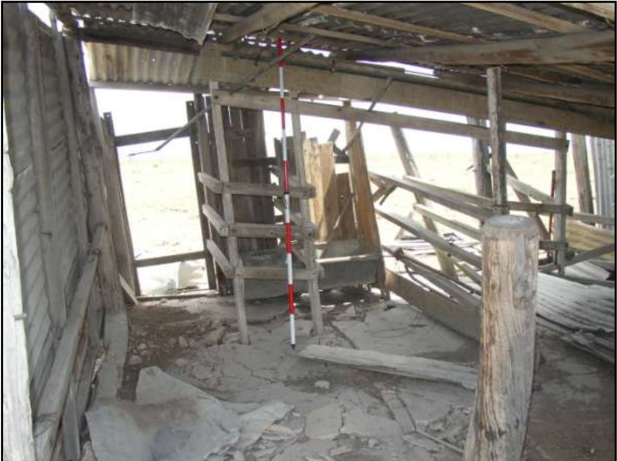
Plate 131: P59. Internal view of dairy. Note use of round timber, beam to carry milking machinery and bails.
