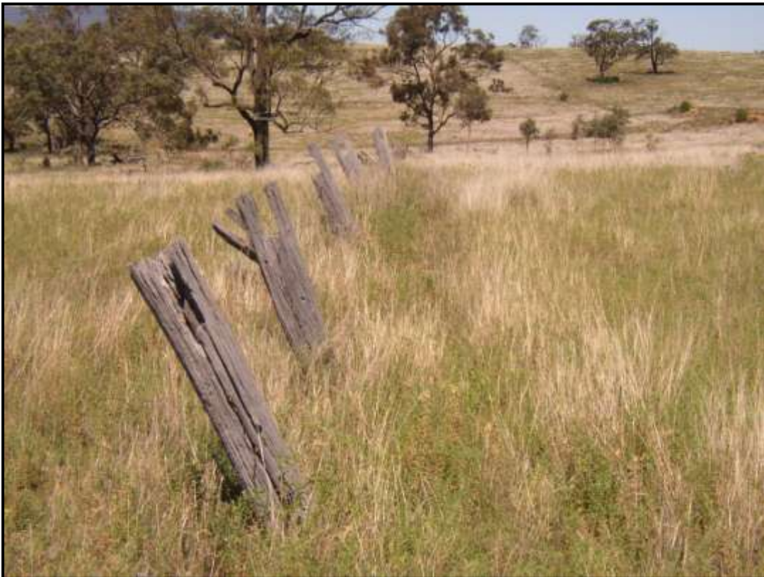
Plate 304: View the fence in 2004, top rail has rotted away.
