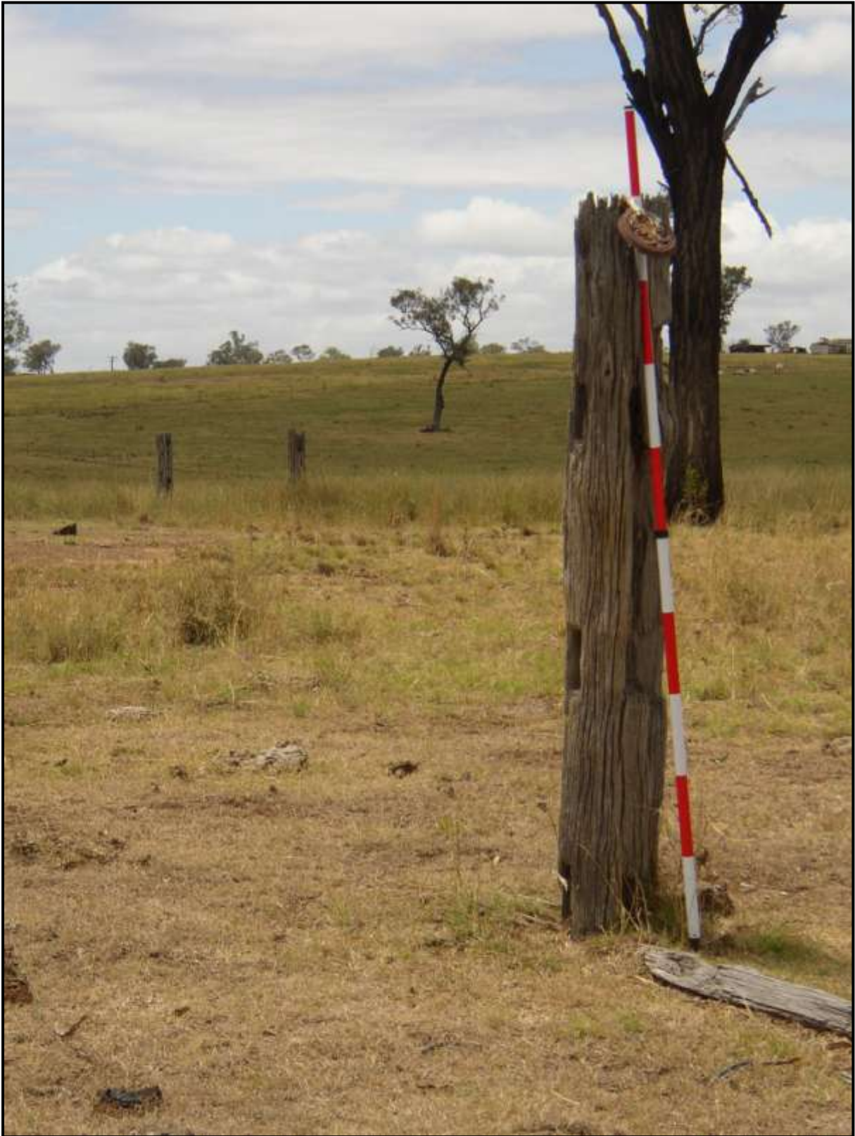
Plate 209: P12.Corner post for four rail stock yard
