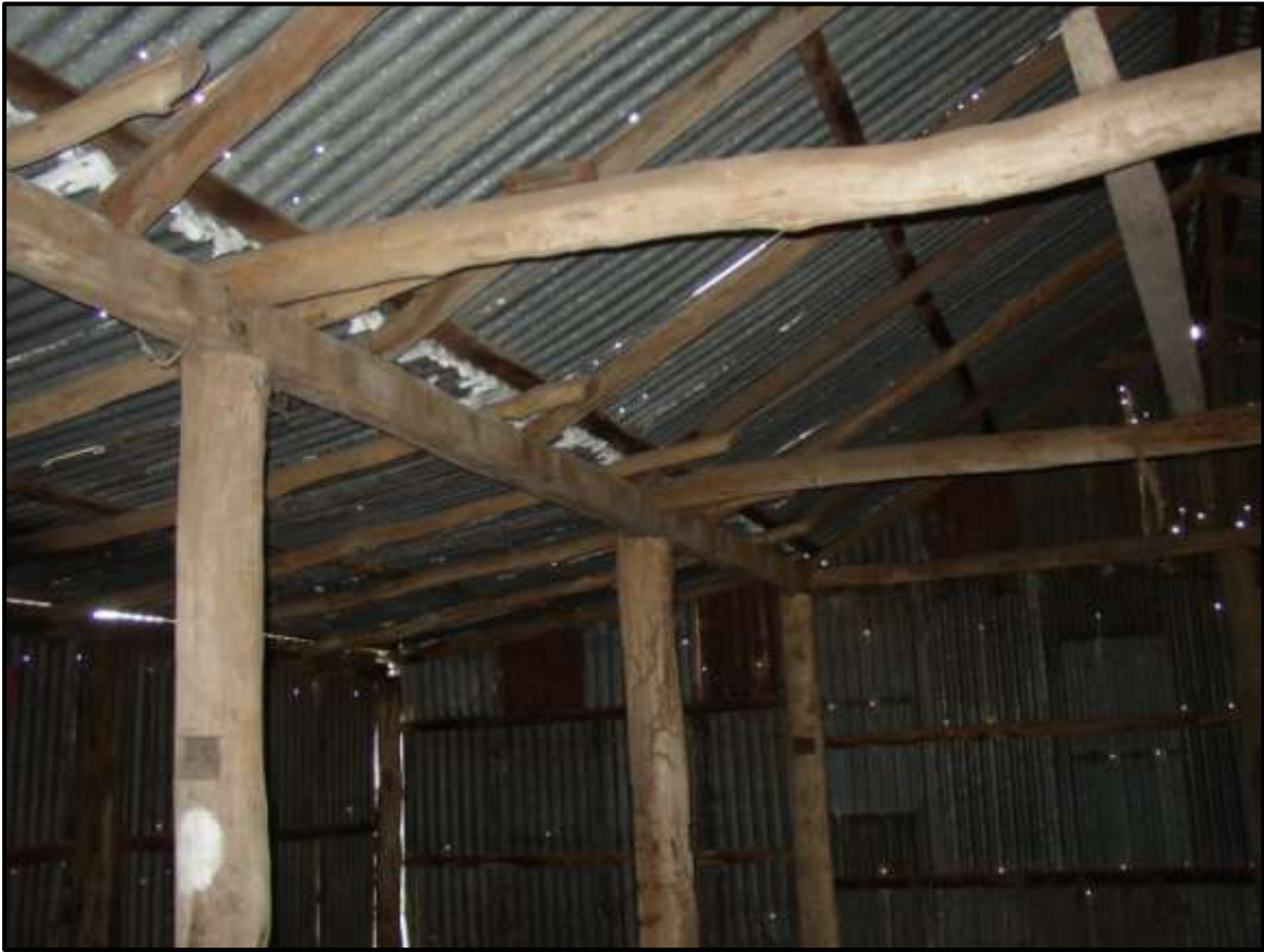
Plate 274: P2.15. Example of frame construction. Note holes in recycled corrugated iron.
