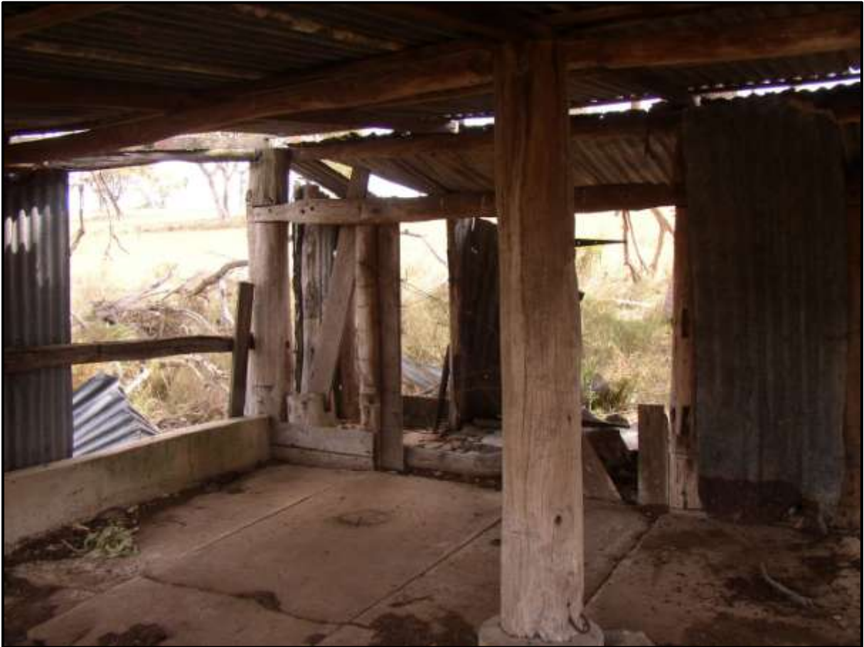
Plate 41: P04 View of part of the dairy. Bail in far corner. Building constructed of bush timber and corrugated iron.
