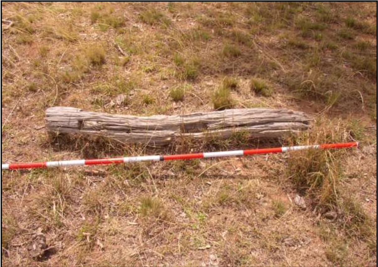
Plate 200: P3. View of mortised post. This is a corner post for two rails.
