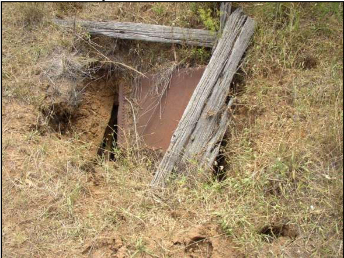
Plate 352: P27 Remains of well. Timber lined, old square tank dumped in shaft.
