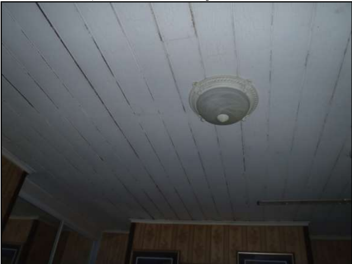
Plate 393: P86. Timber lined ceilings.
