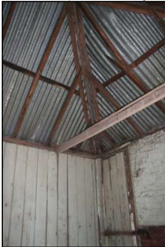
Plate 505: P08 & 12. Roof structure in kitchen and remains of ceiling in hall.
