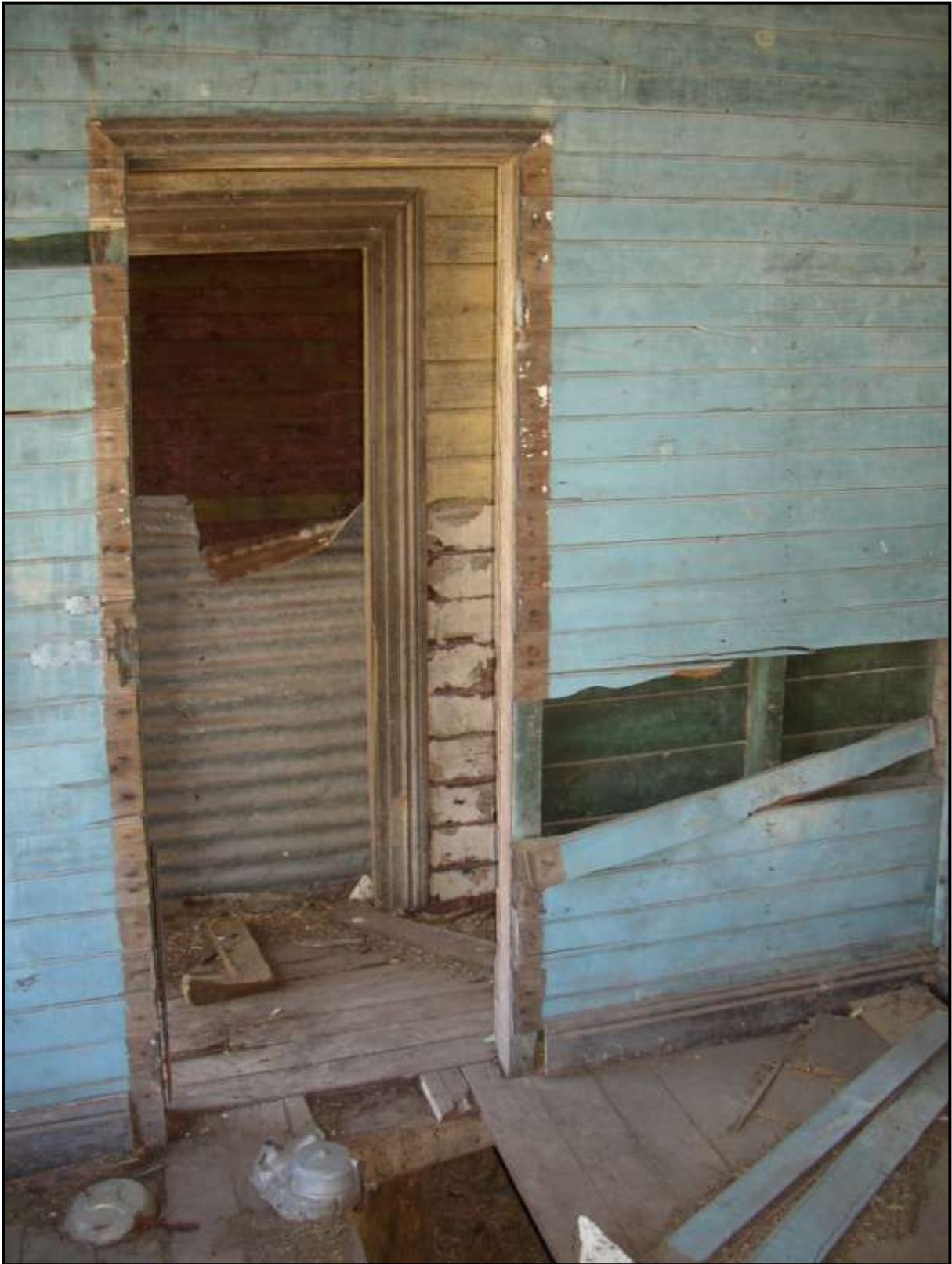
Plate 299: P6 View interior showing part of hall and back of hall lining, changes in lining board and floor board size.
