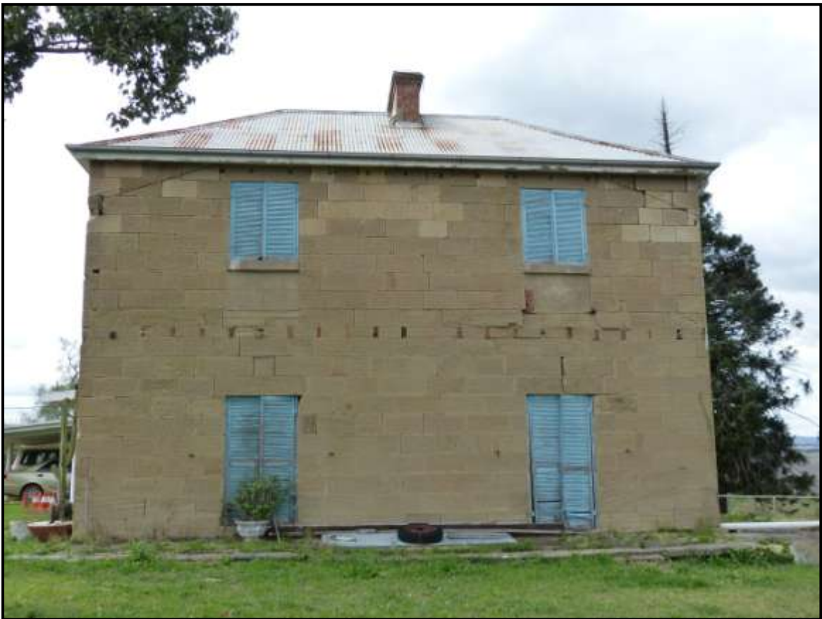
Plate 426: P23. West side of sandstone section. Note holes in sandstone where veranda and balcony were mounted. Also infill on upper French doors.
