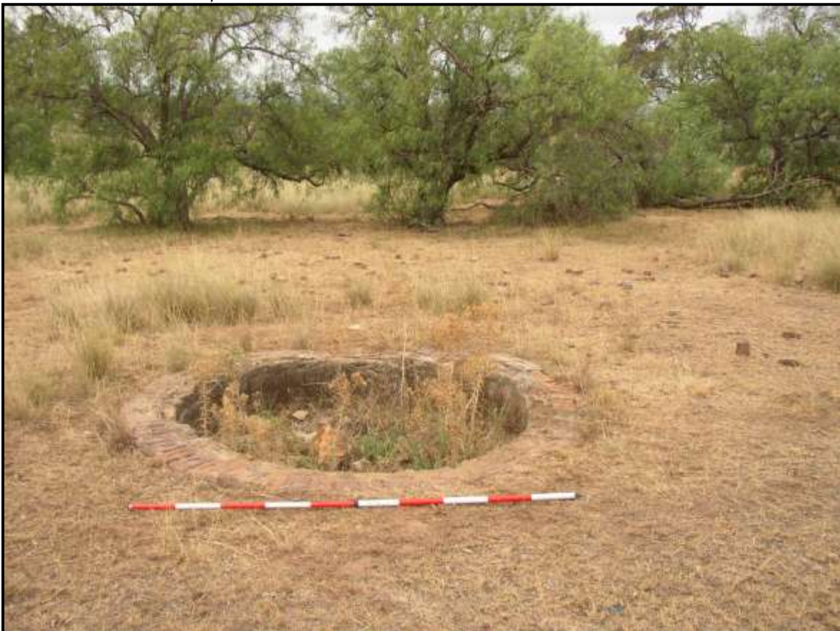
Plate 177: P6. Underground brick tank.
