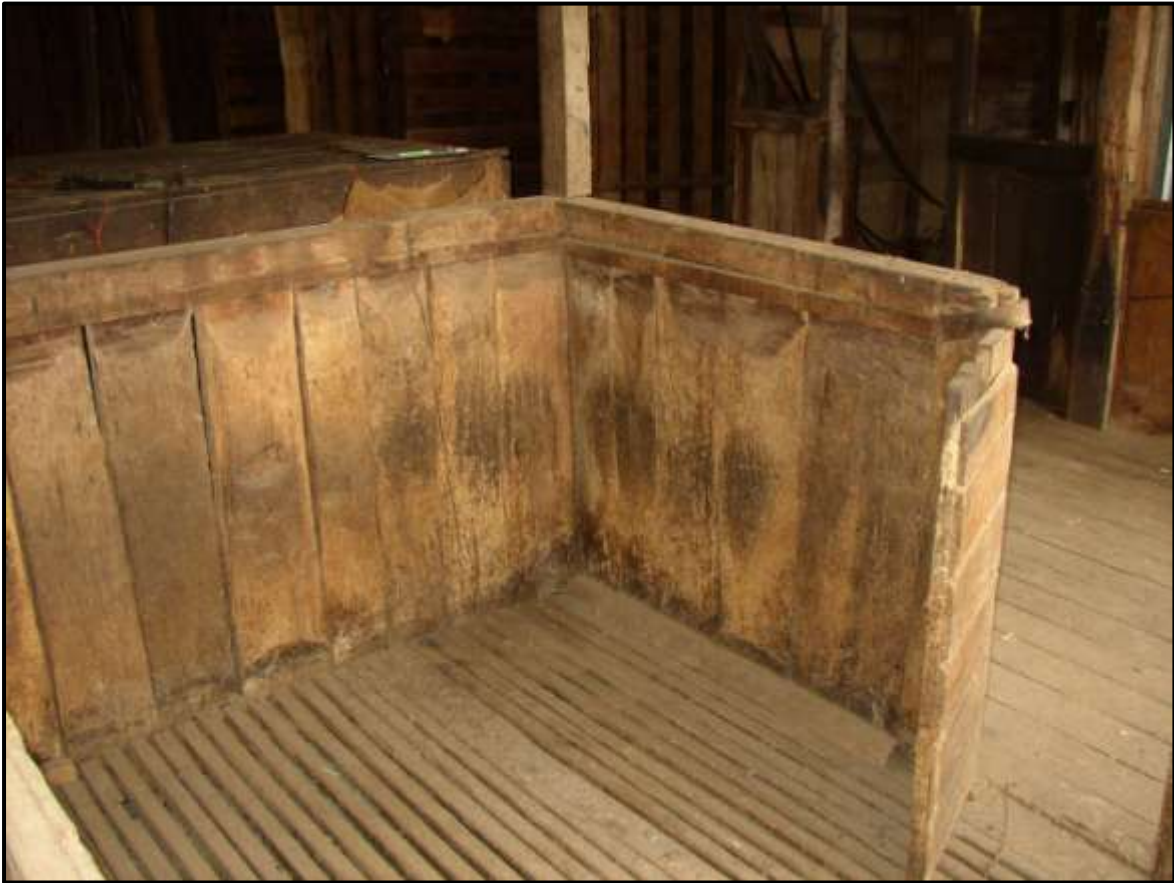
Plate 270: P2.14. View of recycled split slabs in catching pens.
