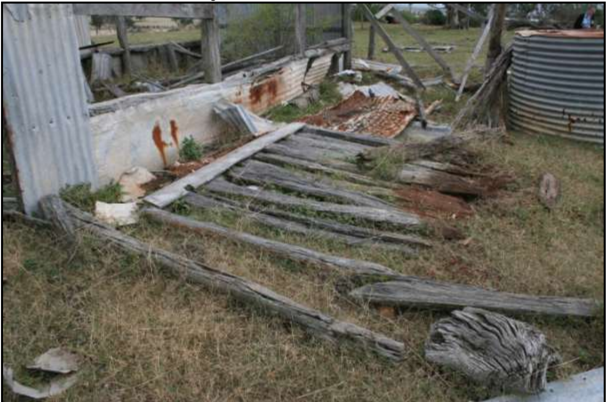
Plate 409: P18 View of slab wall which has fallen.
