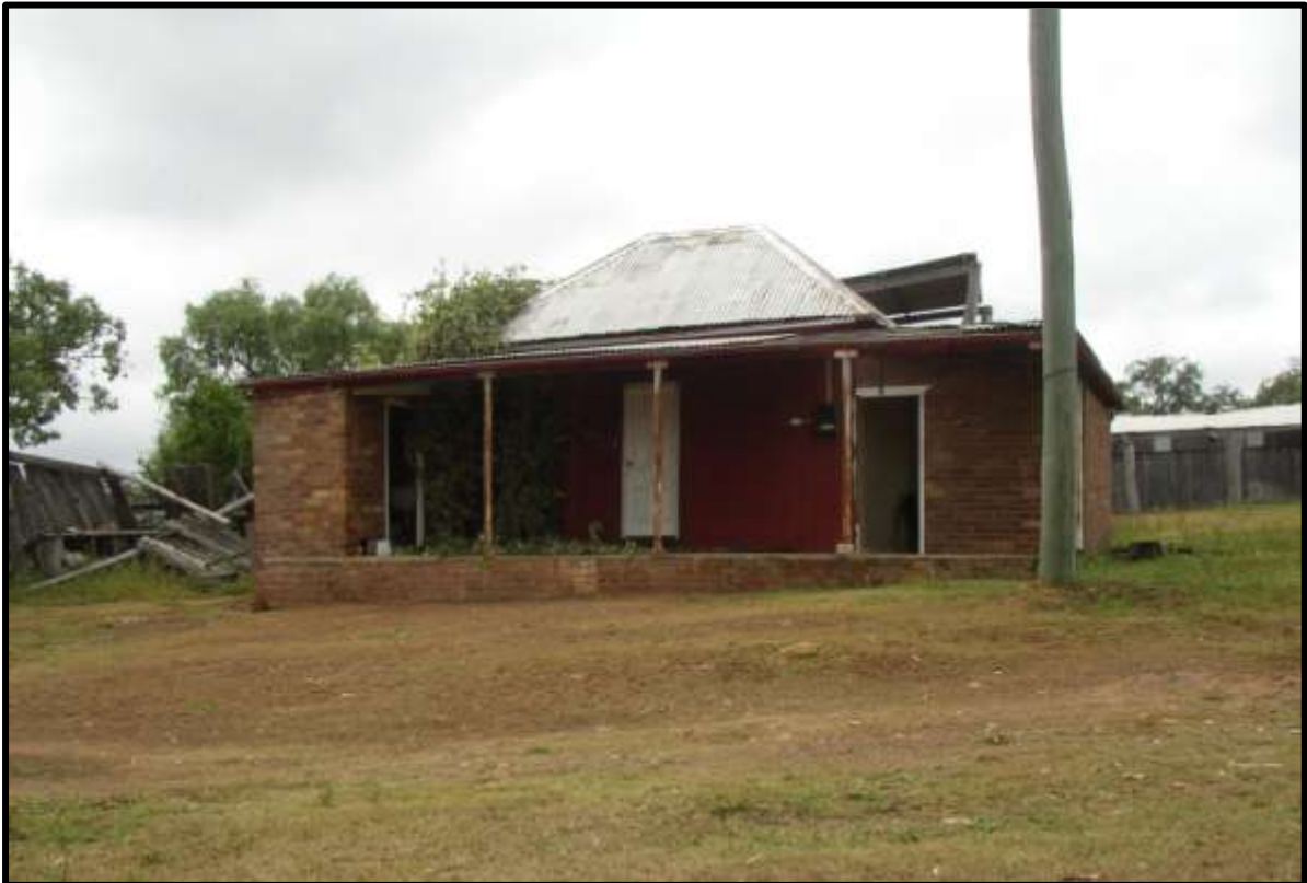
Plate 19: P16 Hut with brick additions on each side. Original section has vertical saw slab walls.
