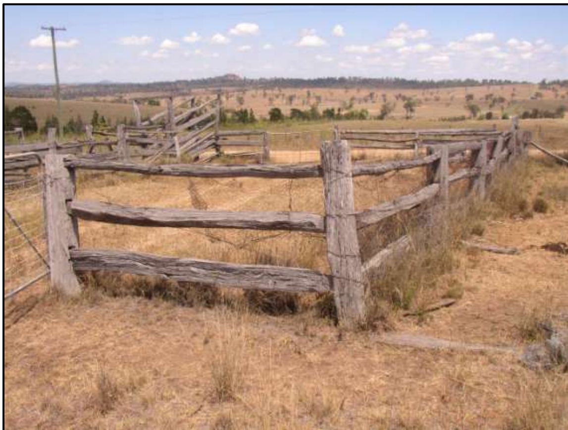
Plate 119: Close up of yard construction. Rails mortised into posts with round top and two split rails
