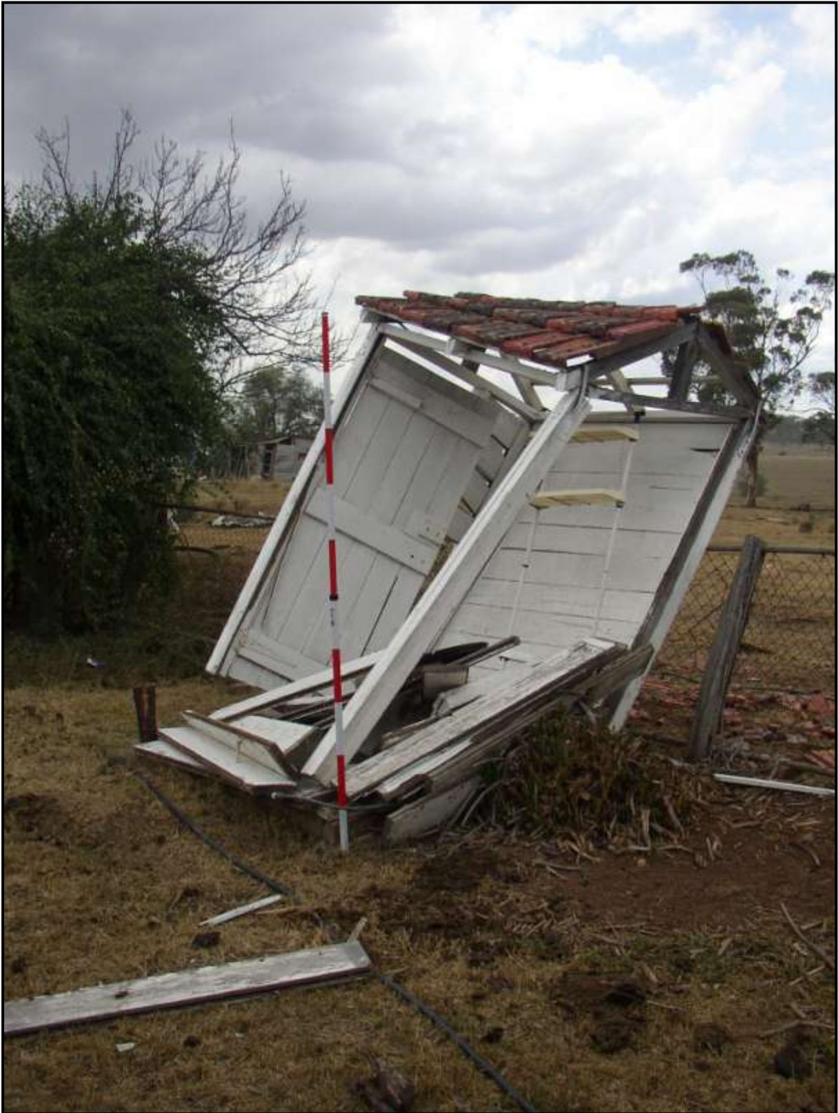
Plate 140: Remains of the toilet. Note thick boards used for walls.
