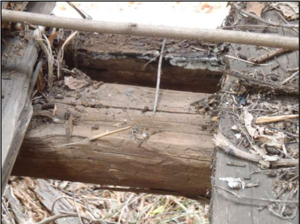
Plate 455: P40. Example of adzed timber for floor joists.
