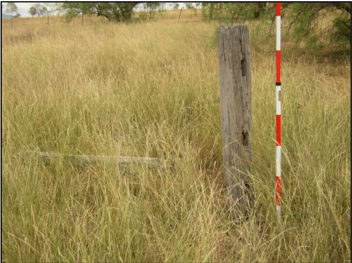
Plate 183: P12. Post mortised for three rails, one post rotted off, may have been gateway to schoolyard from road.
