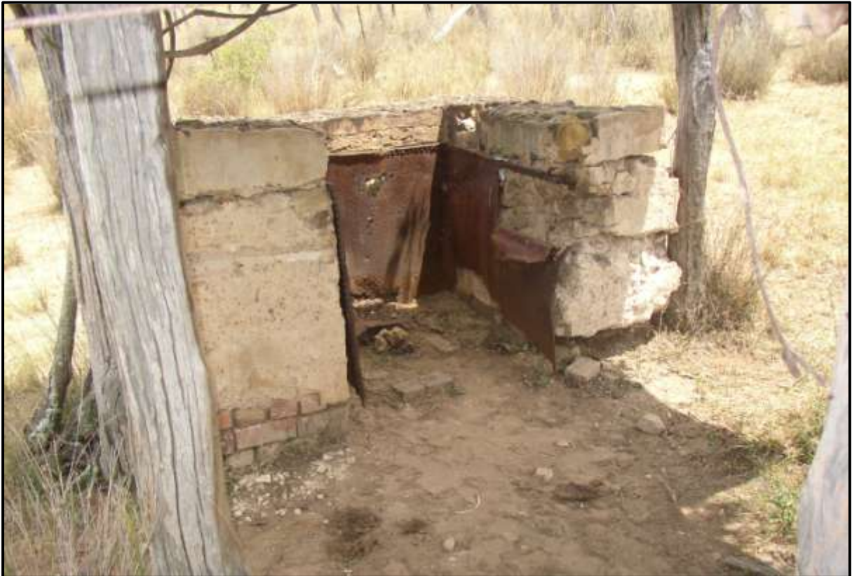
Plate 40: P07 Stone and brick construction at west end of the house. Part of square tank set in.
