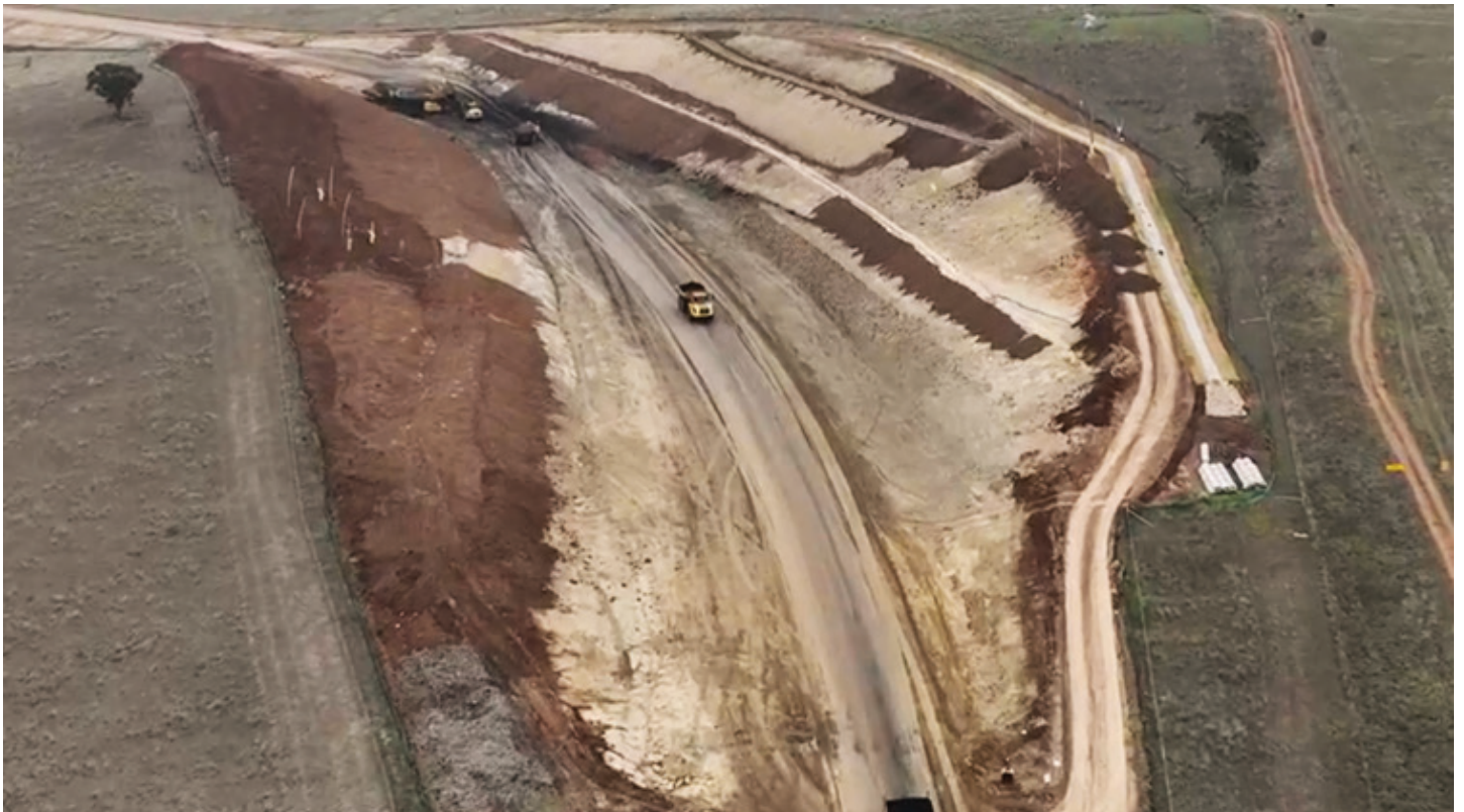
Northern Link Road Works
