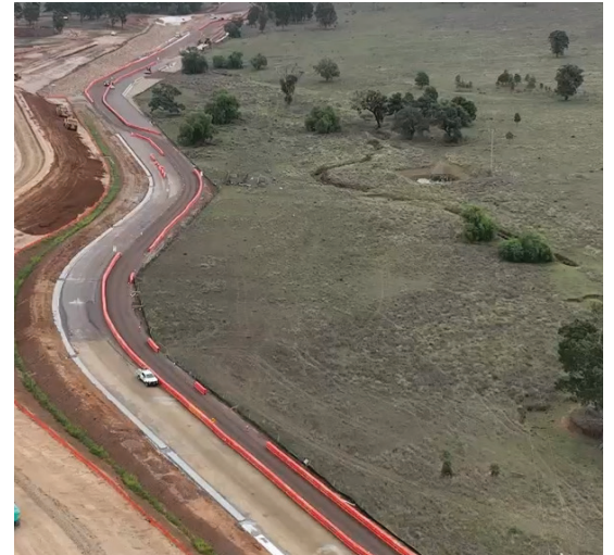
Northern Link Road, Dorset Road Widening
