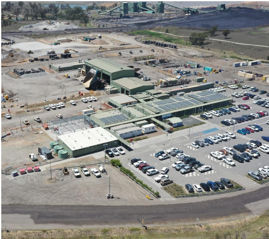
Plate 1 Solar Panels Installed at the MPO Mine Infrastructure Area
