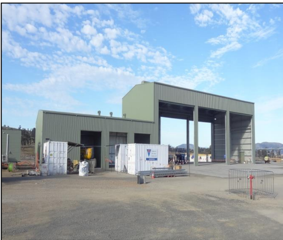
Plate 5: Workshop within the Mine Infrastructure Area.
