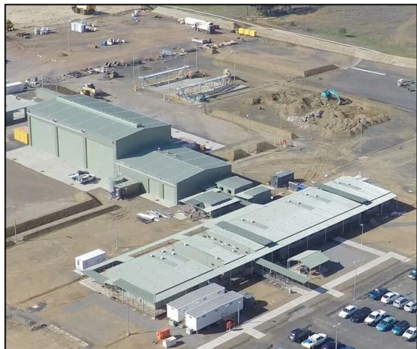
Plate 6: Workshop and associated buildings within the Mine Infrastructure Area.
