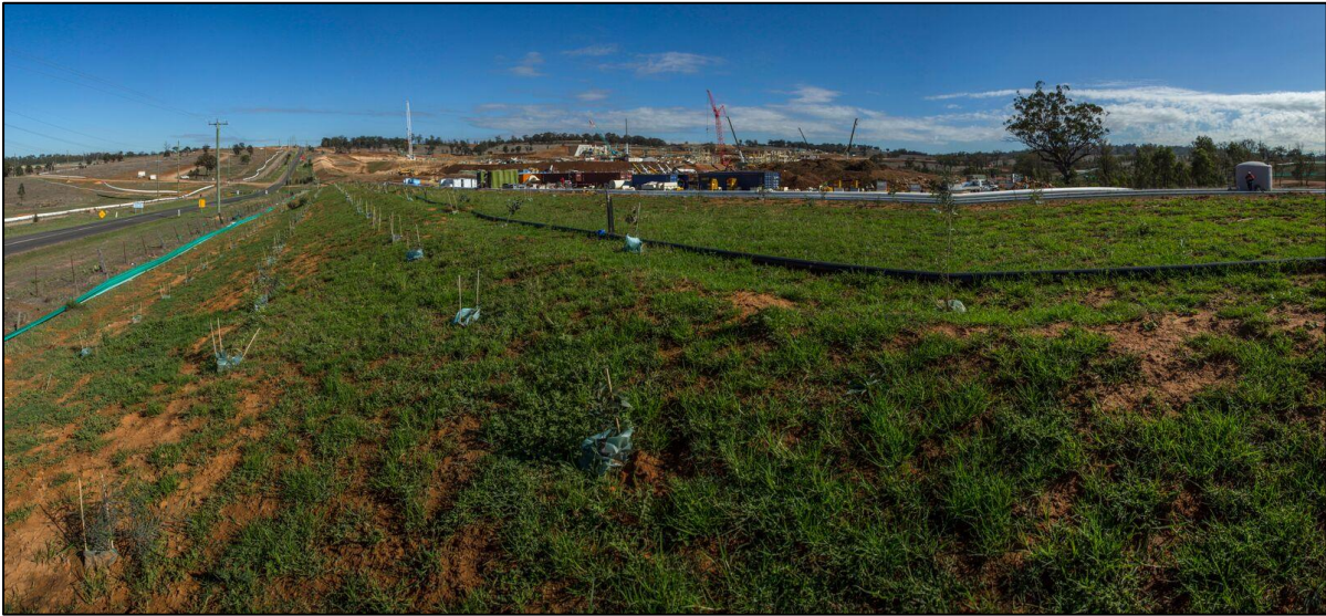
Plate 7: Visual bunding/screen planting along Wybong Road.
