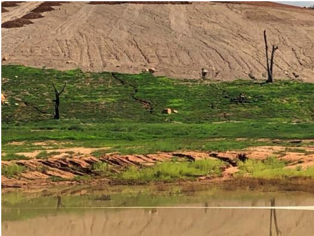
Rehabilitation Photo 4 - Area identified by MACH Energy to require additional rehabilitation works. Evidence provided that since the site inspection this area has been reworked
