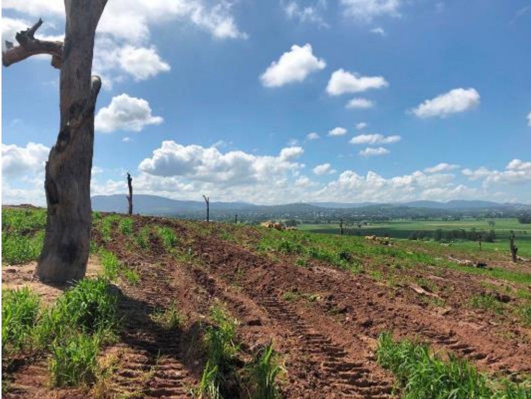
Rehabilitation Photo 3 - Recently shaped and rehabilitated area
