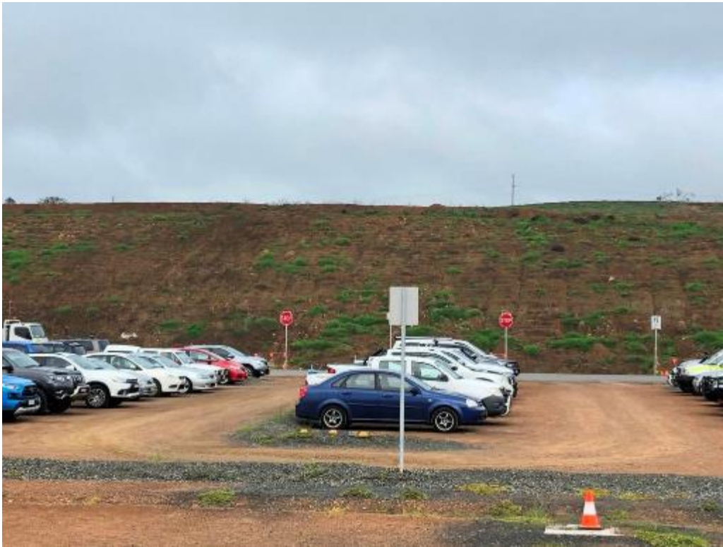
Erosion Photo 1 - Rill erosion in box cut area (near the carpark)
