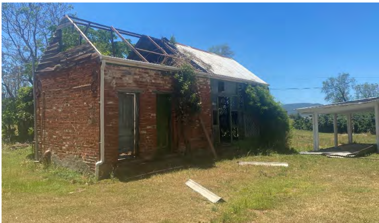
Figure 22. The servants' quarters, showing some of the damage sustained to the roof as a result of a storm event in December 2020.
