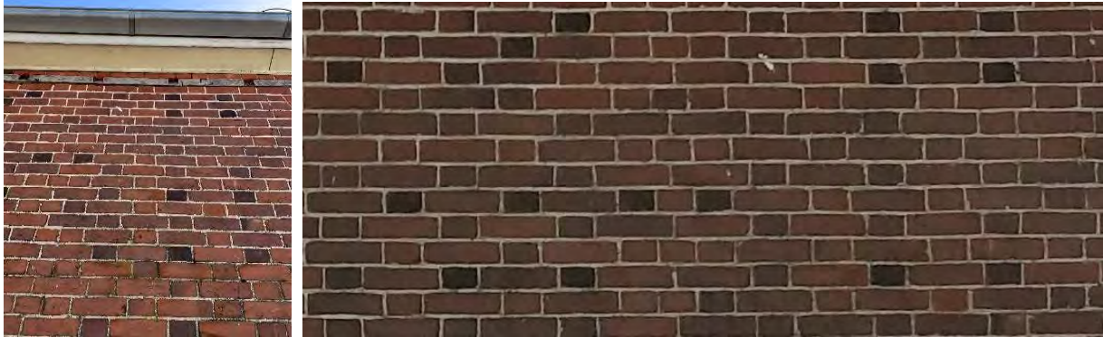
Figure 46. Detail of the brickwork on the southern elevation of the 1840s brick section of the homestead showing the typical Flemish bond (alternating headers and stretches) and flush pointing
