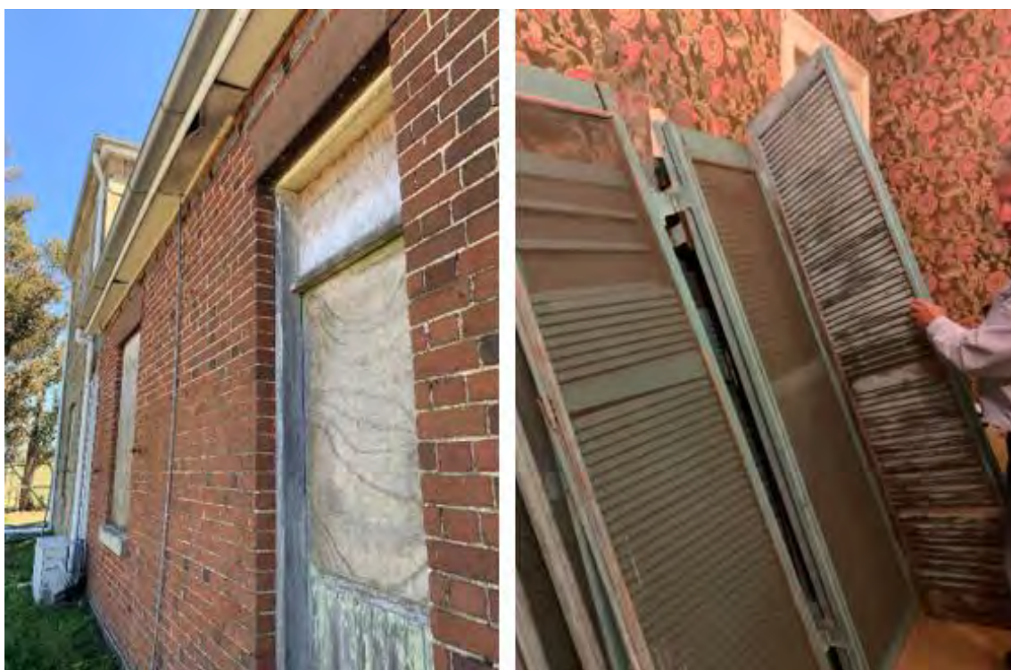
Figure 39. Left: The existing external shutters have been removed, and door and window openings along the southern elevation have been boarded with plywood sheets. Right: The removed external shutters stored inside for repair window.
