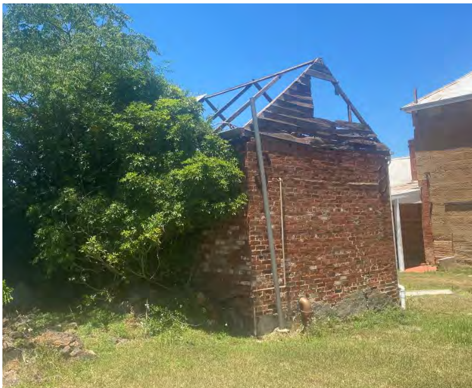
Figure 23. The western elevation of the servants' quarters, showing the damage sustained to the roof as a result of a storm event in December 2020.
