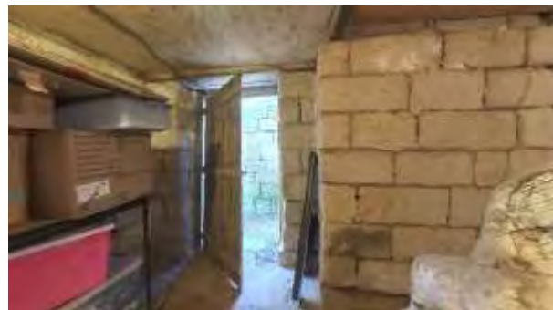
Figure 104. Internal view of the cellar, note the dilapidated timber braced door.
