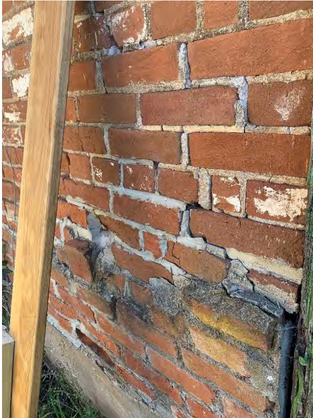
Figure 15. The cracking and bulging of brickwork typical at Negoa, resulting from ground movement. Note the previous cement mortar repairs are failing. Photograph taken September 2020.
