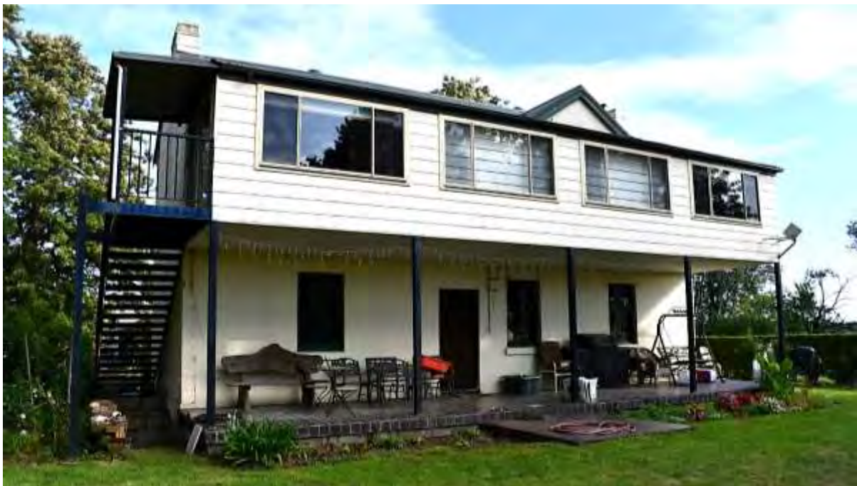
Figure 90. Detailed view of the primary elevation (eastern) of the Rosebrook Homestead. Note the sandstone stair accessing the cellar is positioned to the left, below the contemporary steel stair.
