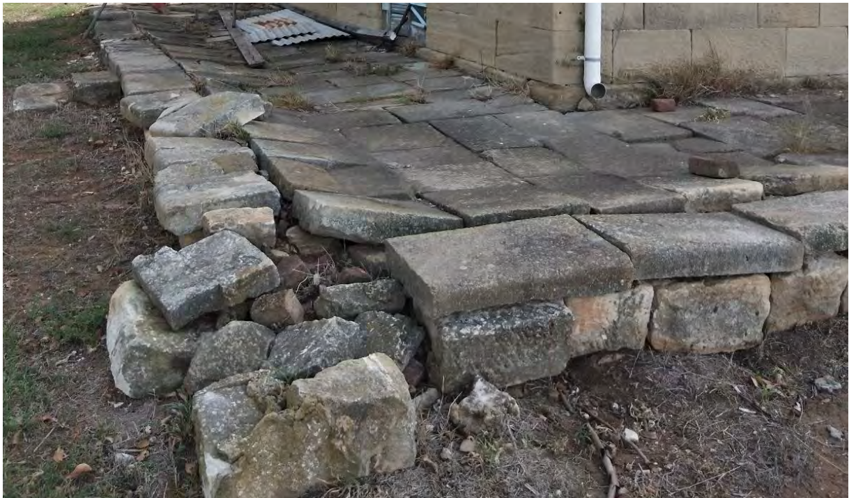
Figure 16. The failed stone paving on west and north elevations of the c.1850s–60s sandstone section of Negoa. Photograph taken April 2018.
