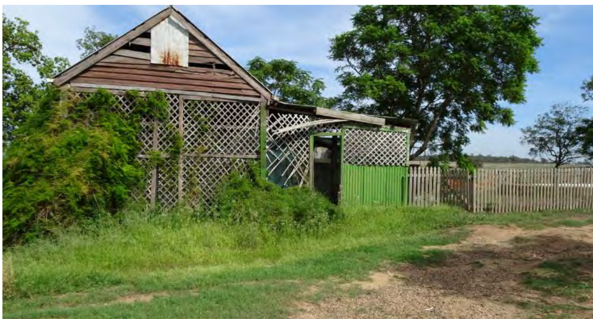
Figure 21. The servants' quarters, showing the extension constructed of timber and corrugated sheet metal. This photograph shows the building as it was in April 2018.
