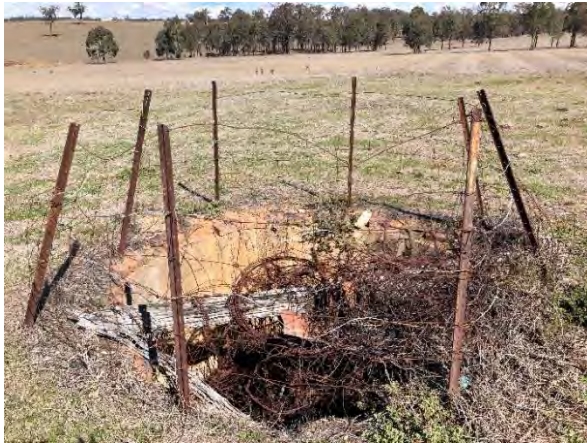
Figure 6. The underground tank at Devine's, constructed of brick and lined with plaster (Source: Extent Heritage 2018).
