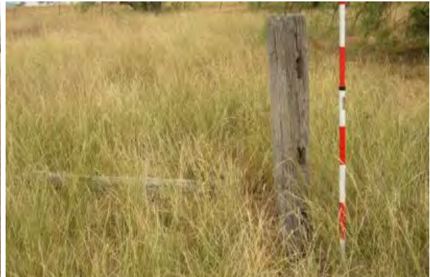
Figure 7. Post mortised for three rails, possible gateway to schoolyard from road (Source: VAHS 2014, p. 257).
