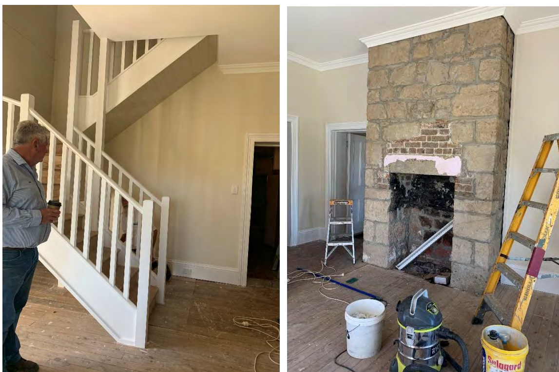
Figure 35. Left: The reconstructed internal stair. Right: The exposed stone chimney breast in ground floor bedroom.
