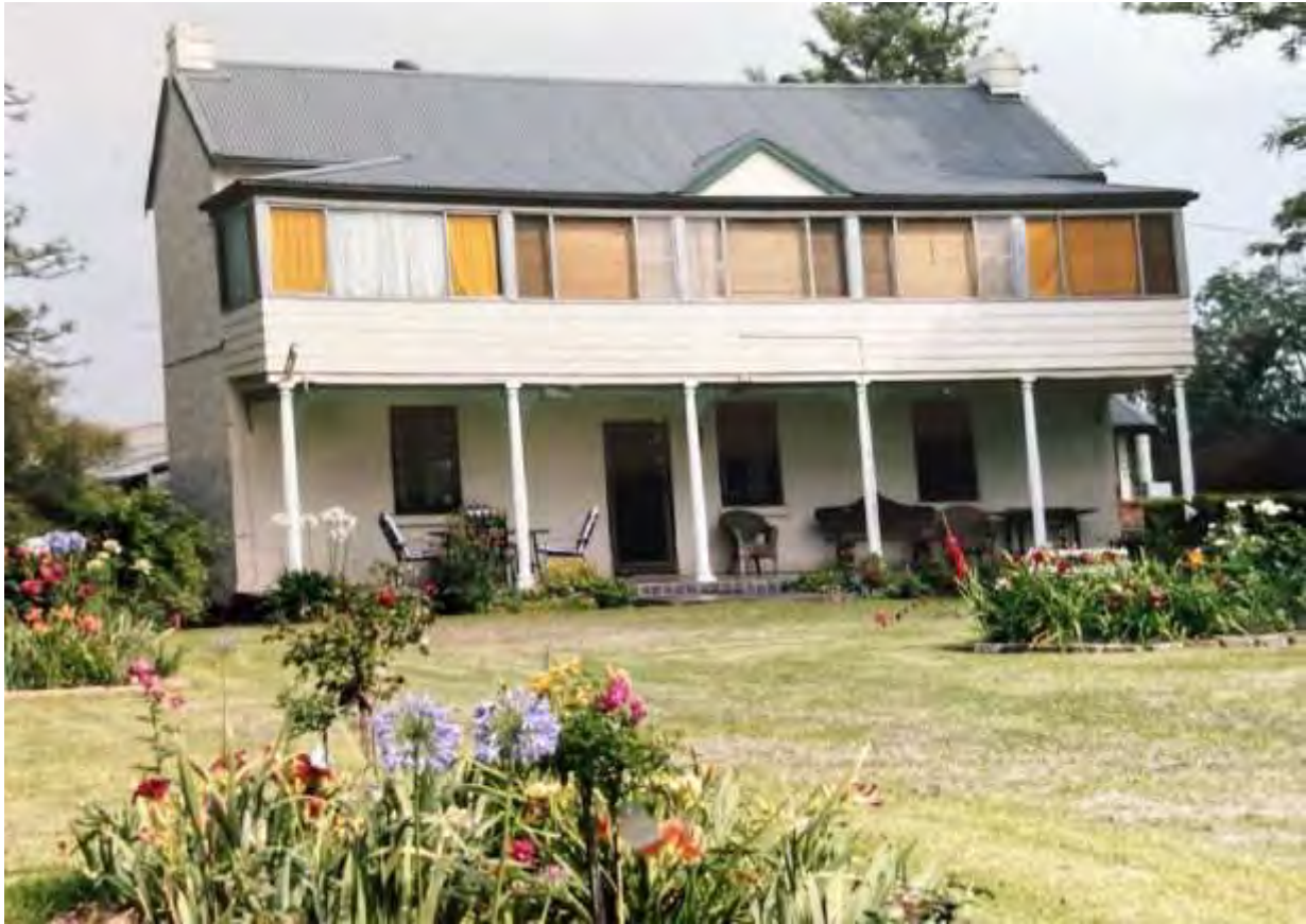
Figure 25. c.2007 photograph of the Rosebrook Homestead noting the roof tiles have been replaced with corrugated galvanised iron sheet. Source: Extent Heritage (2024).
