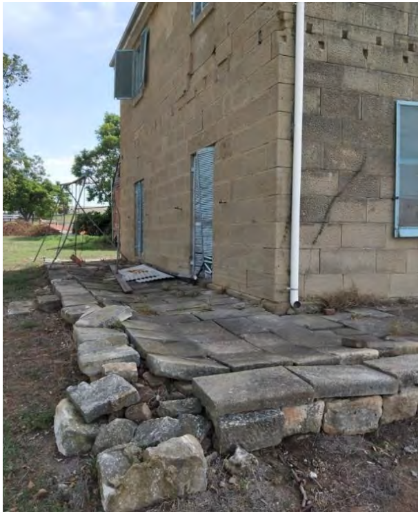
Figure 52. A section of the failing stone paving on western and northern elevations of the sandstone section of Negoa.
