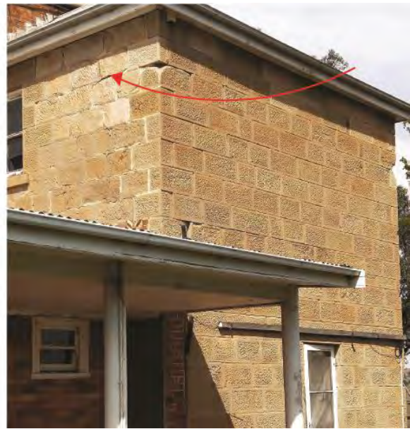
Figure 50. The eastern and northern elevations of Negoa comprising sandstone, showing the cracks in the stonework and the abraded stones (red arrows). The causes must be investigated and repairs undertaken.
