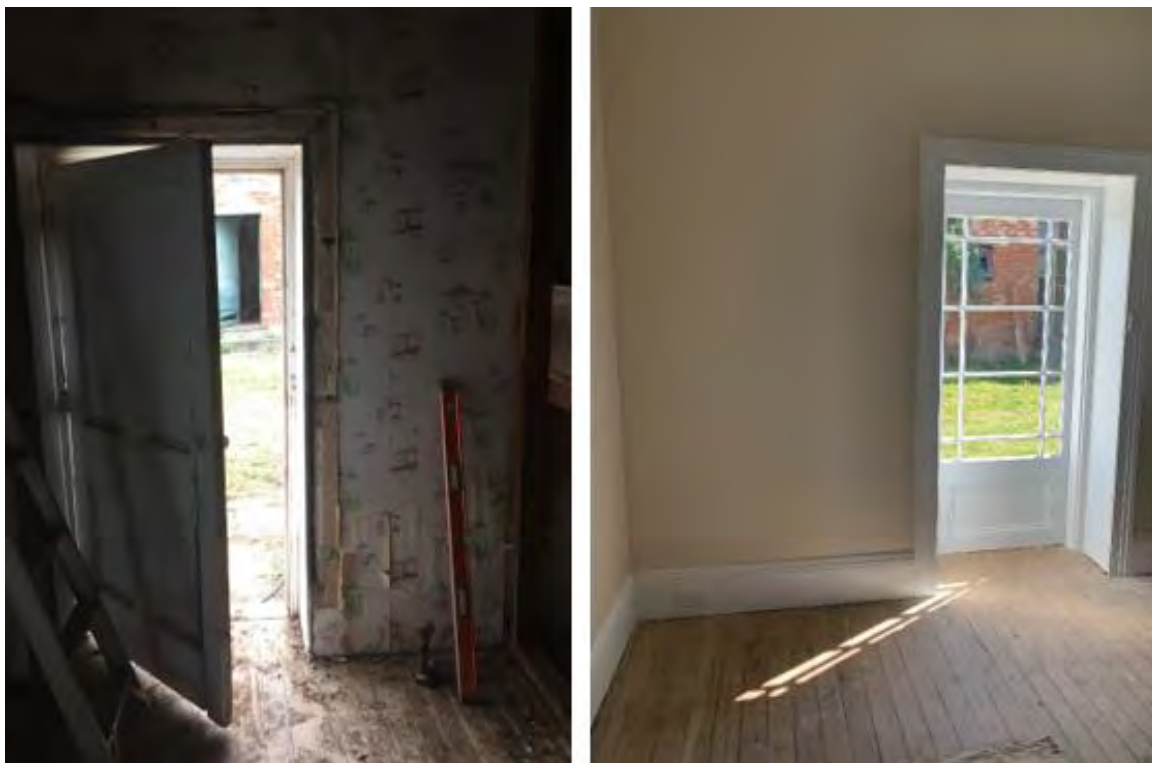
Figure 36. Left: The original four-panel entry door, which has been removed. Right: The replacement half-glazed door with margin glazing.
