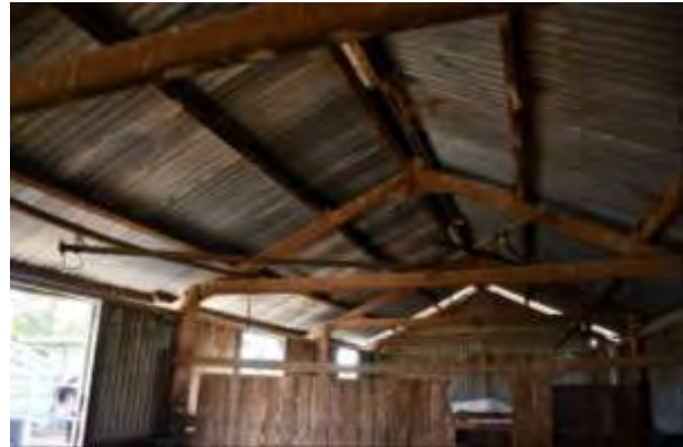
Figure 116. Interior photograph of the open truss timber frame of the stables.
