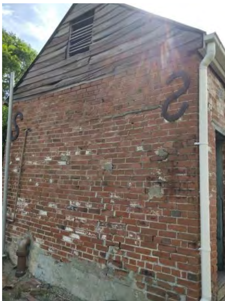
Figure 45. The western elevation of the servants' quarters outbuilding. Note the cement-based repair work. Do not employ this method of repair in future. Where possible without inflicting further structural damage, reverse where it has occurred by raking out joints and repointing with lime mortar.
