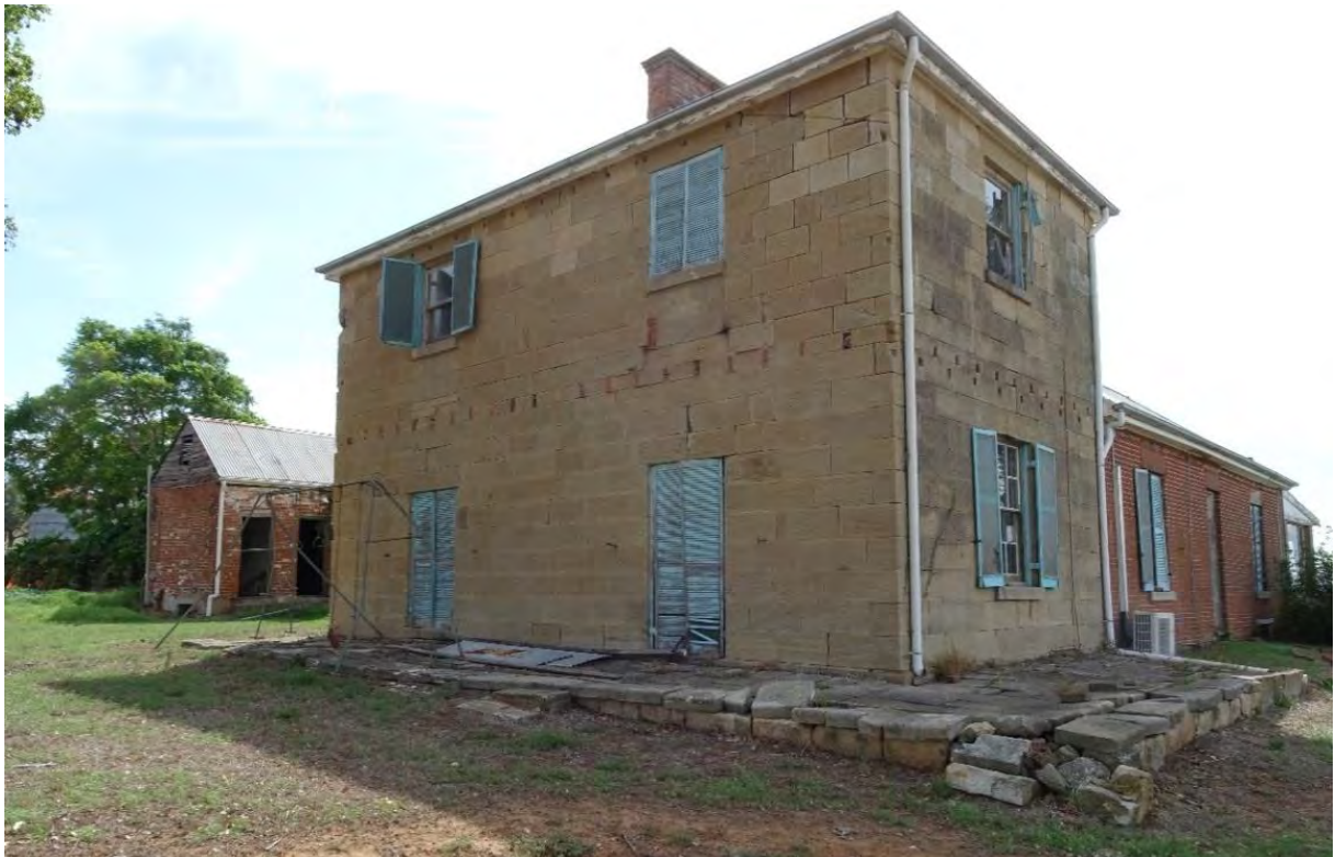
Figure 10. The western elevation of Negoa's sandstone section. Note the holes in the sandstone where the verandah was originally mounted. The servants' quarters are visible to the left and the c.1845 brick section of the homestead is visible to the right along the southern elevation. Photograph taken April 2018.
