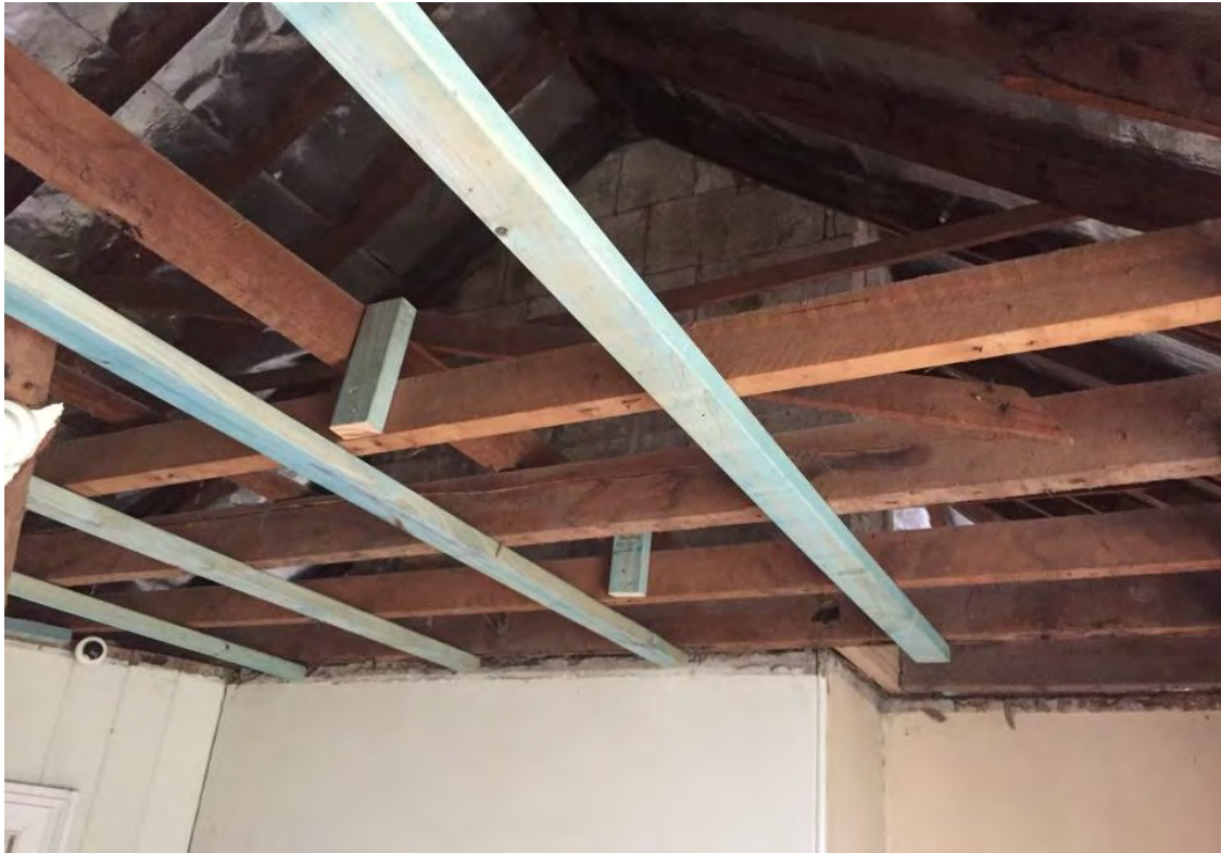
Figure 32. Image illustrating the ceiling space in one of the upstairs rooms showing the augmentation of the roof structure following the removal of the dilapidated ceiling fabric.
