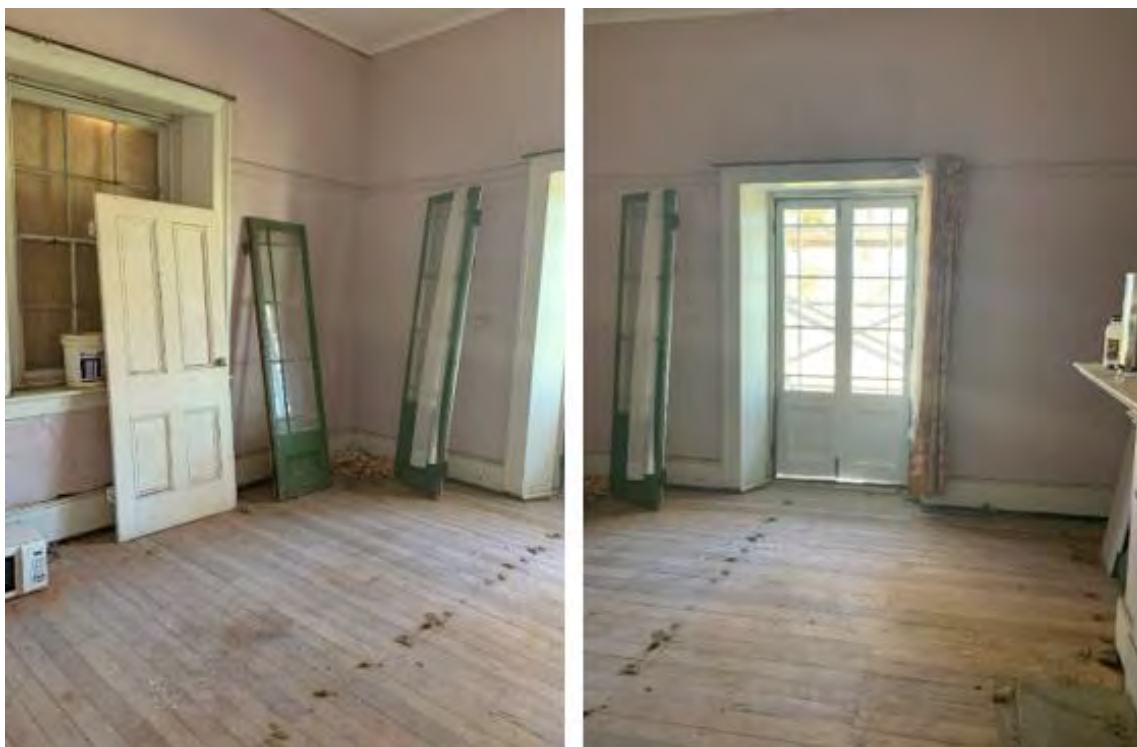
Figure 37. Left: The removal of the existing French doors. Right: The reinstatement of new doors reconstructed to the original profile.
