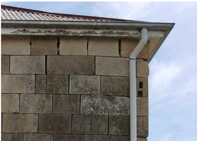
Figure 51. Southern elevation of the sandstone section of Negoa, showing damage to the upper courses of stonework caused by building movement. The causes are to be investigated and the stones reset.
