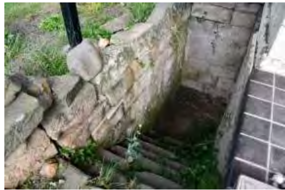
Figure 102. Detail view of the sandstone retaining walls and stair providing access to the underground cellar.
