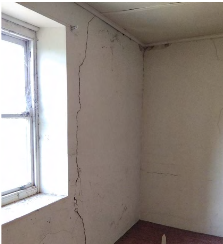
Figure 29. Interior view of one of Negoa's rooms, showing possible structural cracking typical in the internal walls of the c.1850s–60s sandstone section. Photograph taken April 2018.
