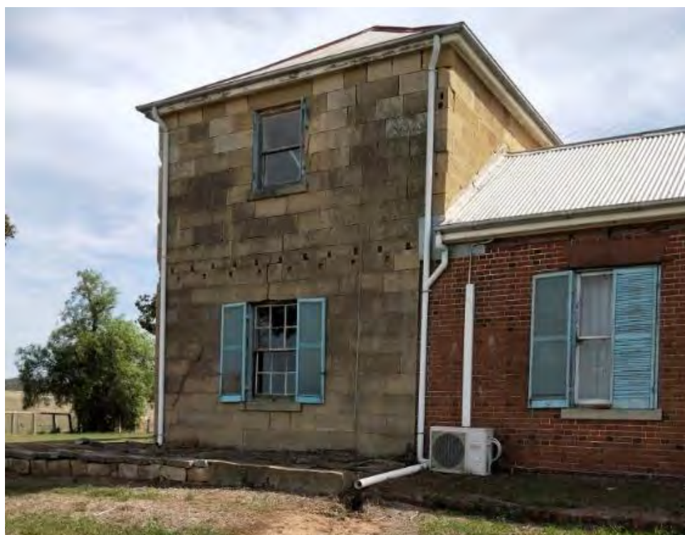
Figure 47. The white downpipes and air conditioning materials detract from the aesthetic appearance of the southern elevation. The air conditioners should be removed and the downpipes replaced with galvanised ones.
