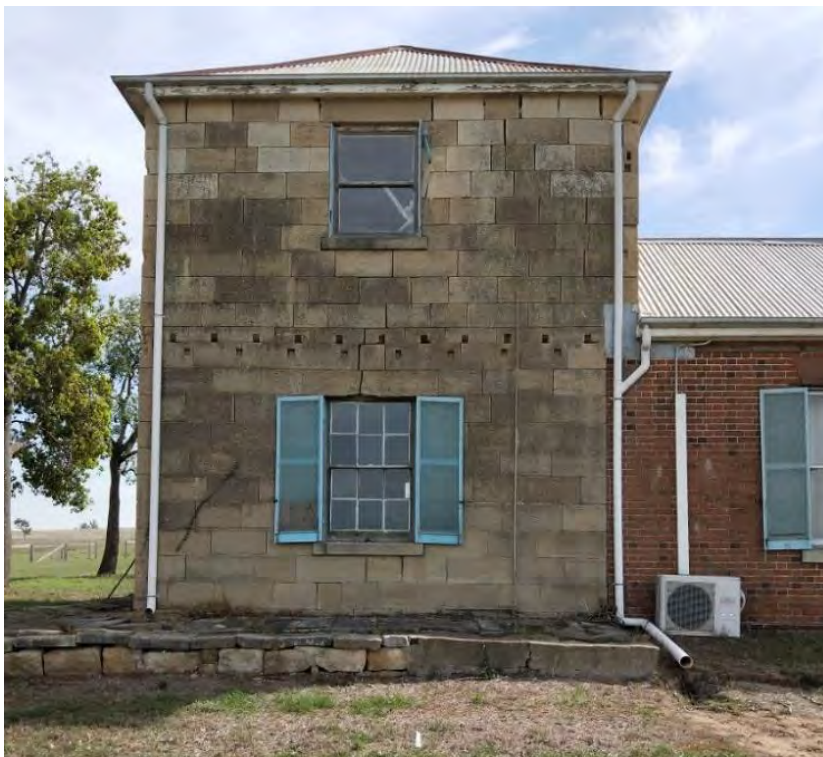
Figure 12. The southern elevation of the c.1850s–60s sandstone section of Negoa, showing the original lower floor window and the non-original upper floor window. It is noted that there is currently no access from the upstairs rooms to the location of the former verandah on this southern elevation. Photograph taken April 2018.
