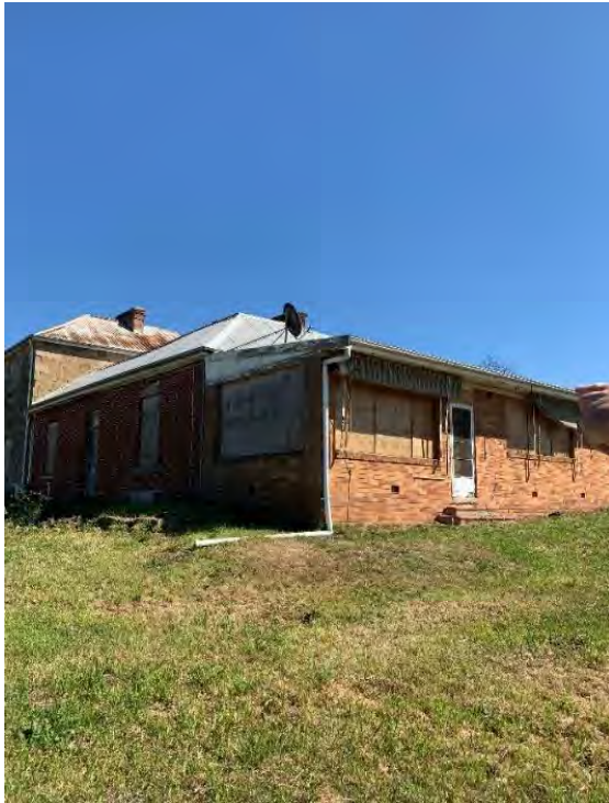
Figure 30. The downpipes have been extended to carry water away from the walls, footings and stone paving around the homestead's structures
