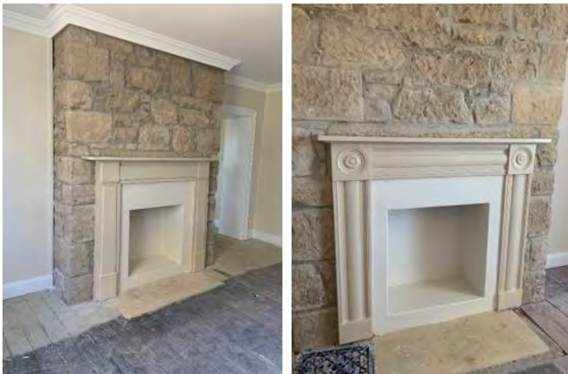
Figure 40. The exposed repointed stone chimney breast and reinstated fireplace and mantelpieces in the upstairs bedrooms.
