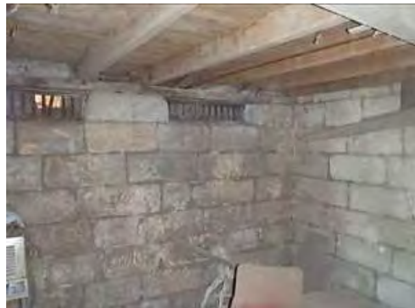
Figure 30. Cellar area with ventilation openings fitted with steel rods and the timber framing to the ground level above. Source: VAHS (2014, 466).
