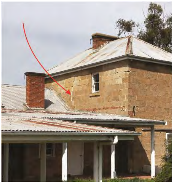
Figure 50. The eastern and northern elevations of Negoa comprising sandstone, showing the cracks in the stonework and the abraded stones (red arrows). The causes must be investigated and repairs undertaken.
