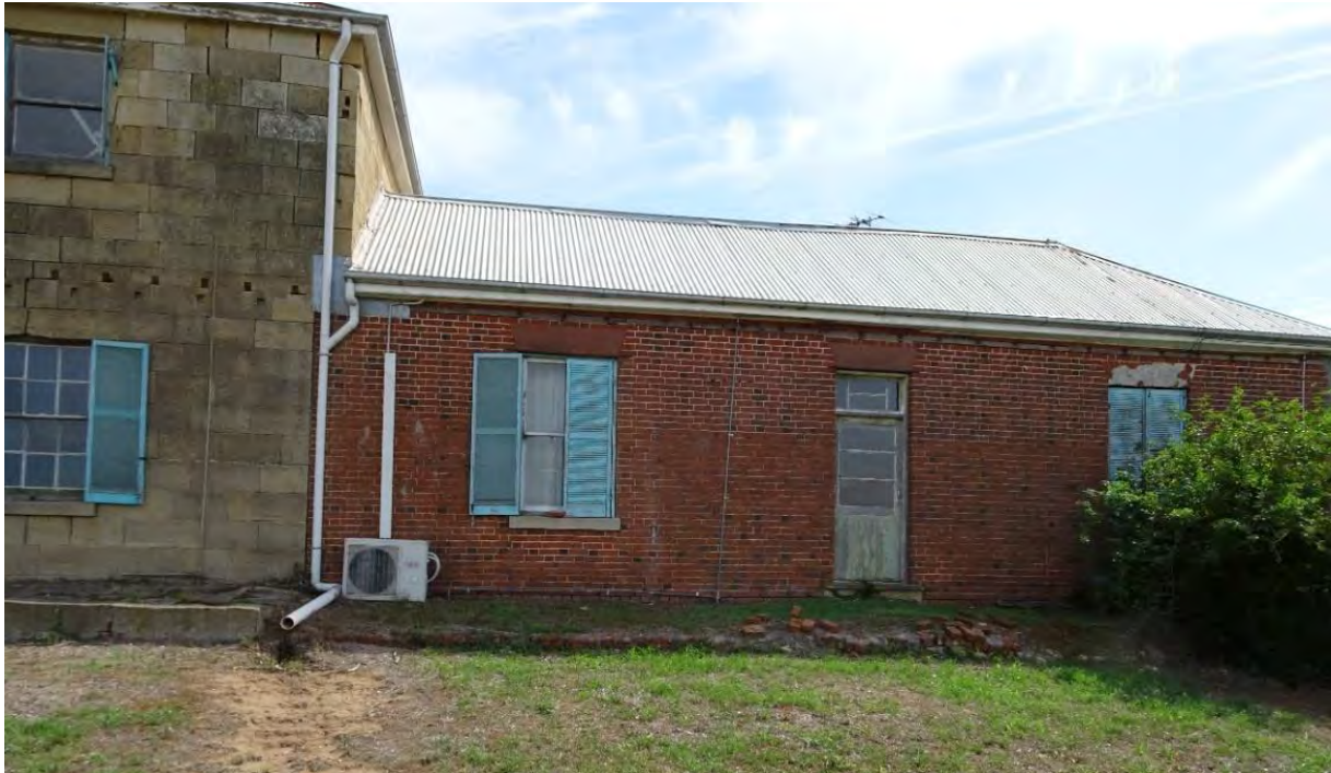
Figure 11. The southern elevation of the c.1845 brick section of Negoa. Note the Flemish bond brickwork of this original c.1845 section. Photograph taken April 2018.
