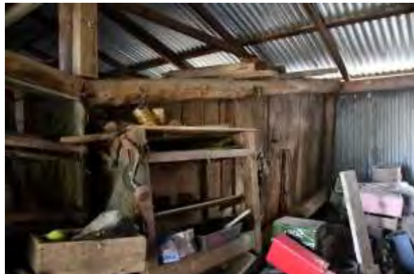
Figure 108. Interior view of the timber-framed shed, note the remnant bush timber elements.
