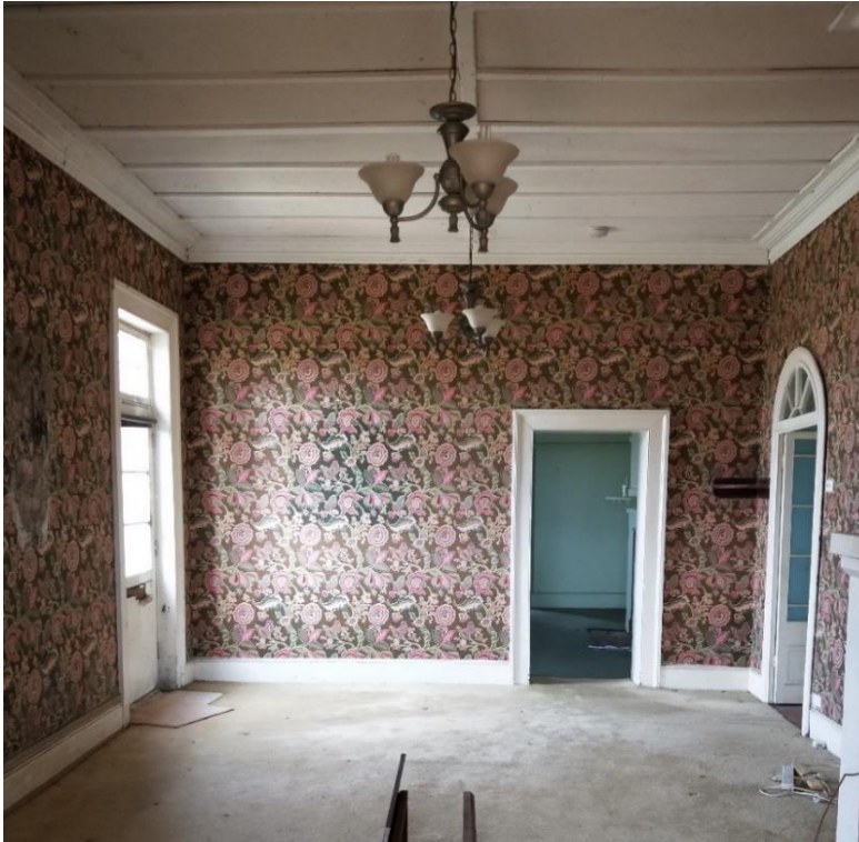
Figure 27. Interior view of the c.1845 section of the homestead. Note the timber-panelled ceiling and contemporary wallpaper. Photograph taken April 2018.
