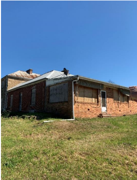
Figure 30. The downpipes have been extended to carry water away from the walls, footings and stone paving around the homestead's structures
