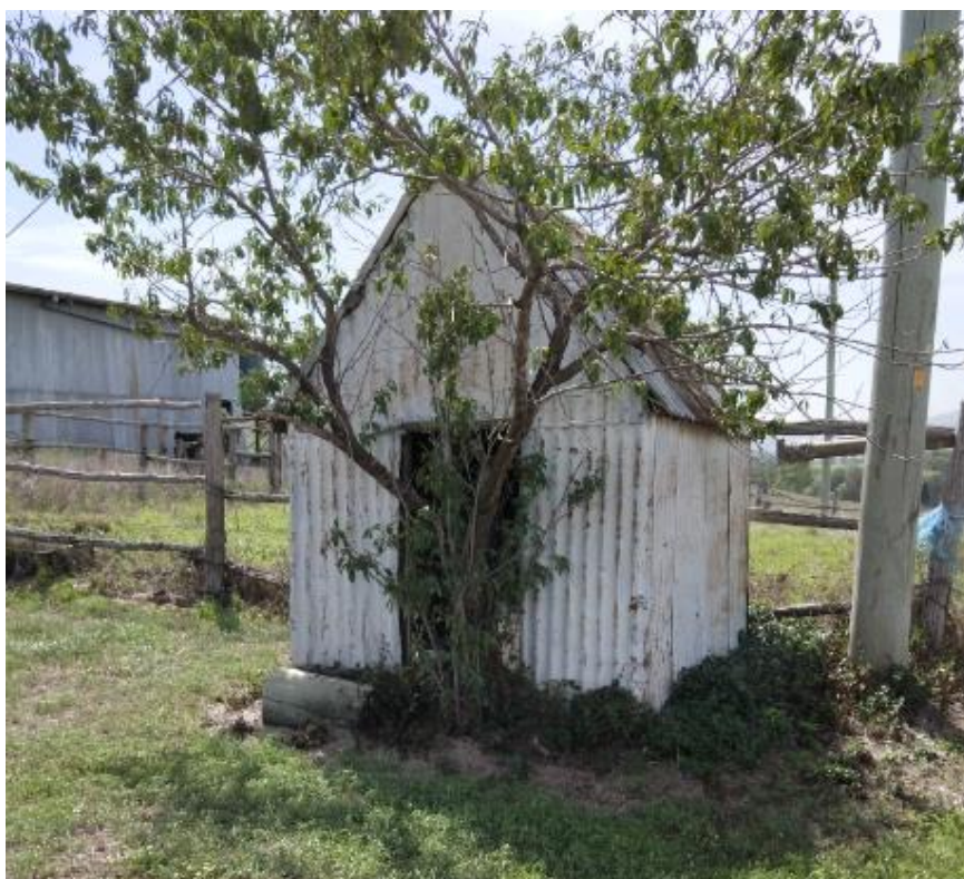
Figure 25. The smaller shed, of corrugated metal sheeting construction, located to the north of the larger weatherboard shed. Photograph taken April 2018.
