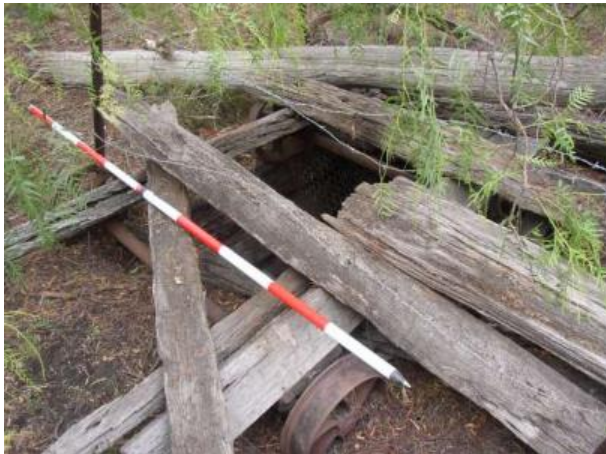
Figure 6. View of open mine shaft partially covered over with timbers and a piece of machinery (shaft with wheels) (Source: VAHS 2014, p. 241).
