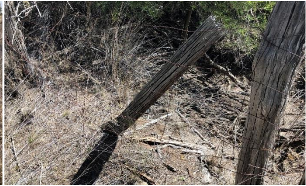
Figure 5. Timber posts near mine shaft at MP20 (Source: Extent Heritage 2020, p. 56).
