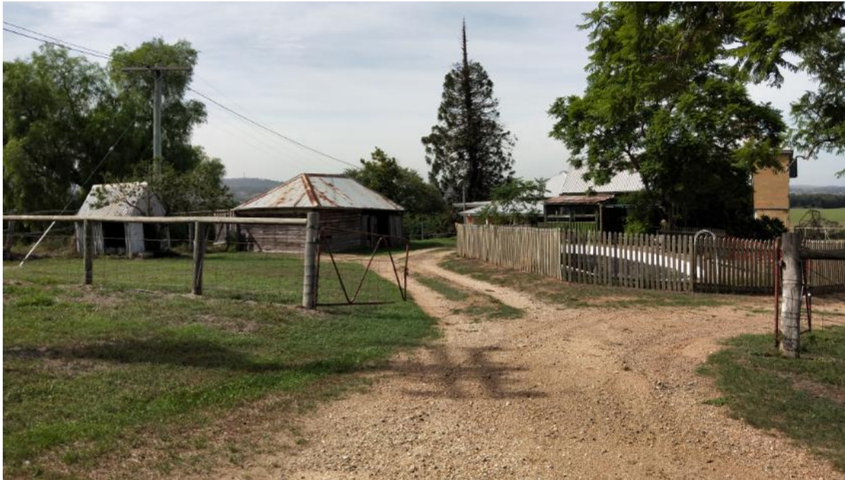
Figure 26. View looking towards Negoa showing the relationship between the three outbuildings: the smaller shed is visible to the far left, adjacent to the larger weatherboard shed (centre) and behind the timber paling fence to the right is the servants' quarters. Photograph taken April 2018.
