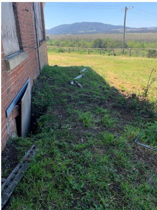
Figure 48. The remnant original brick paving visible on the homestead's southern elevation.
