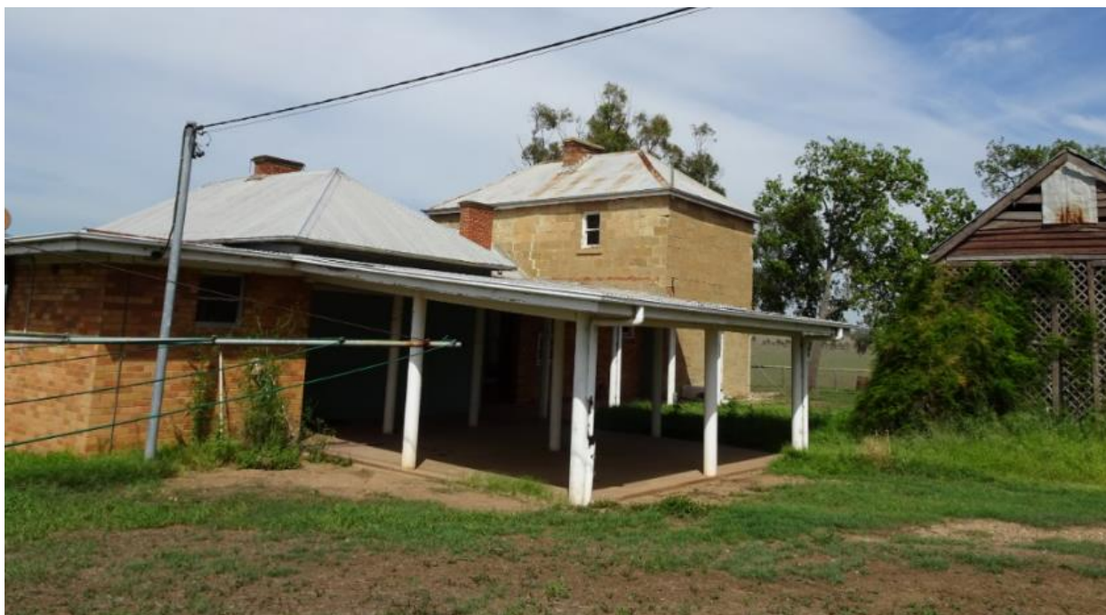
Figure 17. The c.1950s addition to the brick homestead, comprising a single-storey structure with a corrugated metal skillion roof. The 1850s–60s sandstone extension is evidence in the background, and the servants' quarters is visible to the right. Photograph taken April 2018.
