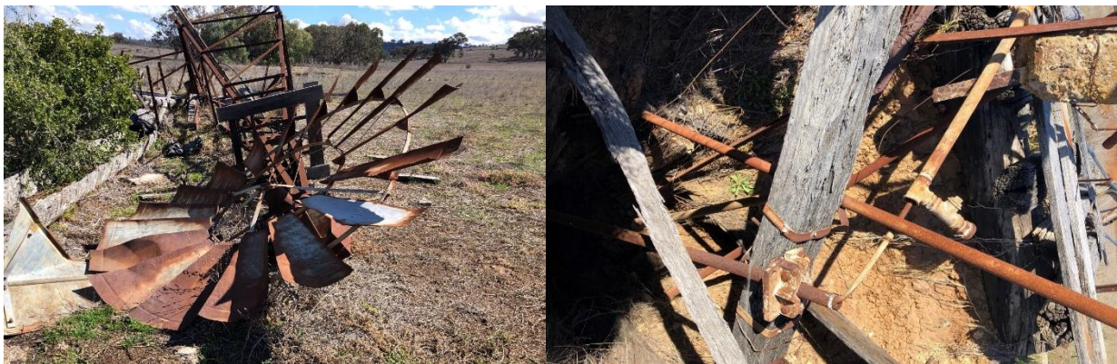
Figure 10. The collapsed windmill and the remains of Figure 11. The well under the windmill at MP25, which is the wooden trough at MP25 (Source: Extent Heritage 2020, p. 80) filled with debris and soil deposits (Source: Extent Heritage 2020, p. 56).
