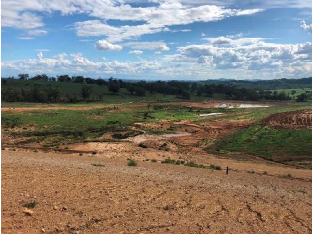
Rehabilitation Photo 5 - Seeding is required in area above ED2 which is showing signs of erosion
