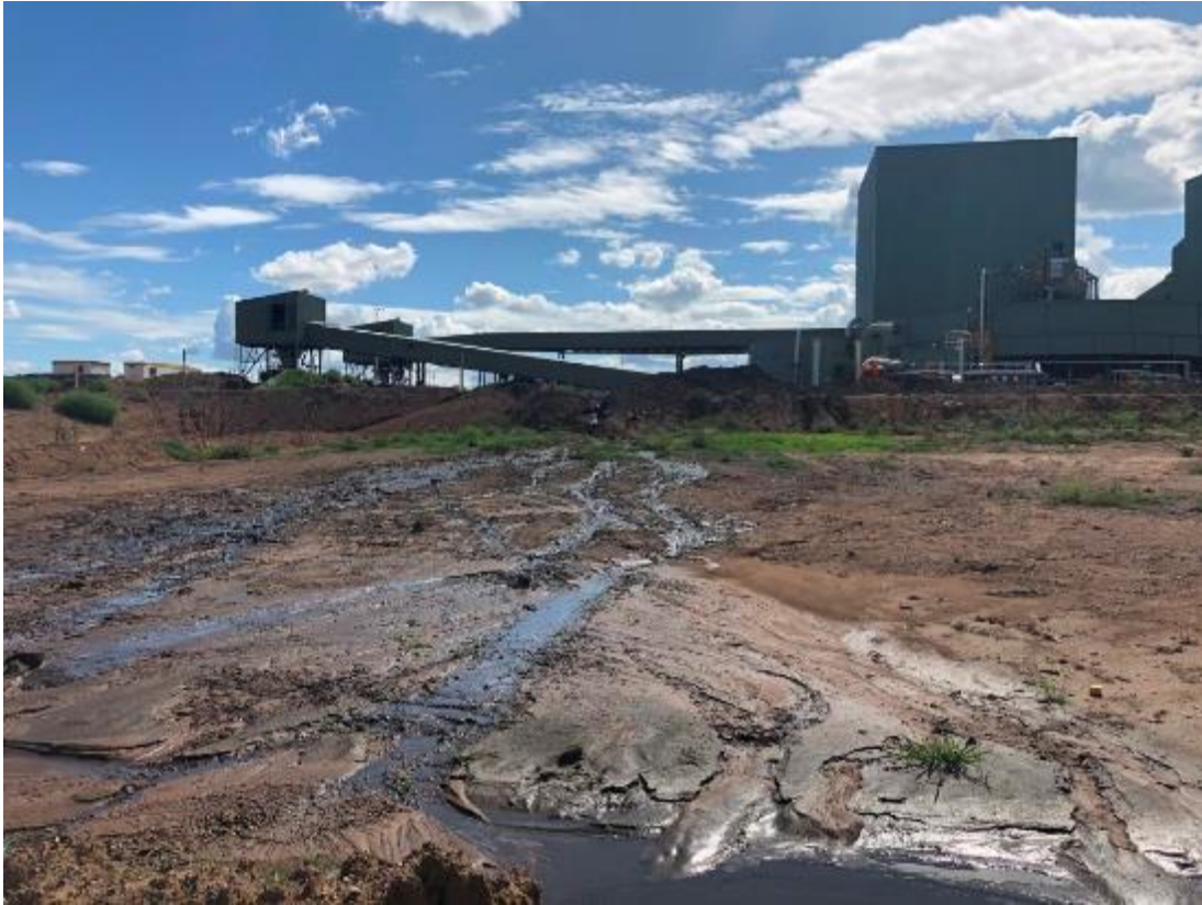
Erosion Photo 9 - Erosion and sediment at the CHPP area
