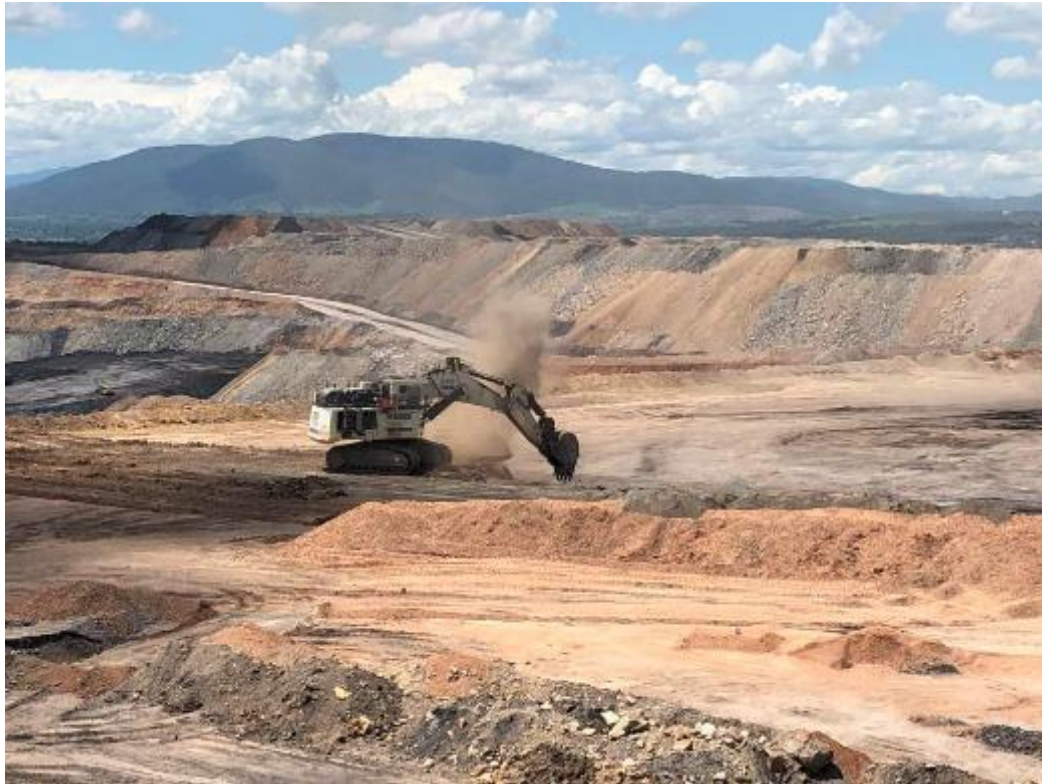
Photo Air 3 -Dust generation from excavator staying within the pit floor
