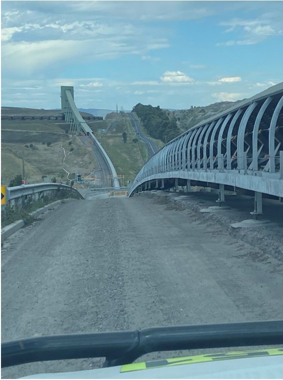
Photograph F.70 Coal conveyor
