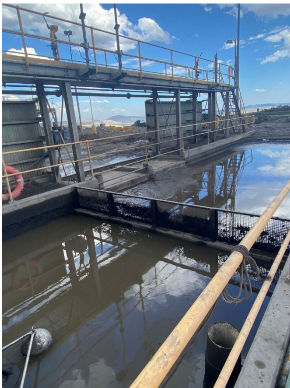
Photograph F.104 Oily water separator
