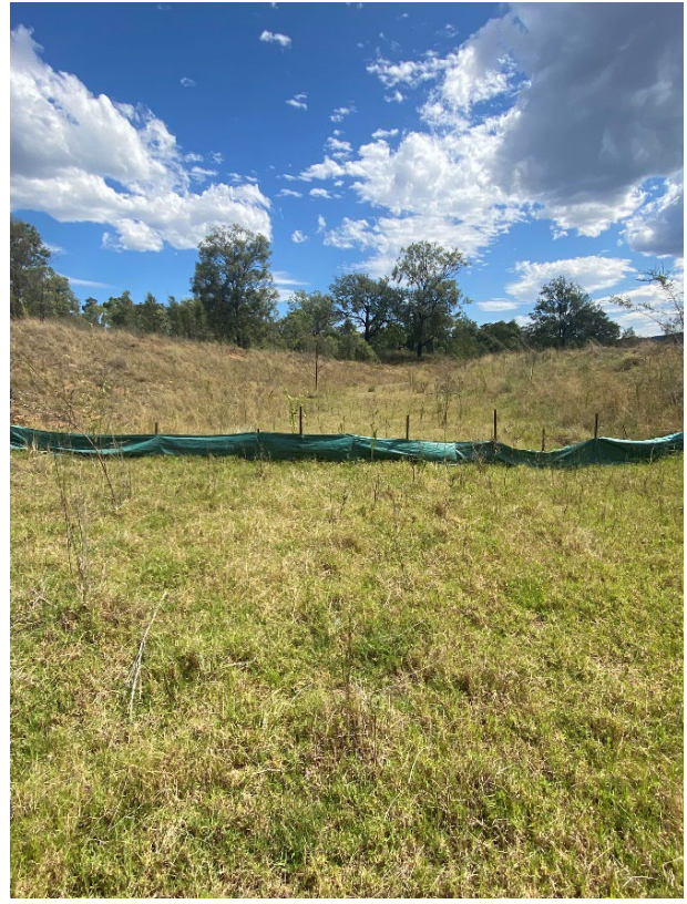
Photograph F.52 Erosion fencing
