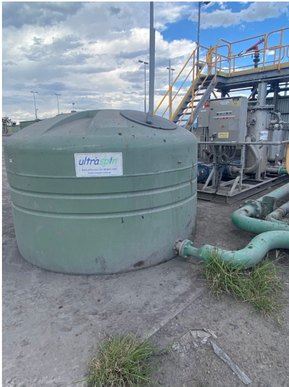
Photograph F.102 Oily water separator
