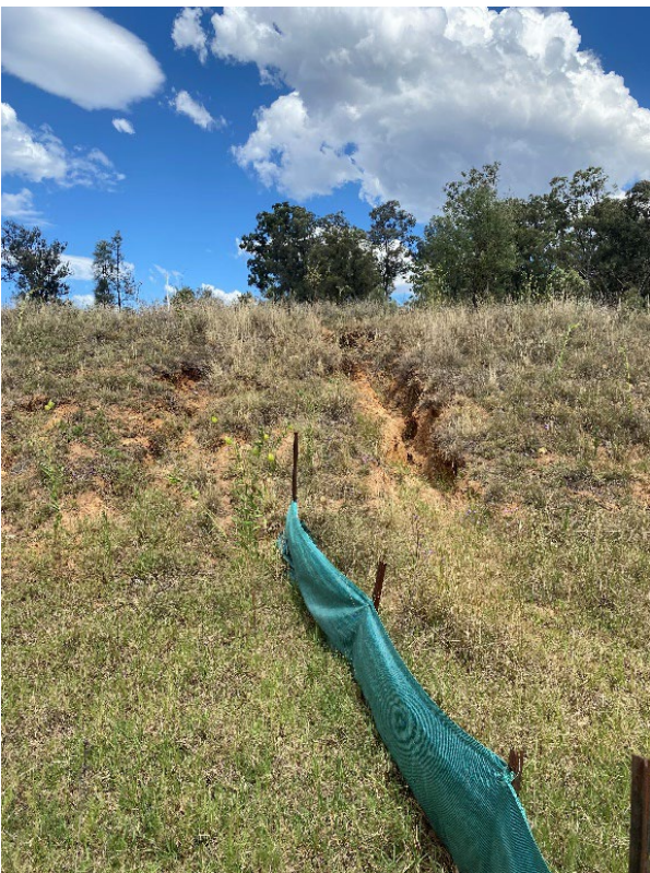
Photograph F.46 Erosion fencing
