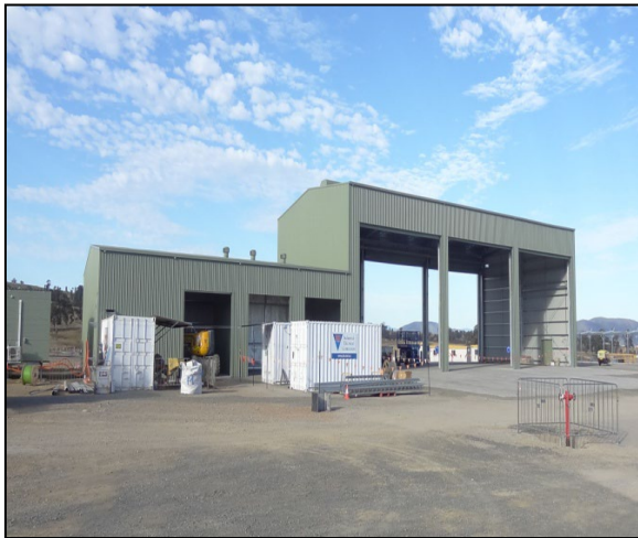
Plate 5: Workshop within the Mine Infrastructure Area.
