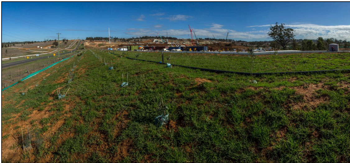
Plate 7: Visual bunding/screen planting along Wybong Road.
