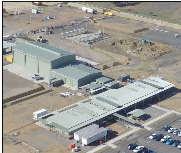
Plate 6: Workshop and associated buildings within the Mine Infrastructure Area.
