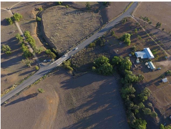
Plate 5: Sandy Creek (SC) – Aerial View (Bio-Analysis , 2020)
