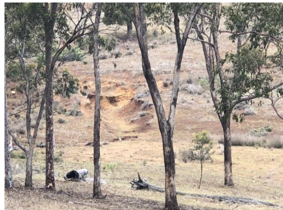
Plate 12: Unnamed Drainage Line (UD2) (Bio-Analysis , 2020)
