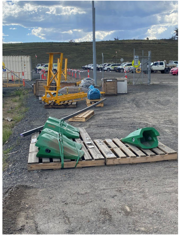
Photograph F.115 Laydown area
