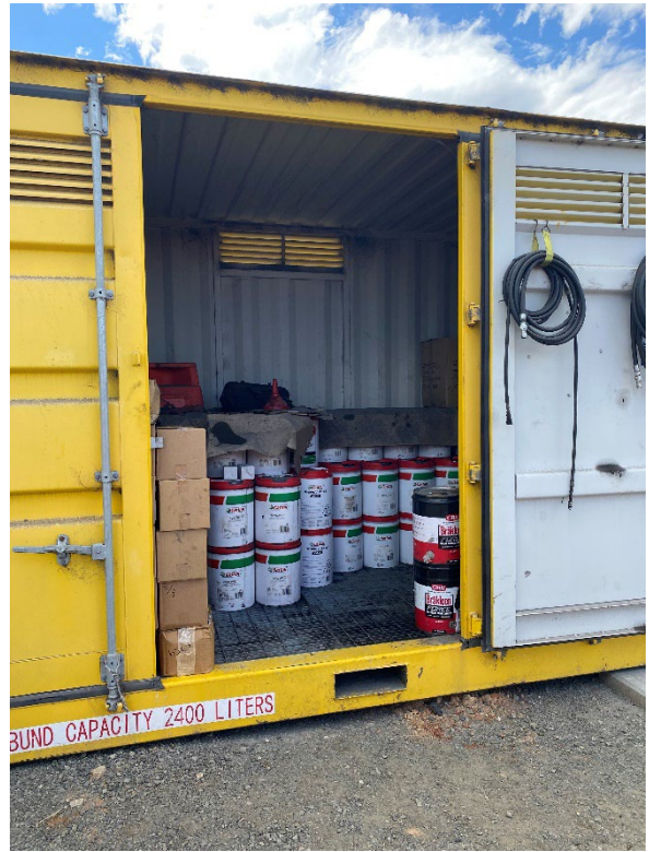
Photograph F.59 Hydraulic oil storage
