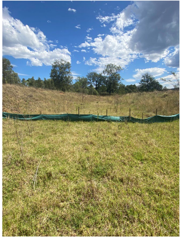
Photograph F.52 Erosion fencing
