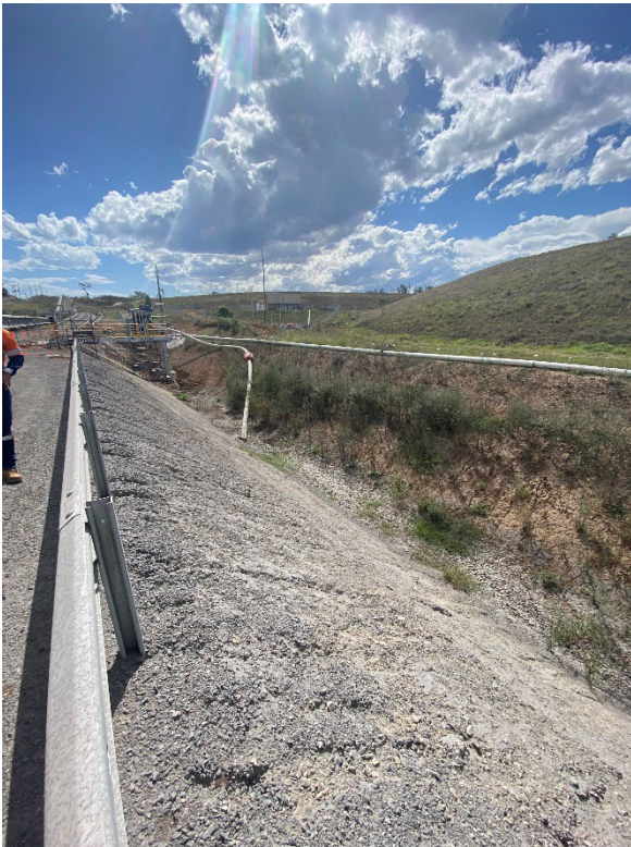
Photograph F.74 Sediment dam (CHPP area)
