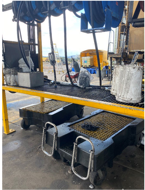
Photograph F.91 Mine infrastructure area
