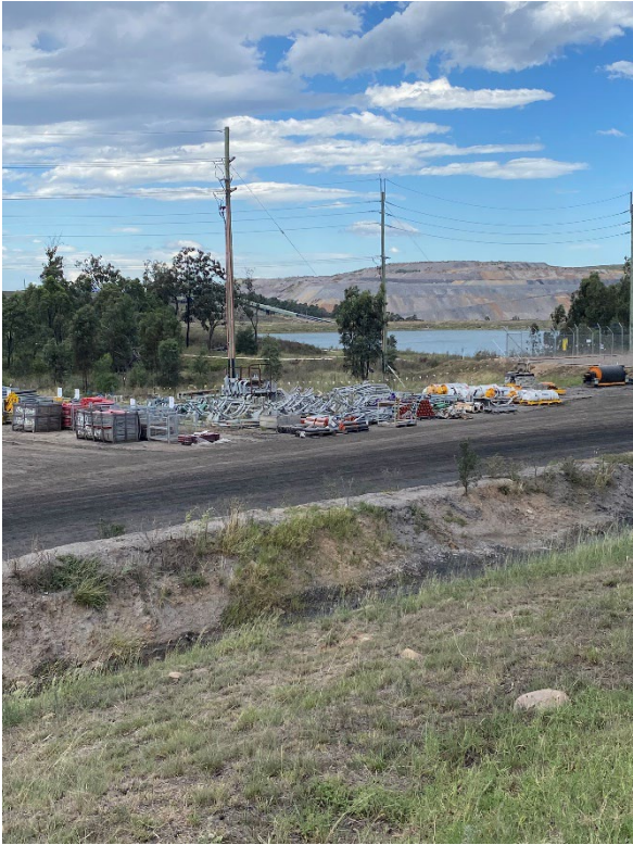
Photograph F.66 Laydown area
