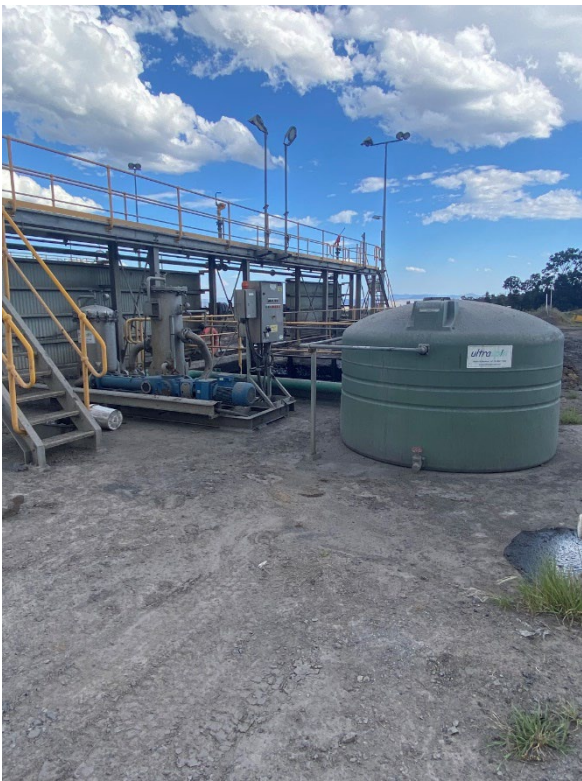
Photograph F.100 Mine infrastructure area
