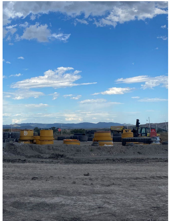
Photograph F.109 Laydown area
