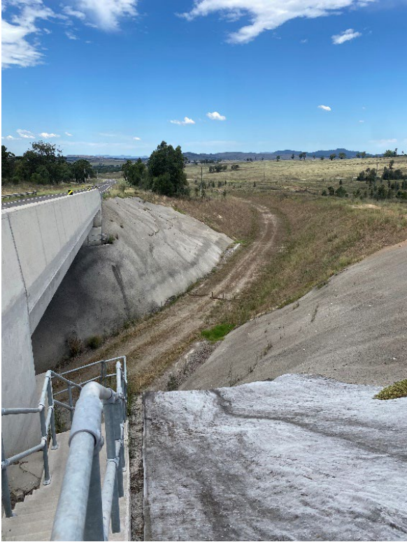
Photograph F.37 Stage 1 rail corridor
