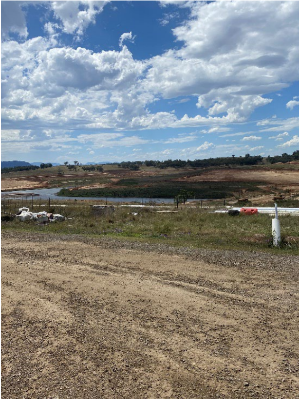
Photograph F.40 Fines emplacement area
