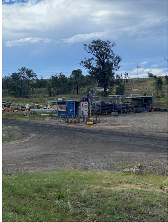
Photograph F.67 Laydown area
