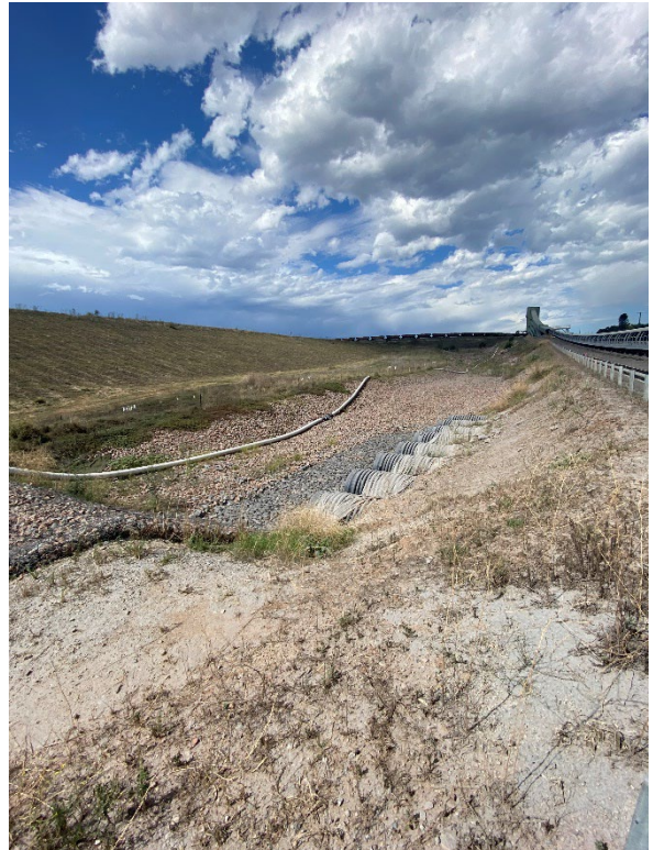
Photograph F.73 Sediment dam (CHPP area)
