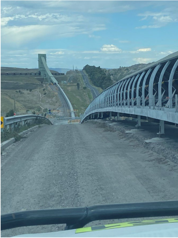
Photograph F.70 Coal conveyor
