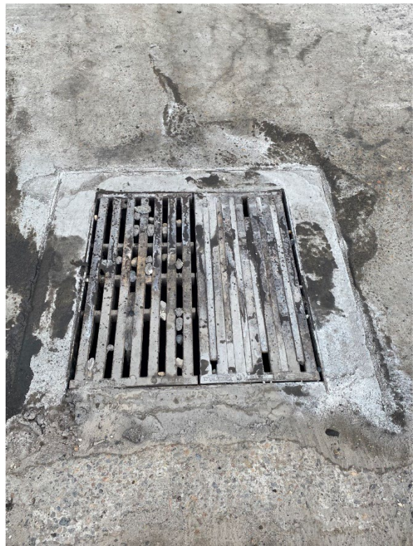
Photograph F.99 Mine infrastructure area
