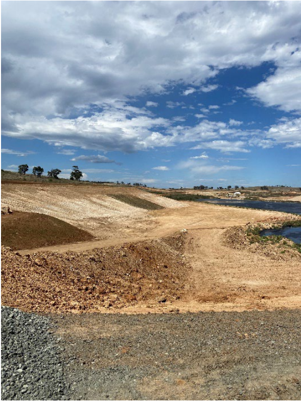
Photograph F.44 Fines emplacement area
