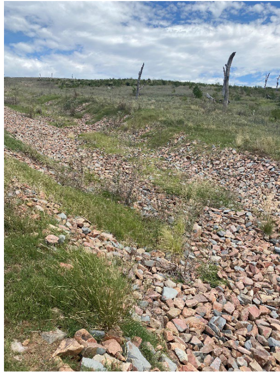
Photograph F.31 Surface water drainage on eastern out of pit emplacement area
