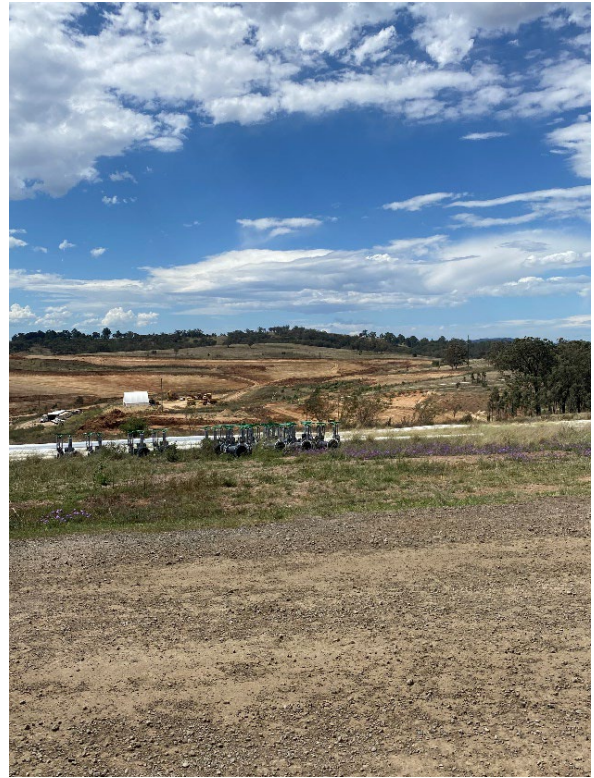
Photograph F.41 Fines emplacement area
