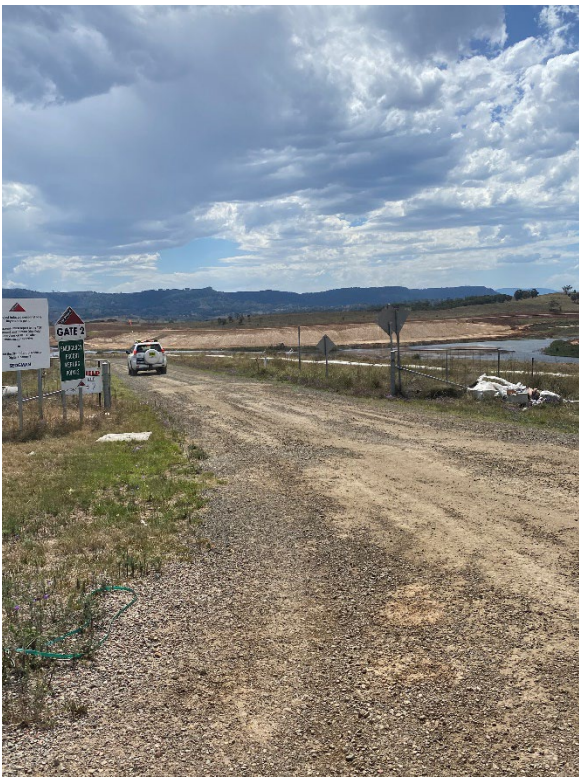
Photograph F.42 Fines emplacement area
