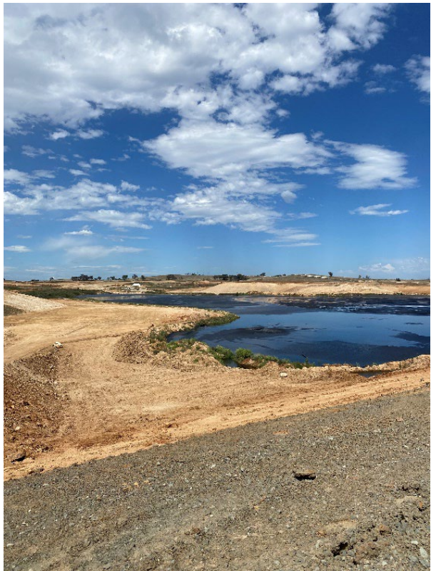
Photograph F.47 Fines emplacement area
