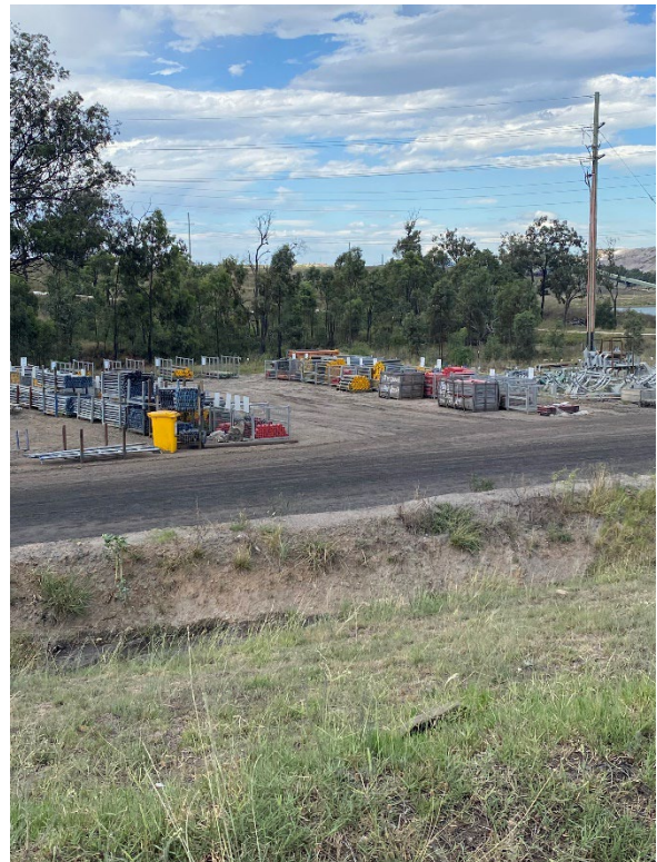
Photograph F.65 Laydown area
