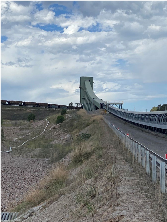
Photograph F.72 Coal conveyor
