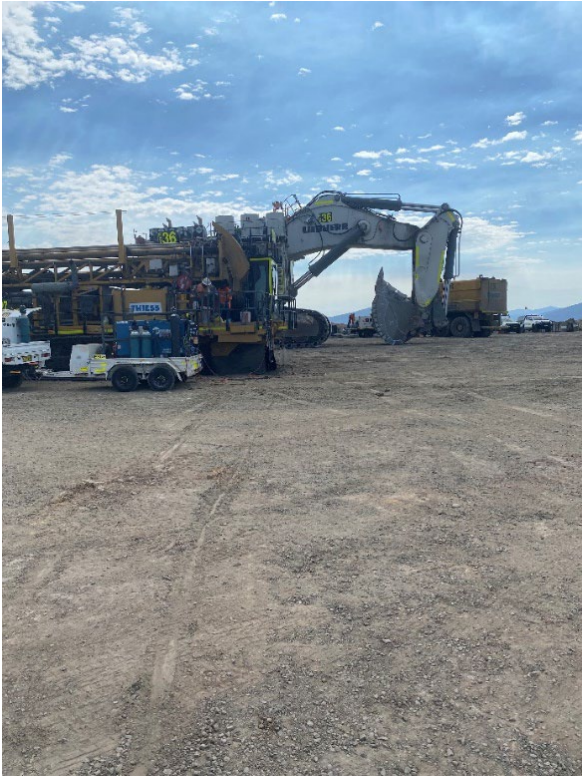
Photograph F.16 Laydown area
