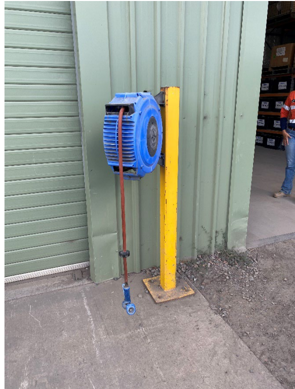
Photograph F.83 Mine infrastructure area
