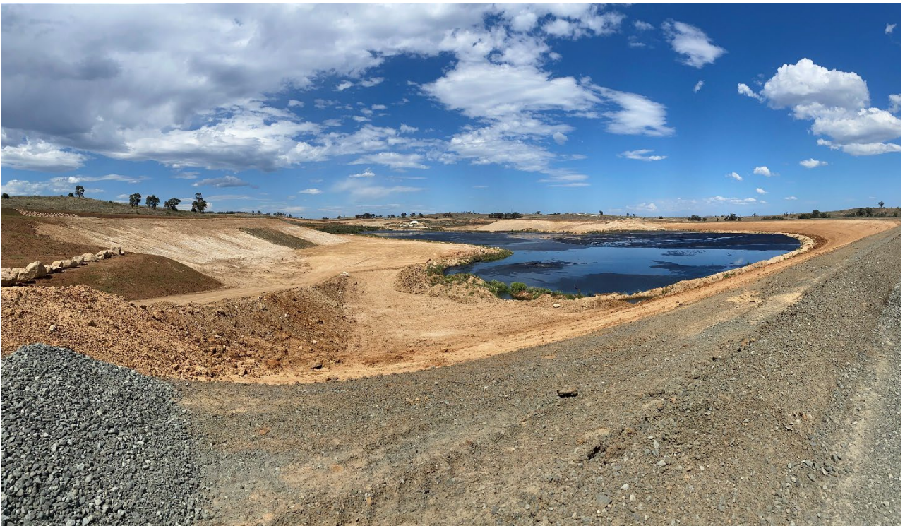
Photograph F.50 Fines emplacement area
