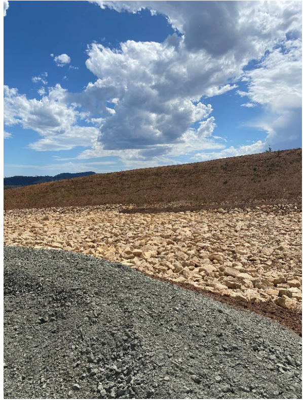
Photograph F.45 Fines emplacement area
