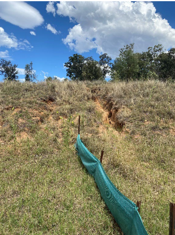
Photograph F.46 Erosion fencing
