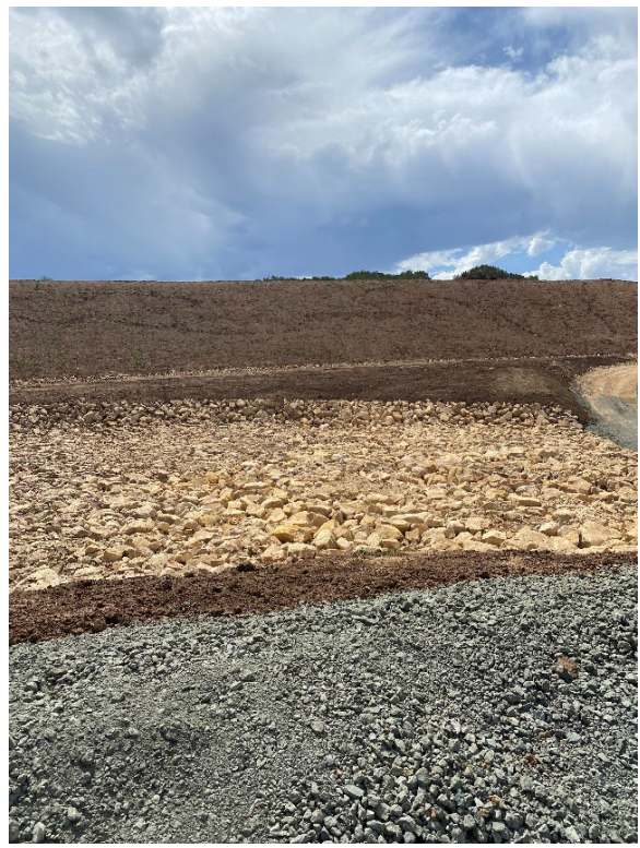
Photograph F.43 Fines emplacement area
