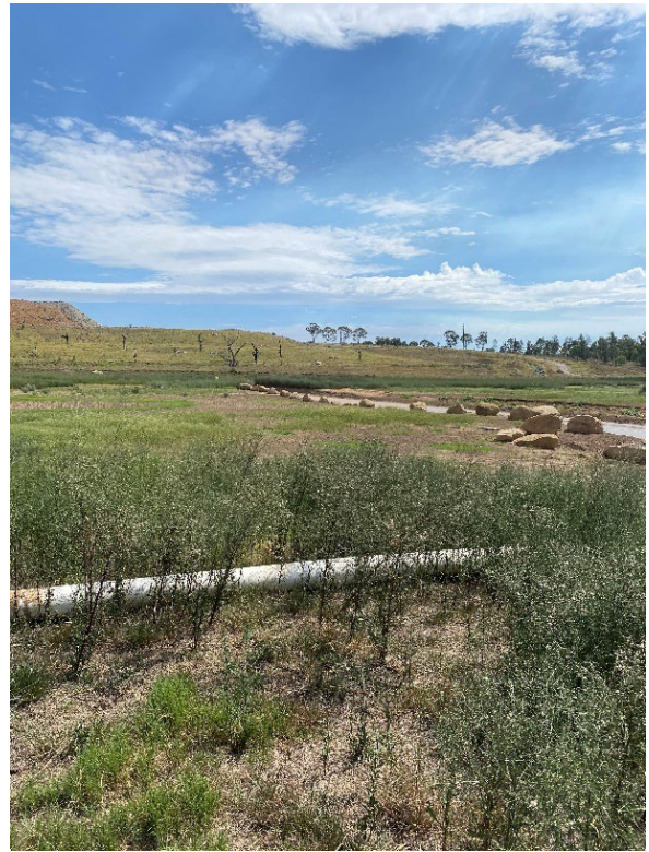
Photograph F.24 New rehabilitation behind ED2
