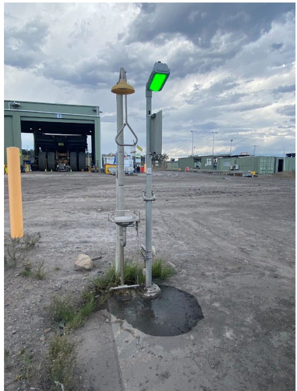
Photograph F.101 Mine infrastructure area
