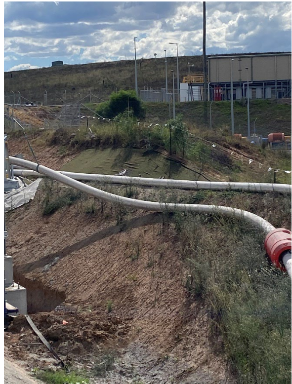
Photograph F.75 Sediment dam (CHPP area)
