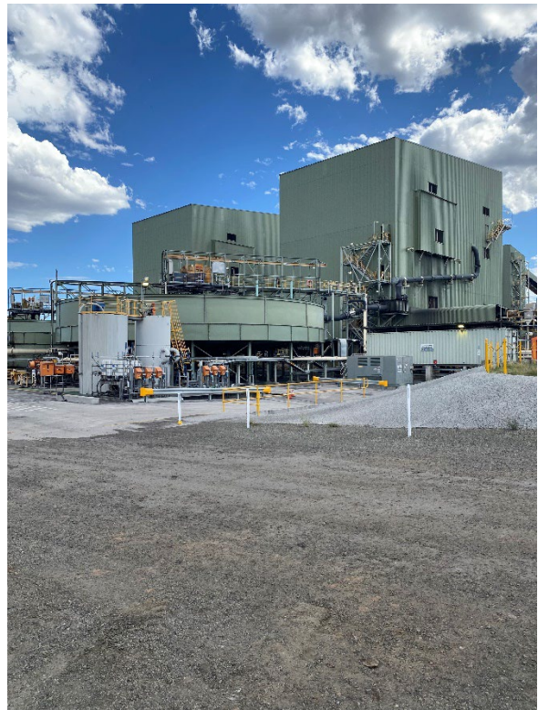
Photograph F.69 CHPP
