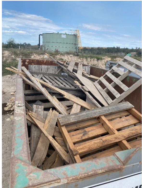
Photograph F.13 Timber recycling
