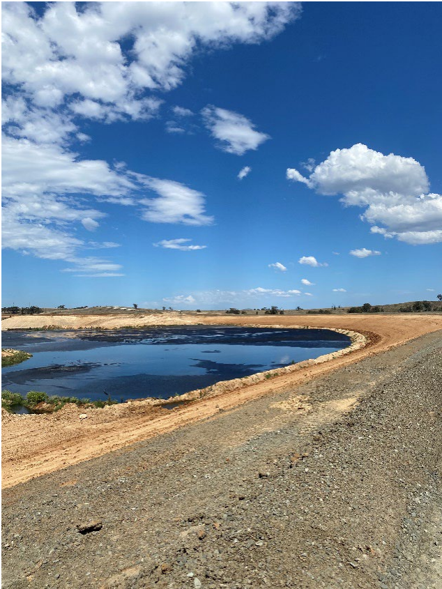
Photograph F.48 Fines emplacement area
