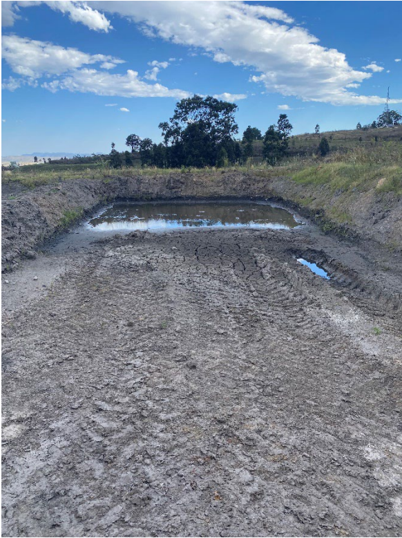
Photograph F.106 Mine infrastructure area
