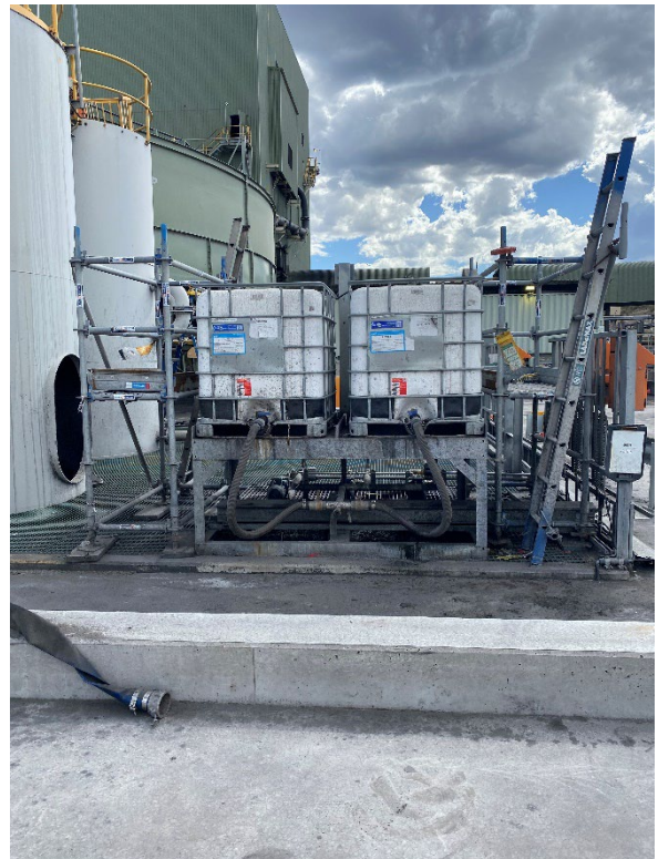
Photograph F.61 CHPP area
