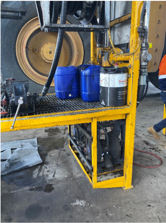
Photograph F.90 Mine infrastructure area
