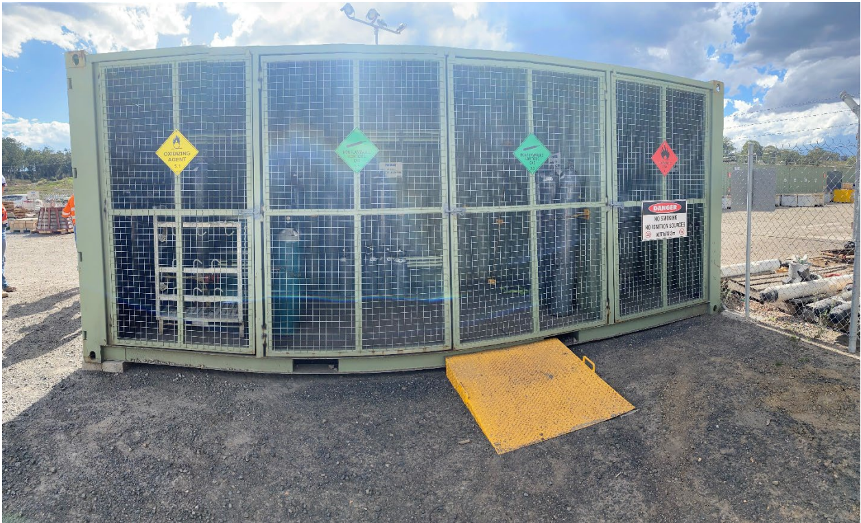
Photograph F.118 Gas storage
