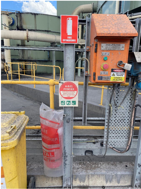
Photograph F.54 Safety signage
