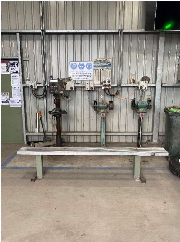
Photograph F.78 Mine infrastructure area
