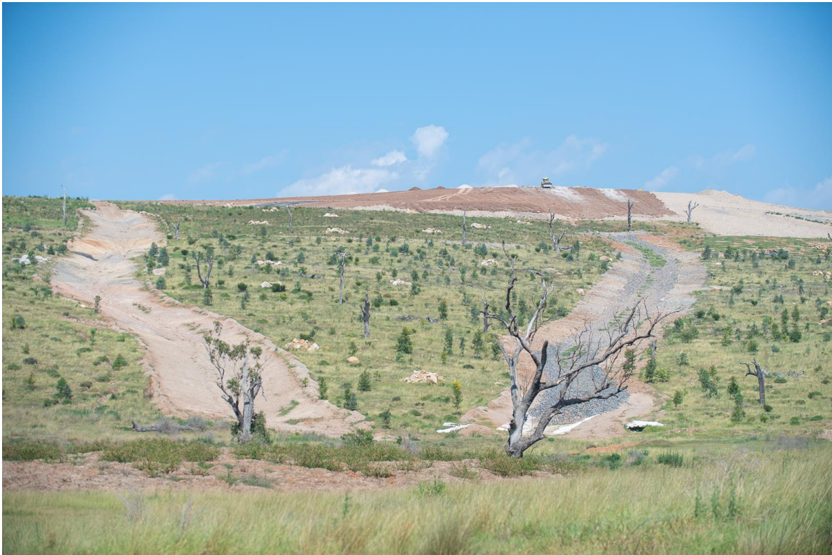
Plate 2: Eastern Out of Pit Emplacement Rehabilitation
