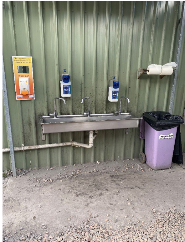
Photograph F.77 Mine infrastructure area
