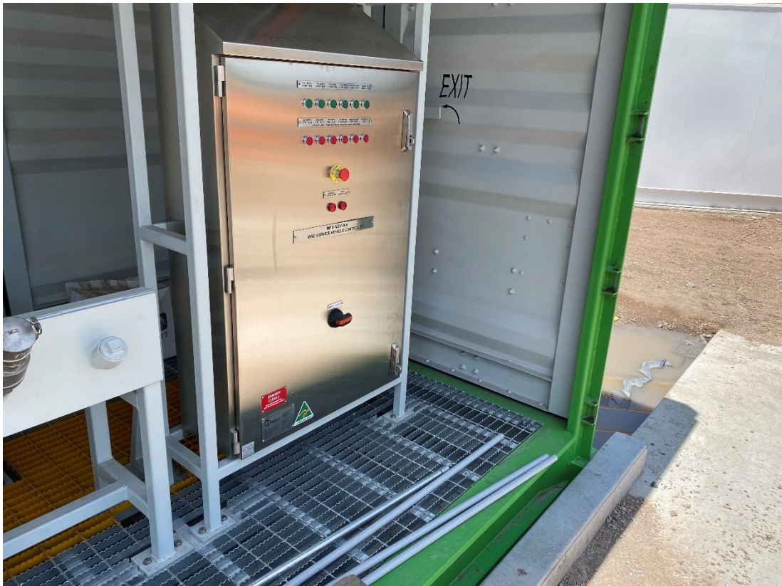
Plate 3 – New workshop lubricant / oil fill point with drainage and bunding
