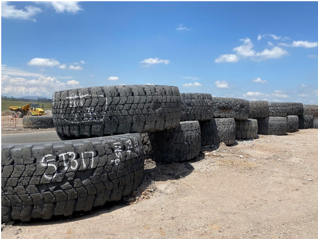
Plate 7 –Used machinery tyres used for traffic management around new workshop construction zone
