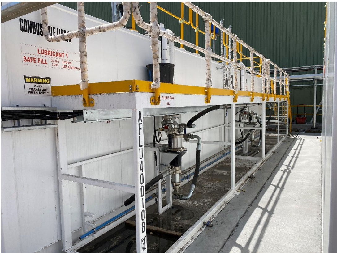
Plate 4 – New workshop lubricant storage with bunded drainage
