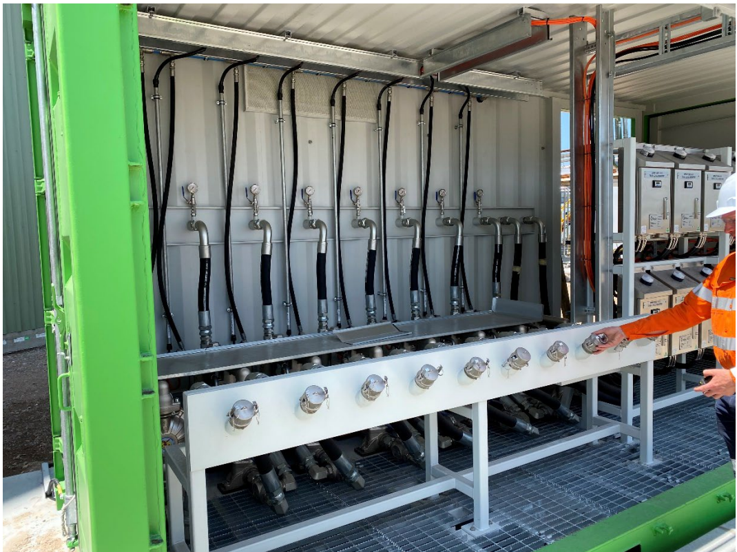
Plate 2 – New Workshop New lubricant / engine oil fill point
