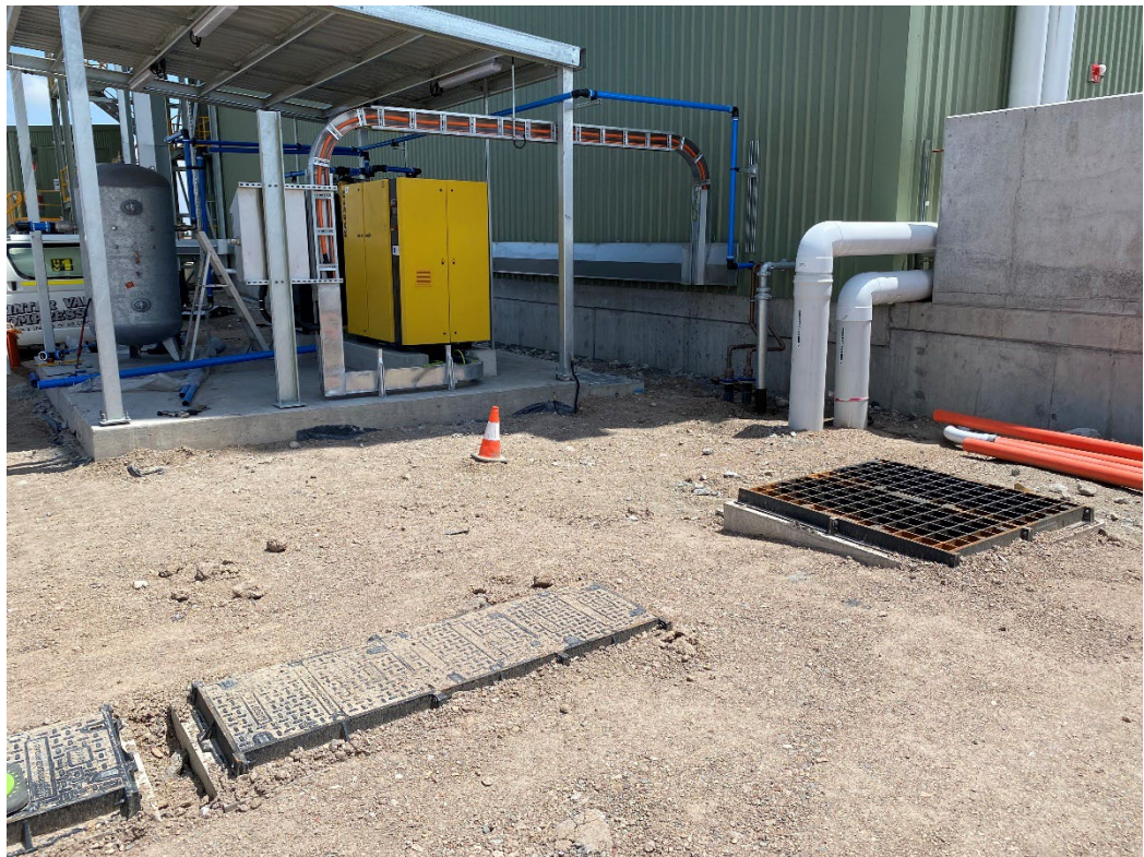
Plate 9 – New workshop stormwater pit for new workshop slab
