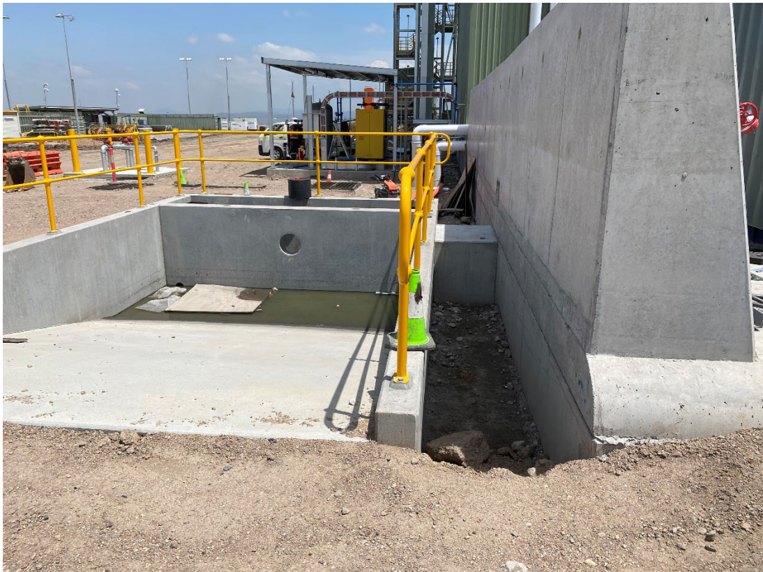
Plate 9 – New workshop stormwater pit for new workshop slab
