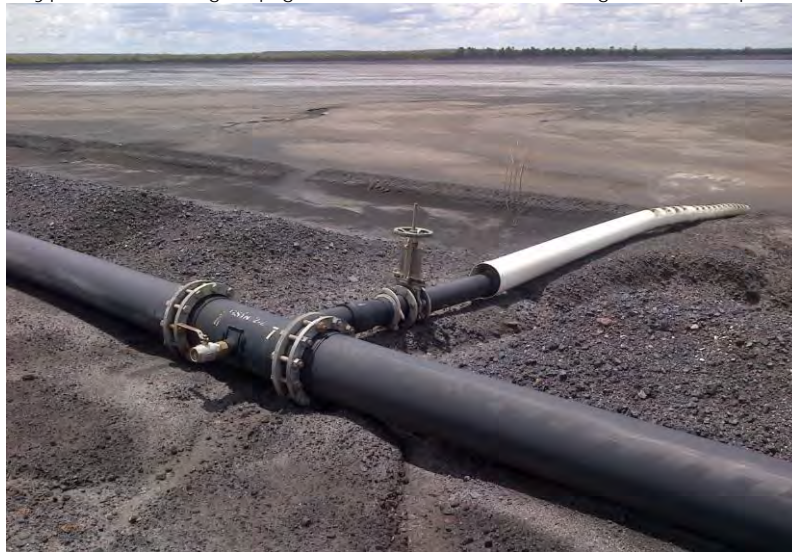
Plate 3 Typical Discharge Spigot Off-Take Line Showing Slotted Pipe
