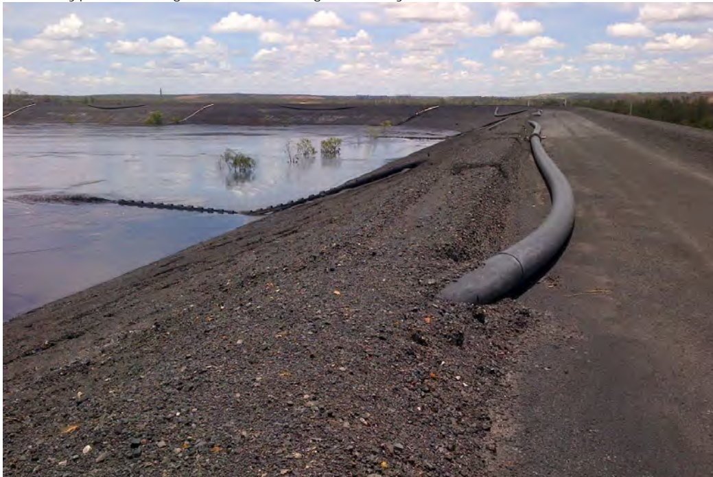
Plate 2 Typical Arrangement of Tailings Delivery Line from Embankment Crest
