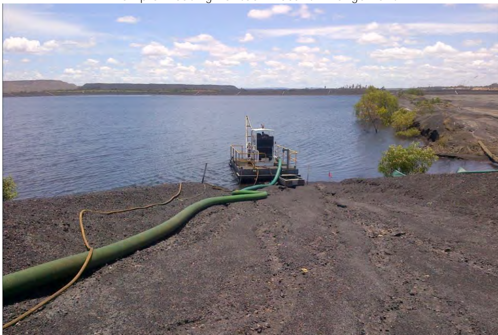
Plate 4 Example Floating Pontoon Decant Arrangement
