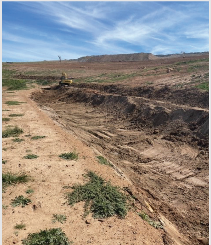
Sediment removed from a drain after a rainfall event.
